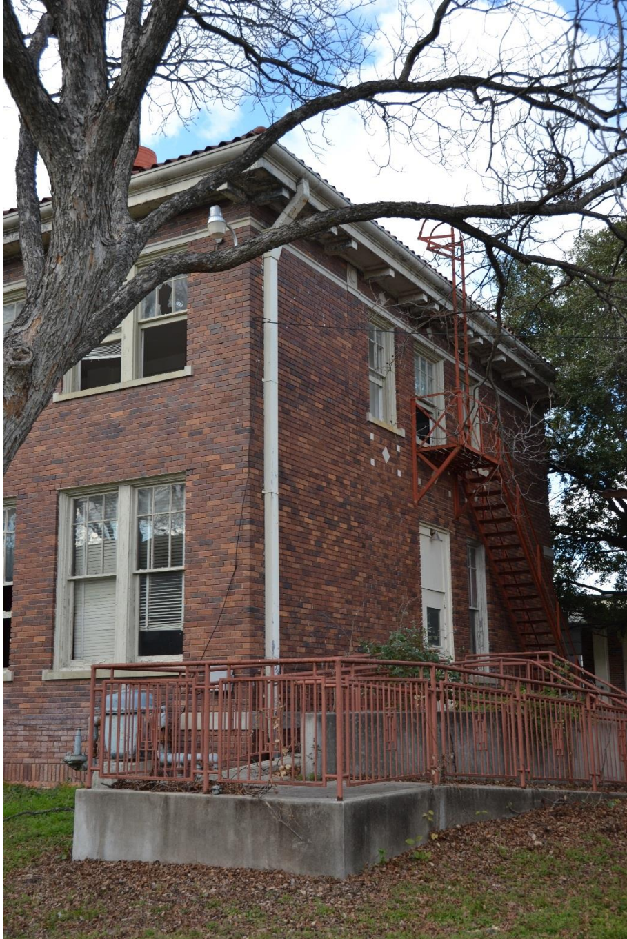
Photo 16 Margil Hall, southeast elevation Camera facing northwest
