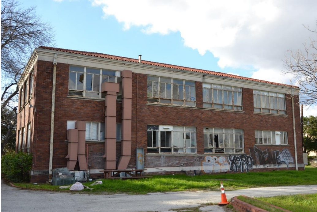
Photo 27 St. Mary's Hall, east elevation Camera facing northwest
