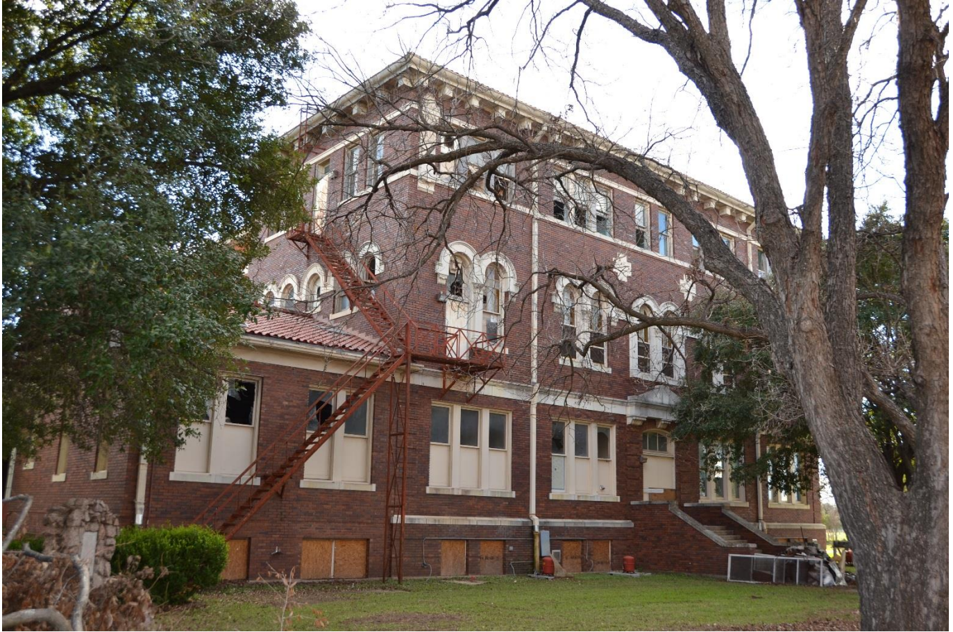
Photo 5 Main Seminary/Drossaerts Hall, north elevation Camera facing southeast
