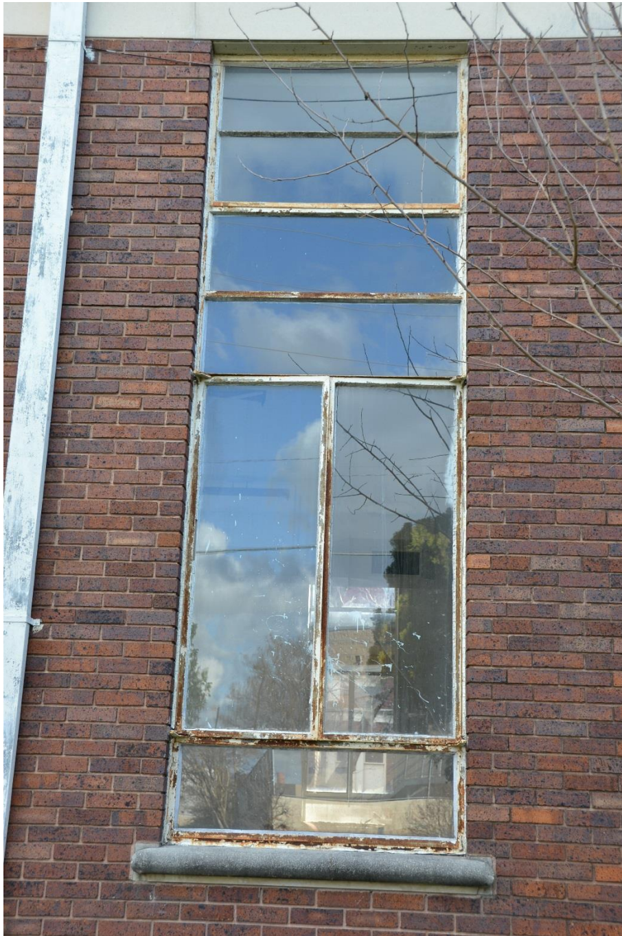
Photo 30 St. Mary's Hall, north elevation, window detail Camera facing south
