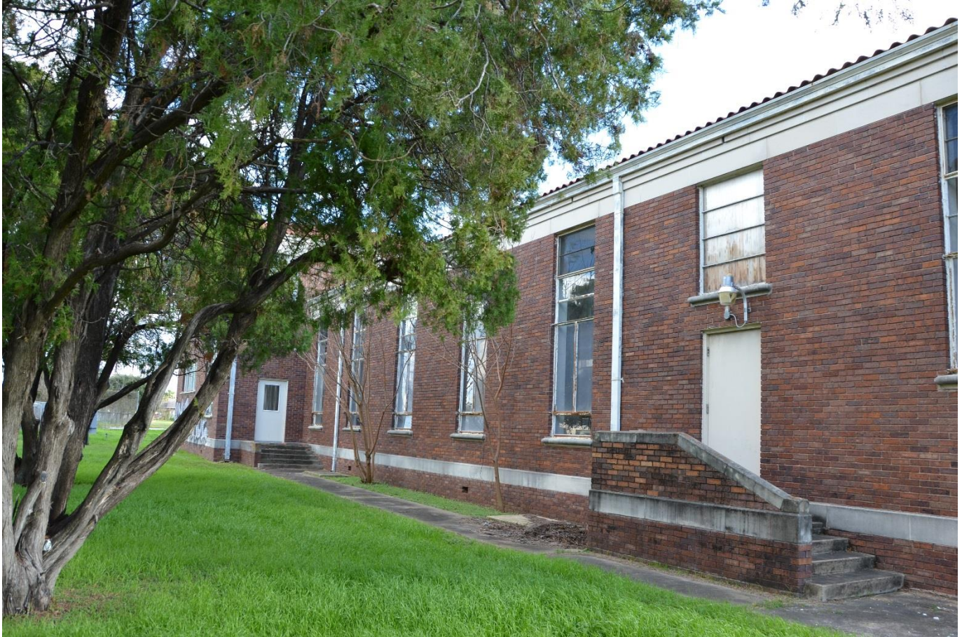
Photo 29 St. Mary's Hall, north elevation Camera facing southeast
