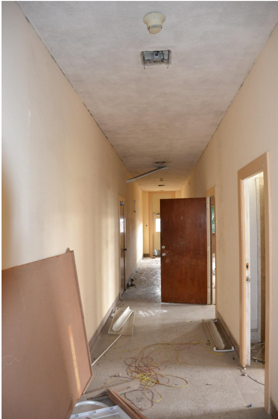
Photo 22 Margil Hall, interior first floor corridor Camera facing east
