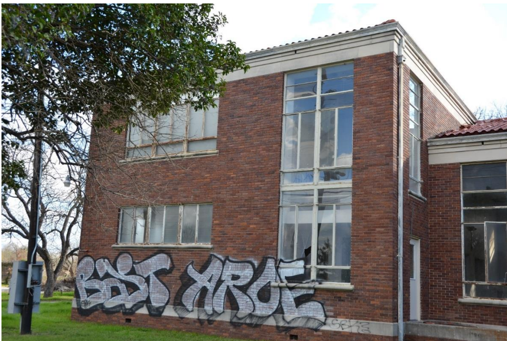
Photo 28 St. Mary's Hall, north elevation, Camera facing south
