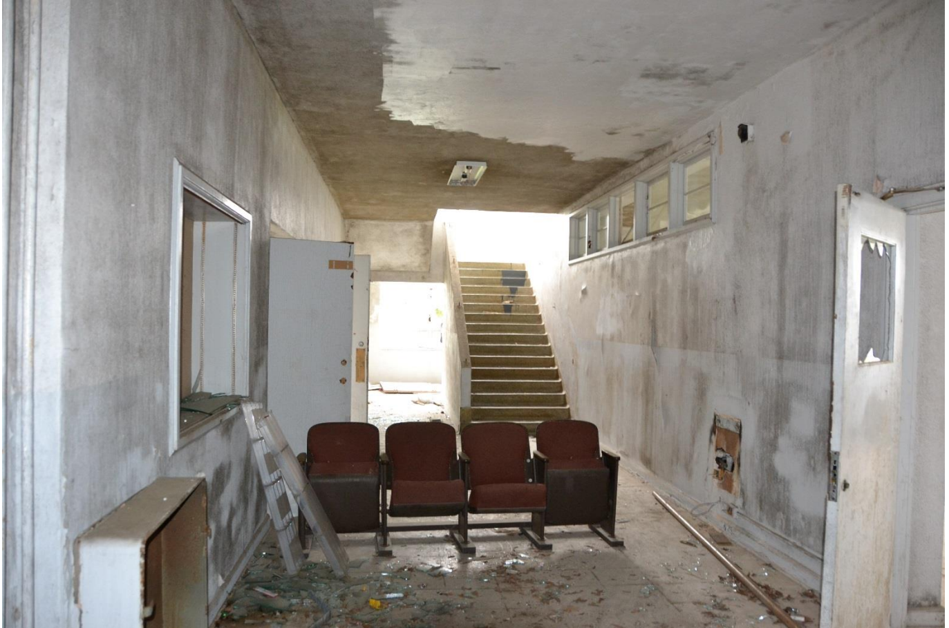
Photo 33 St. Mary's Hall, first floor Camera facing north
