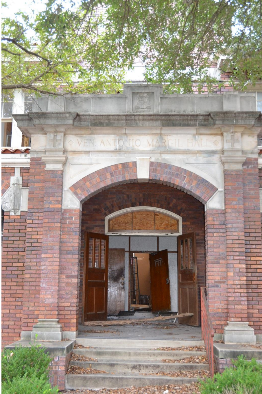
Photo 14 Margil Hall, north elevation, main entry Camera facing south
