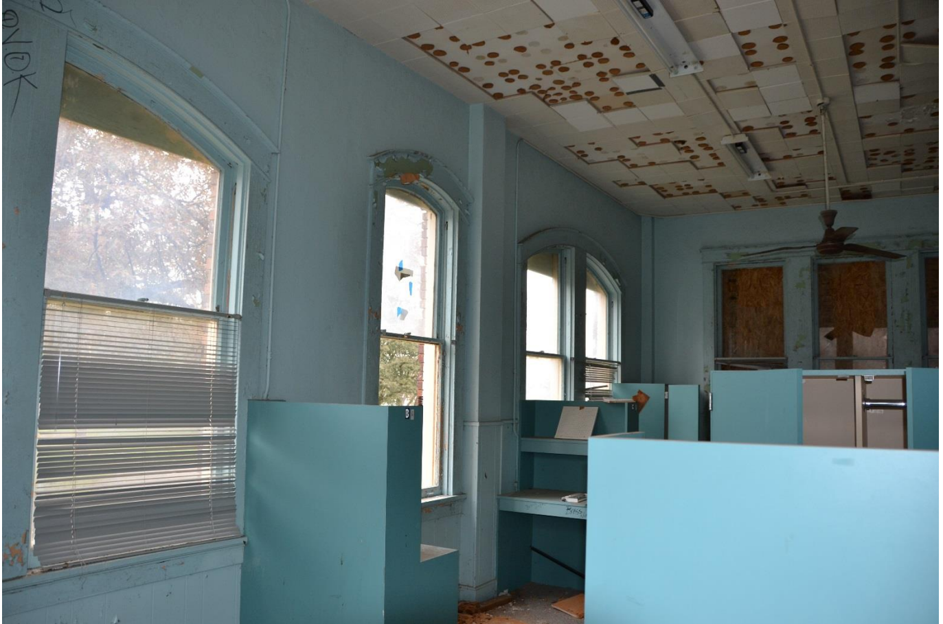
Photo 8 Main Seminary/Drossaerts Hall, interior first floor Camera facing southeast
