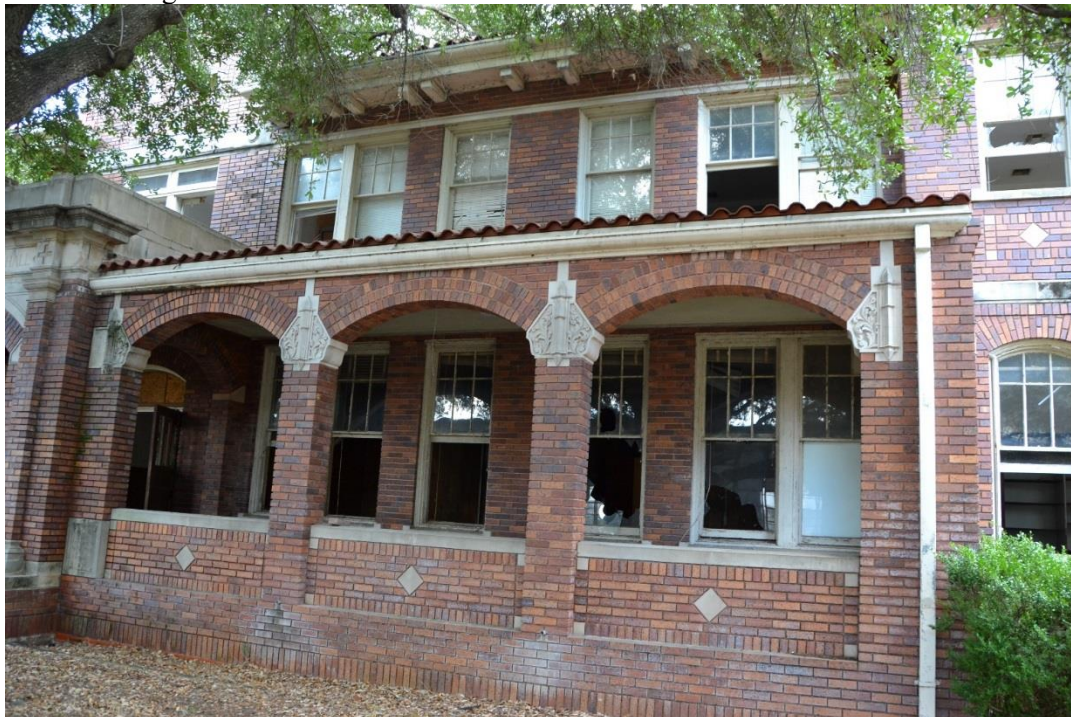
Photo 13 Margil Hall, north elevation Camera facing southeast
