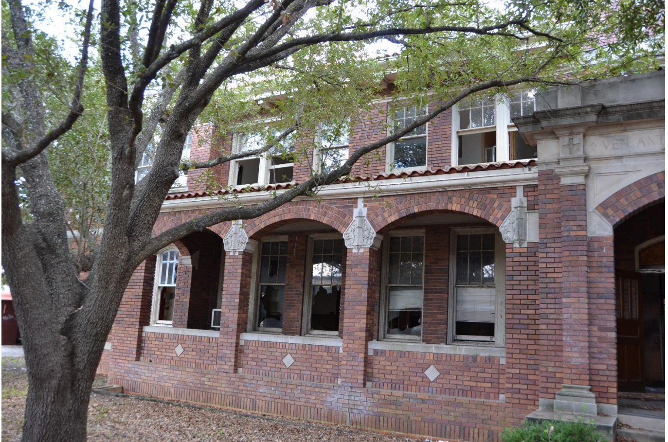
Photo 15 Margil Hall, northeast elevation Camera facing southeast
