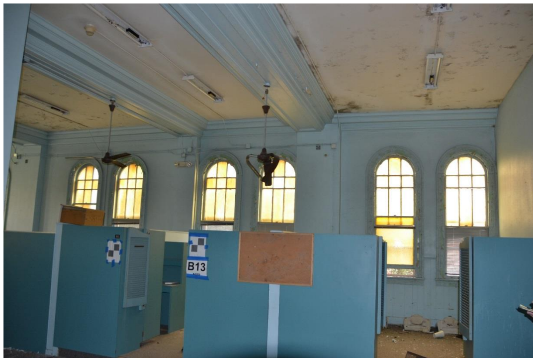
Photo 10 Main Seminary/Drossaerts Hall, interior second story Camera facing north
