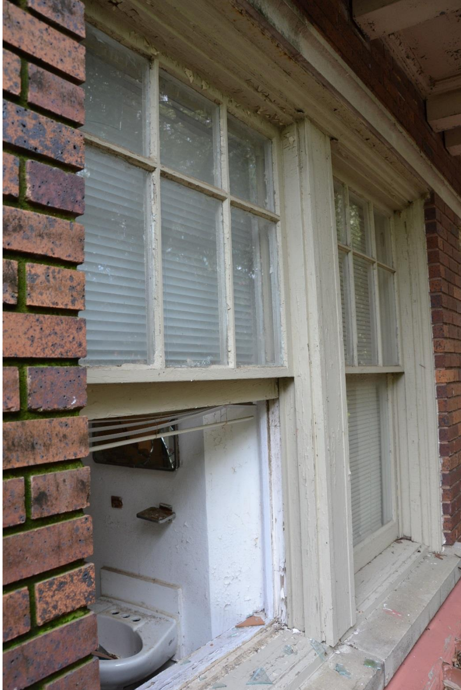
Photo 21 Margil Hall, second story window exterior detail Camera facing southeast
