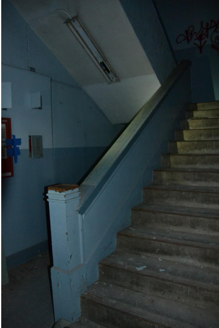
Photo 9 Main Seminary/Drossaerts Hall, interior stair Camera facing east
