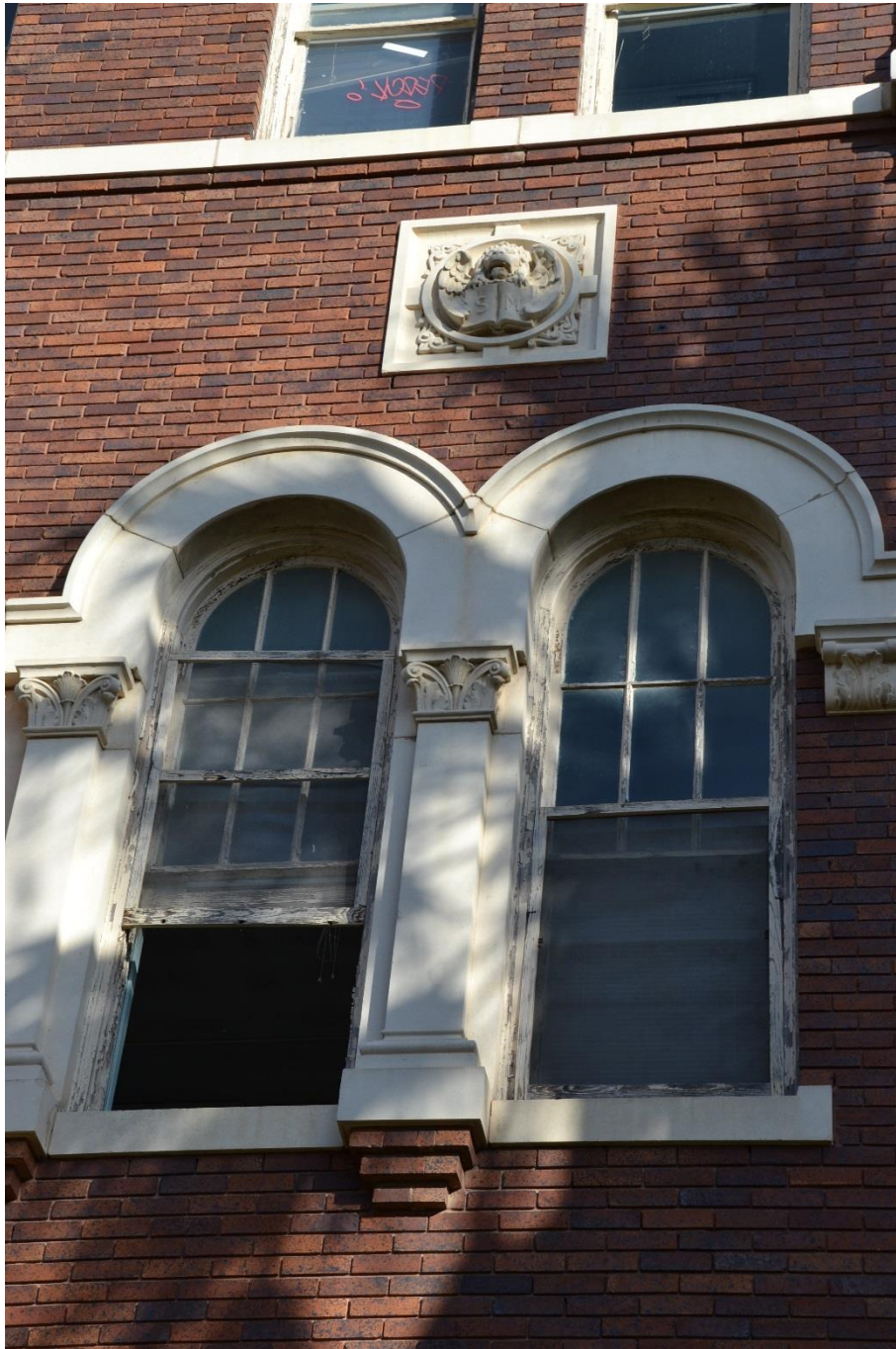
Photo 6 Main Seminary/Drossaerts Hall, window detail, west elevation Camera facing east
