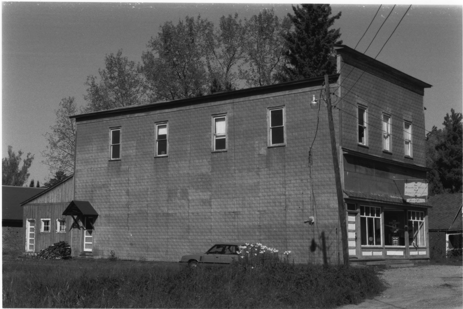
Le Moine Building St. Louis County, MN 09338/15
