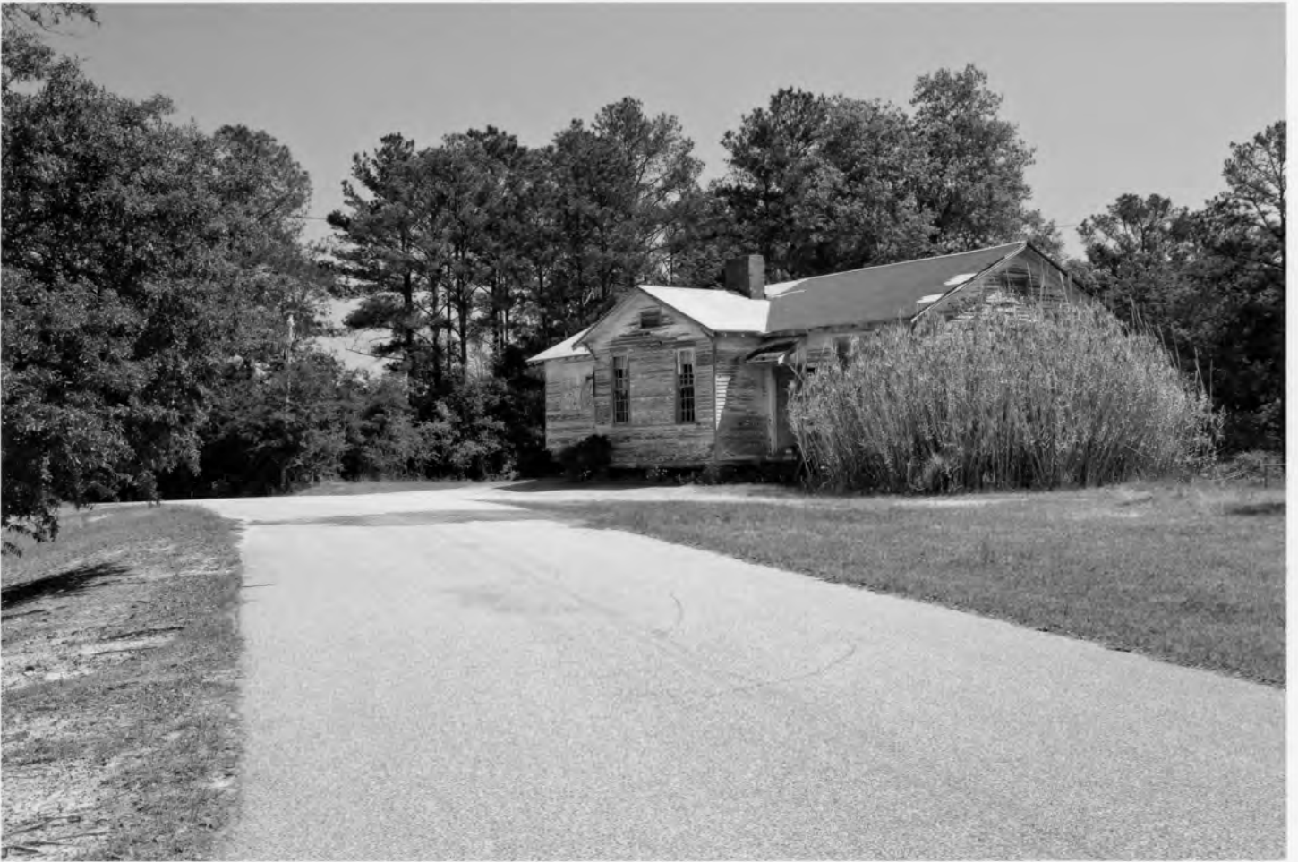
Cusseta Industrial High School Chattahoochee County, Georgia Photograph 1 of 15
