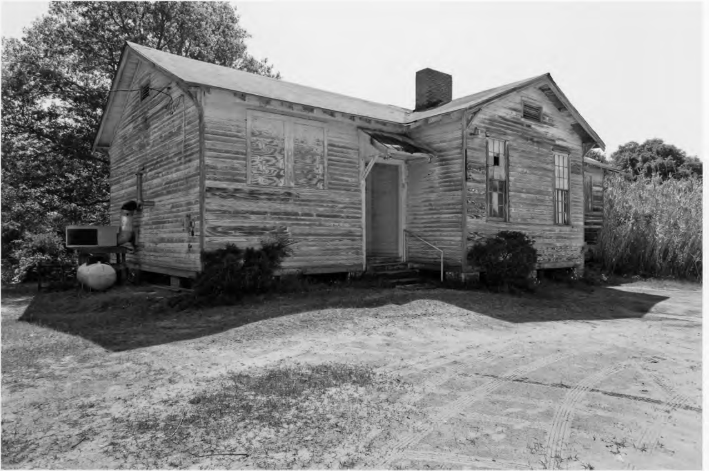
Cusseta Industrial High School Chattahoochee County, Georgia Photograph 5 of 15
