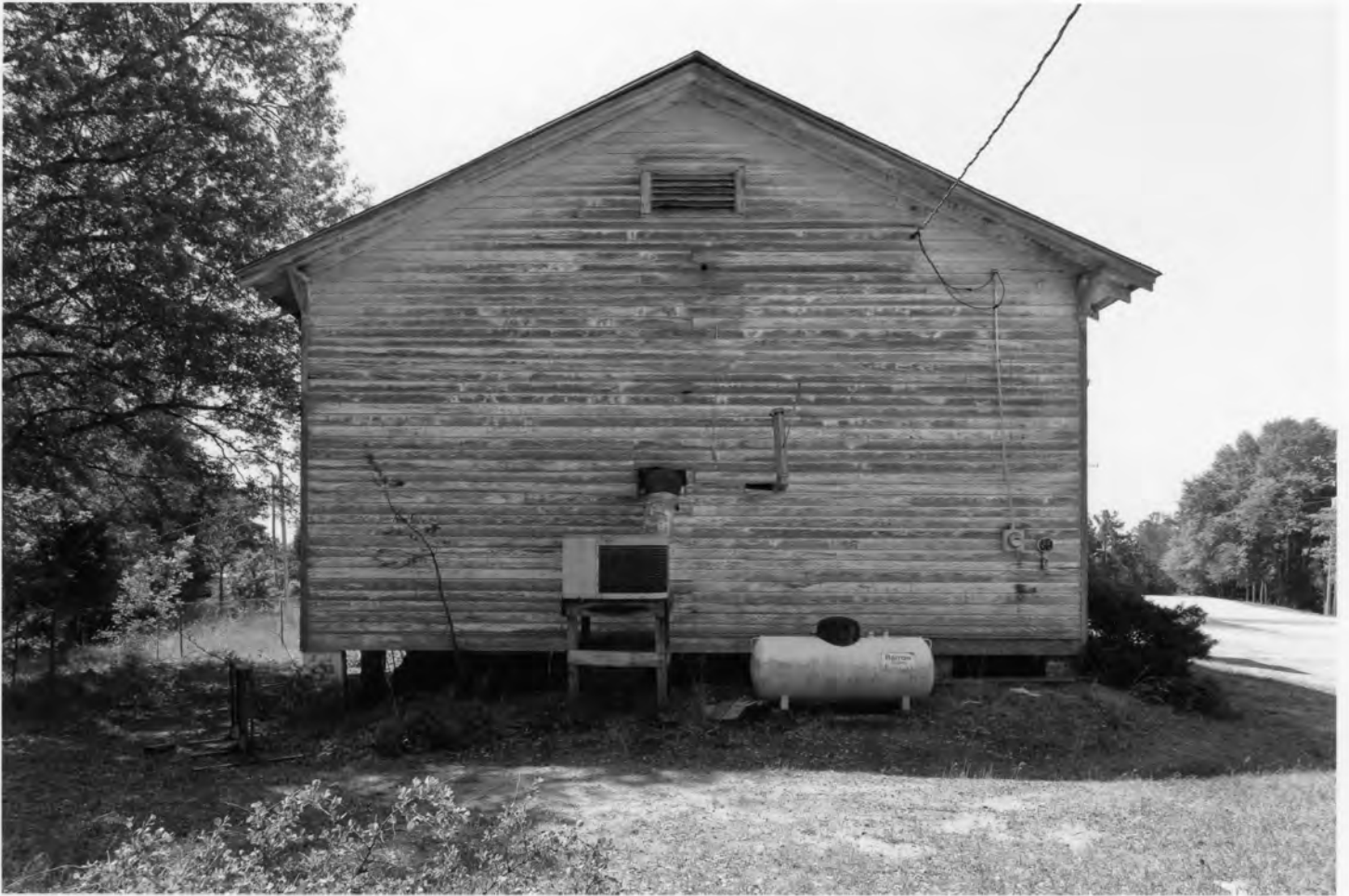
Cusseta Industrial High School Chattahoochee County, Georgia Photograph 6 of 15
