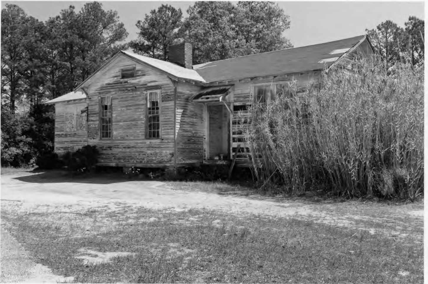
Cusseta Industrial High School Chattahoochee County, Georgia Photograph 3 of 15
