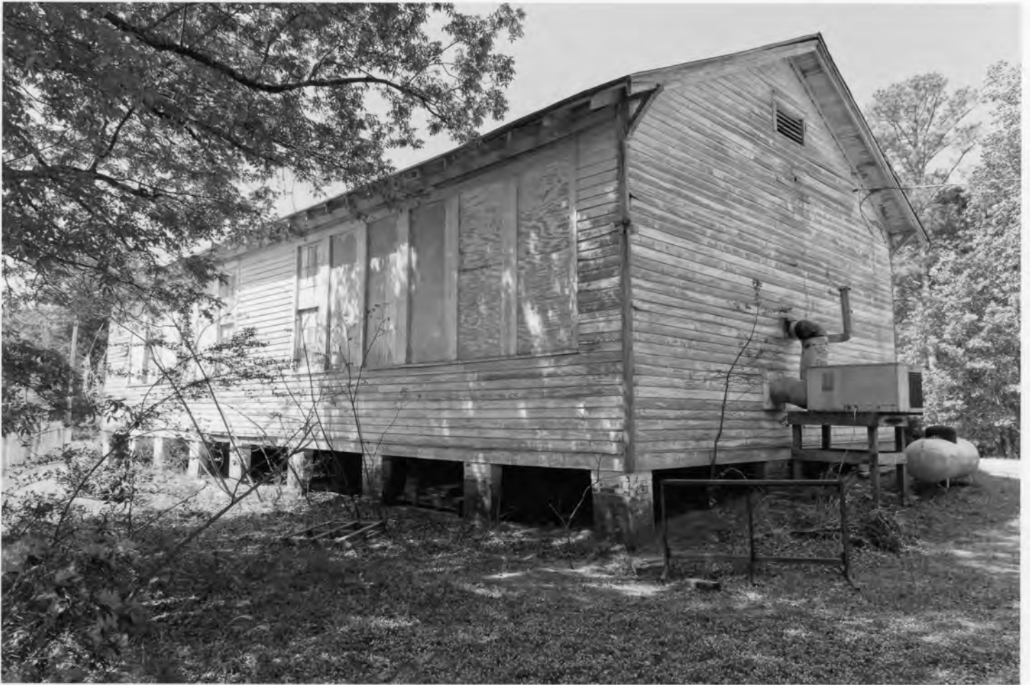
Cusseta Industrial High School Chattahoochee County, Georgia Photograph 7 of 15
