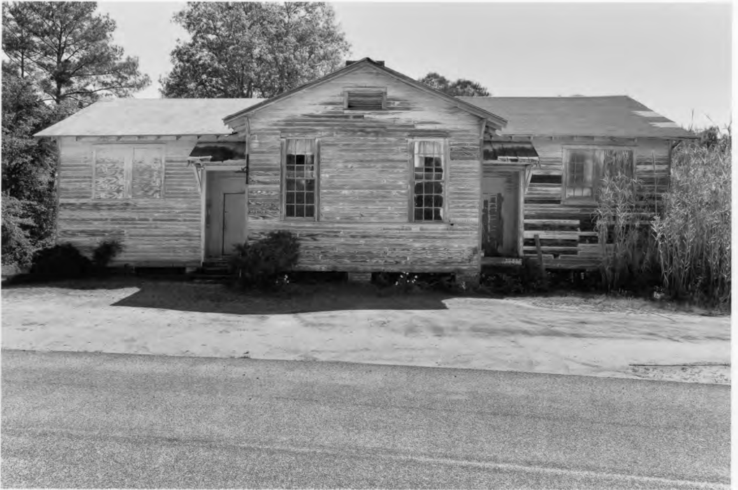
Cusseta Industrial High School Chattahoochee County, Georgia Photograph 4 of 15
