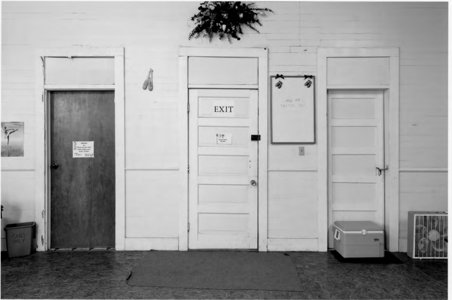
Cusseta Industrial High School Chattahoochee County, Georgia Photograph 13 of 15
