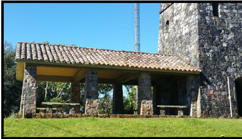
Photo 9. View of the four columns and two of the benches in the eastern picnic shelter taken from the roadway facing southwest.
