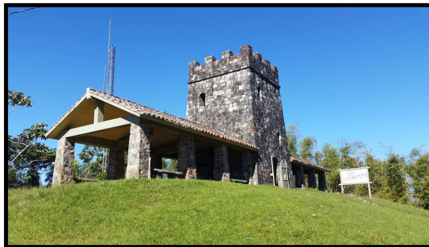
Photo 5. View of the Observation Tower facing southwest.
