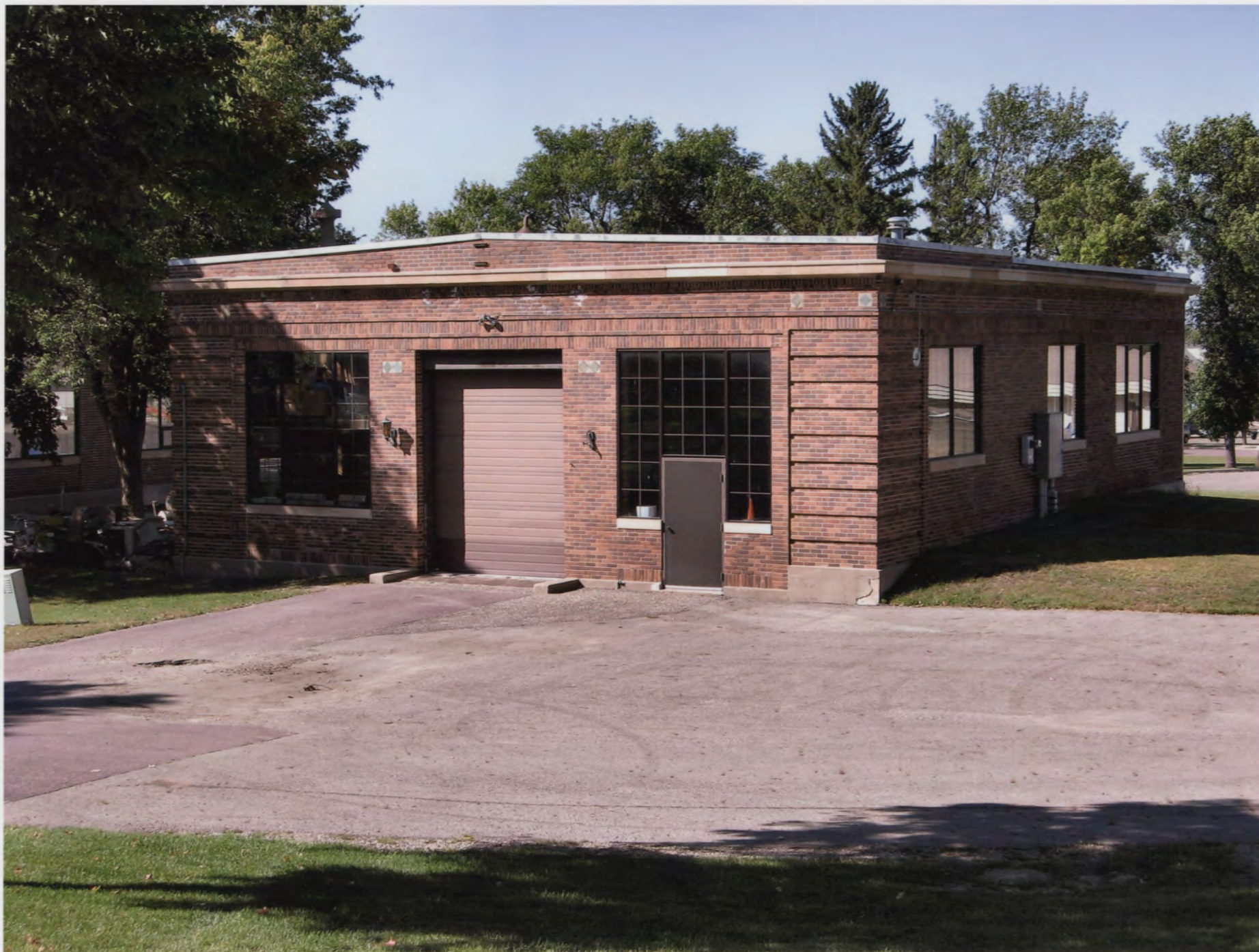
MN SteeleCounty MNStatePublicSchoolHistoricDistrict :Power Plant 0004
