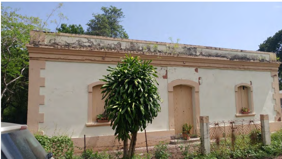
Casilla #12. Located in Coamo on PR-14, km. 27.8. Built around 1880, currently a private residence, this is one of the best preserved casillas , with its original doors and windows.
