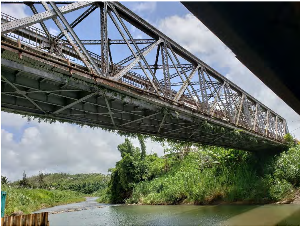
Puente Arenas, Cayey, PR-735 (old section of PR-1), km. 1.5 (b. 1894)
