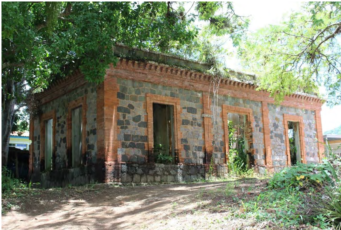
Casilla #6. Abandoned casilla de camineros in PR-14, km. 59.9, Aibonito.
