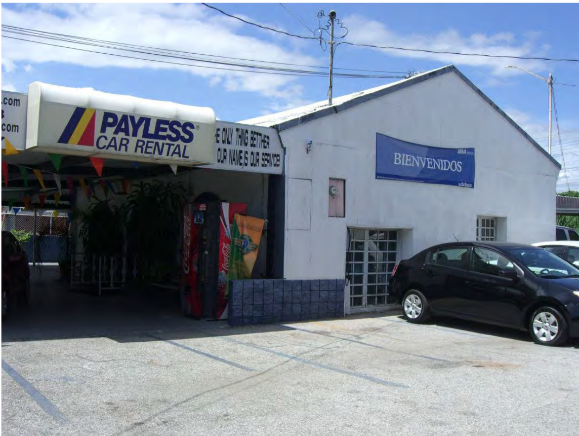
Casilla 17. Beyond recognition, this construction practically absorbed what used to be a casilla de camineros at Playa Ponce, PR-123, #1124. Some of the thick masonry walls from the casilla still visible in the building's interior.
