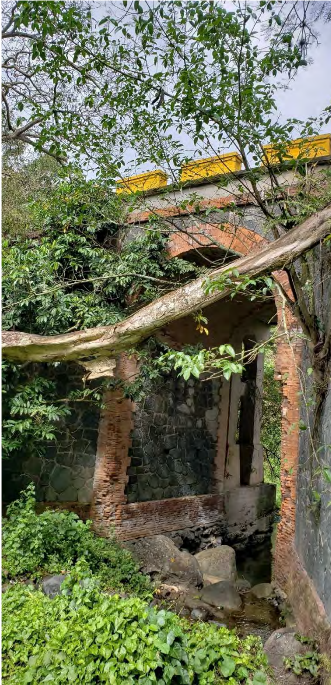
This impressive pontón , known as Puente Gómez, is in PR-14, Km. 61.9 in Aibonito. The picture on the right shows the well-designed and aesthetically early 1930s concrete columns that support the road expansion, allowing for an easier curve as the use of motor vehicles demanded a wider Carretera Central (see Section 8).
