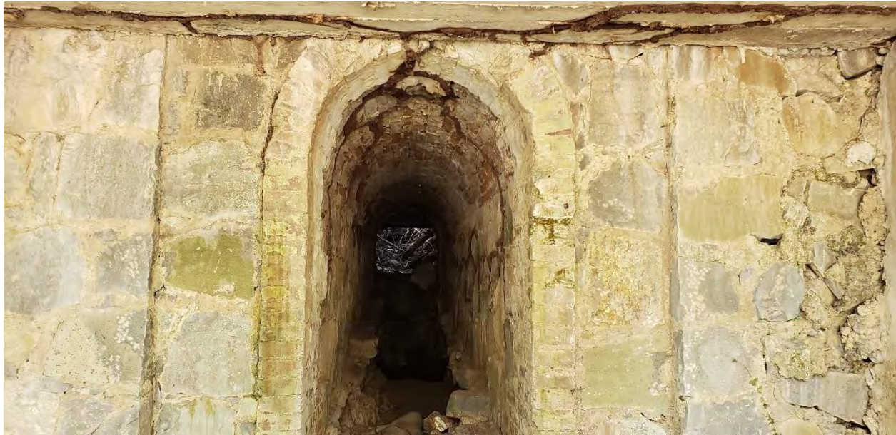
A narrow one-meter wide tajera located in PR-14, Km. 37.5, Coamo
