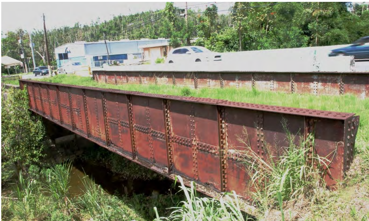
Puente Las Quebradillas, Caguas, PR-1, Km. 41.3 (b. 1881)
