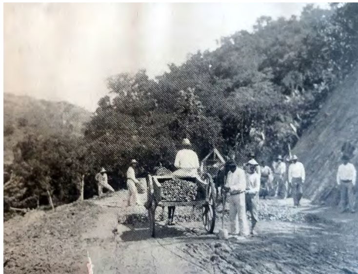
Figure 15. Laborers placing macadam.
