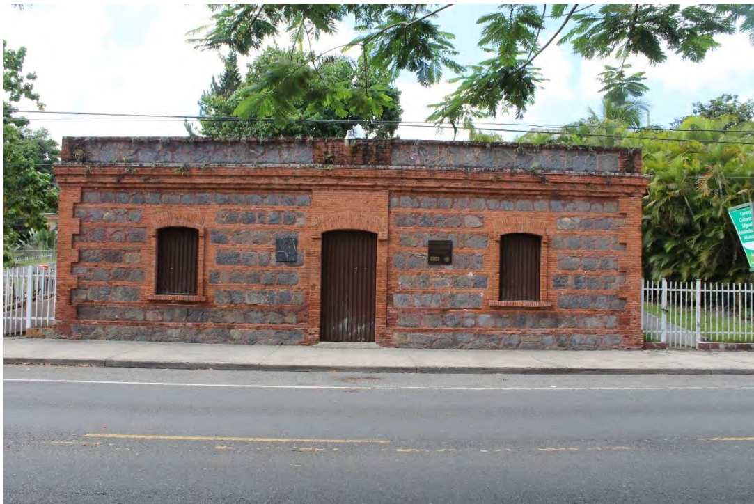
Casilla #4. Located in Cayey, PR-14, Km. 70.8. Built in 1894, is currently used as a Cultural Center.
