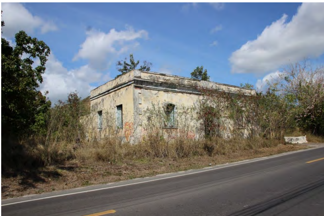
Casilla #14. Abandoned casilla, located in Juana Díaz on PR-14, km.16.4.
