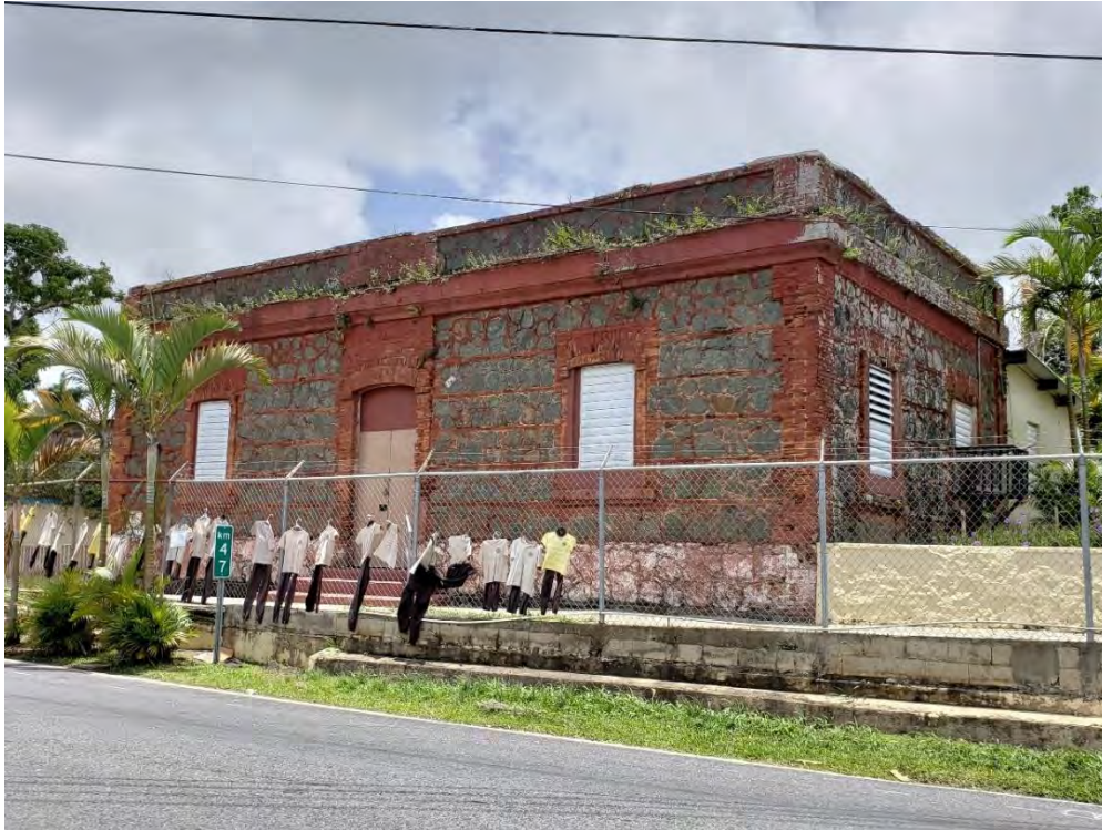
Casilla #3. Part of a school complex today ( Escuela Luis Muñoz Grillo ), the casilla is located on PR-1, KM. 47, in Caguas.
