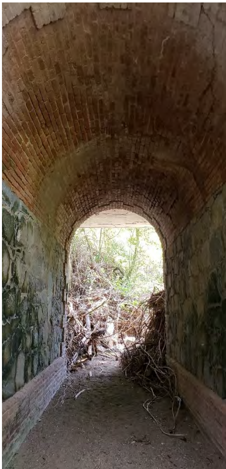
Alcantarilla in PR-14, Km. 36.6, Coamo, showing three different construction periods: the late 1920s ziggurat type columns supporting the first short expansion of the road (top picture), the six-meters long tunnel like brick and stone 19 th century tajea that supported the original travel-way and the early 1940s arched double column that supports an additional and wider expansion to the Carretera Central .
