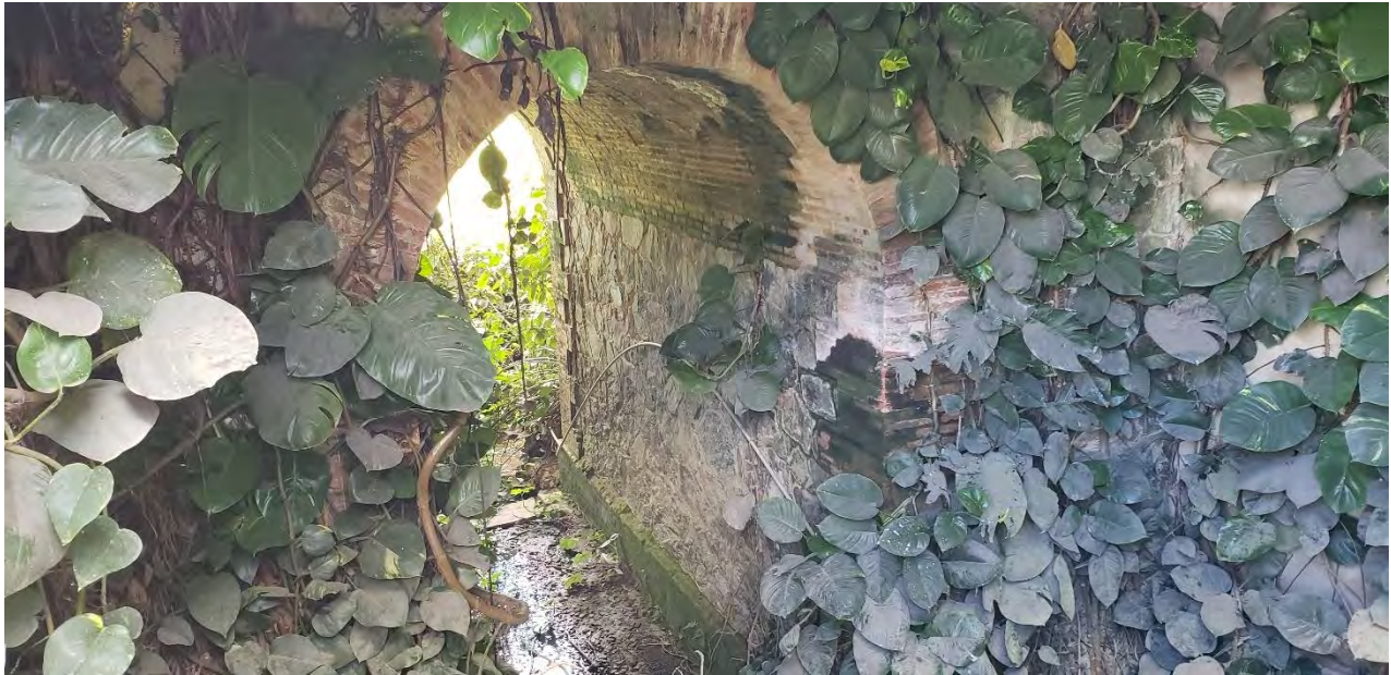
A brick and stone alcantarilla, located at PR-1, Km. 51.5, Cayey.
