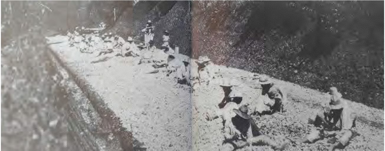
Figure 16. Laborers crushing with hammers in situ the hard stones for the first layer.
