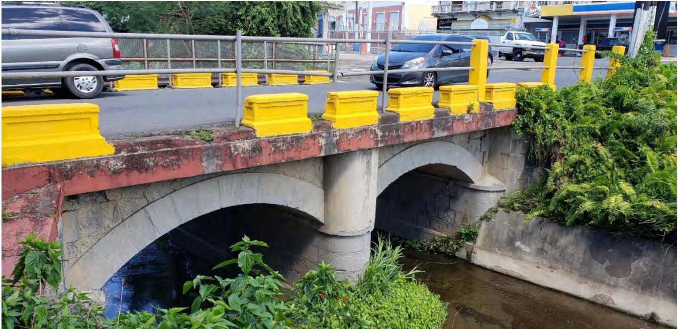
Puente Santo Domingo, Cayey, PR-14, Km. 70 (b. 1881)
