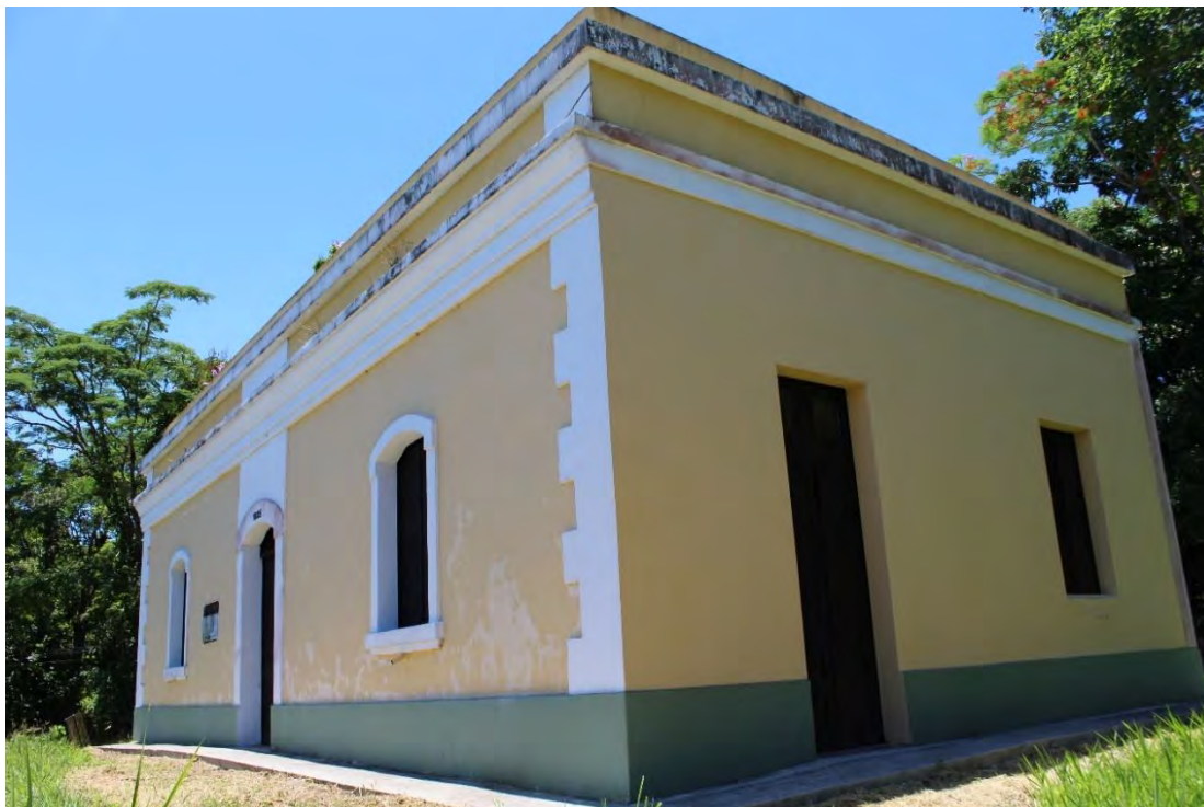
Casilla #8 . Located in Aibonito, on PR-14, km. 51.7, this 1885 casilla is used today as a Cultural Center, administered by the ICP.
