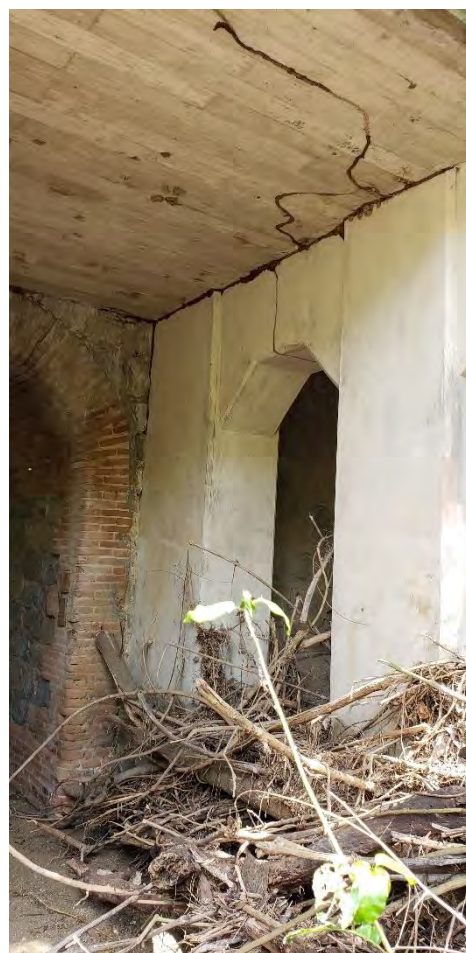
Alcantarilla in PR-14, Km. 36.6, Coamo, showing three different construction periods: the late 1920s ziggurat type columns supporting the first short expansion of the road (top picture), the six-meters long tunnel like brick and stone 19 th century tajea that supported the original travel-way and the early 1940s arched double column that supports an additional and wider expansion to the Carretera Central .
