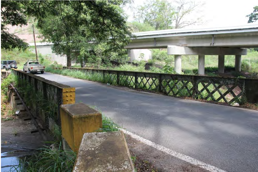
Puente Obispo Zengotita, Coamo, PR-14, km. 23.9 (b. 1879)
