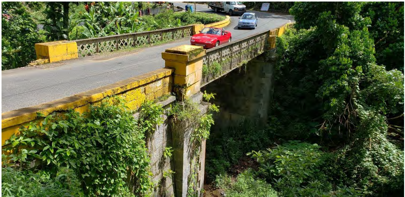
Puente Quebrada Honda, Aibonito, PR-14, km. 57.2 (1892)
