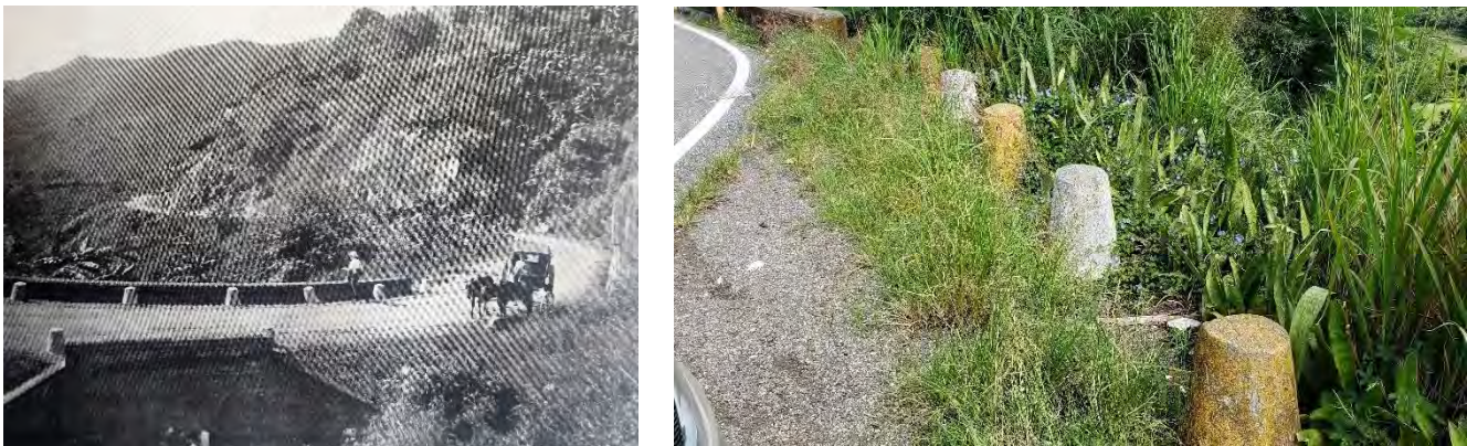
Figure 32. Left, photo of an early 20 th century section of the Carretera Central near Cayey showing the safety barriers. On the right, similar safety posts along the tract Cayey – Aibonito, PR-14, km 60. 106
