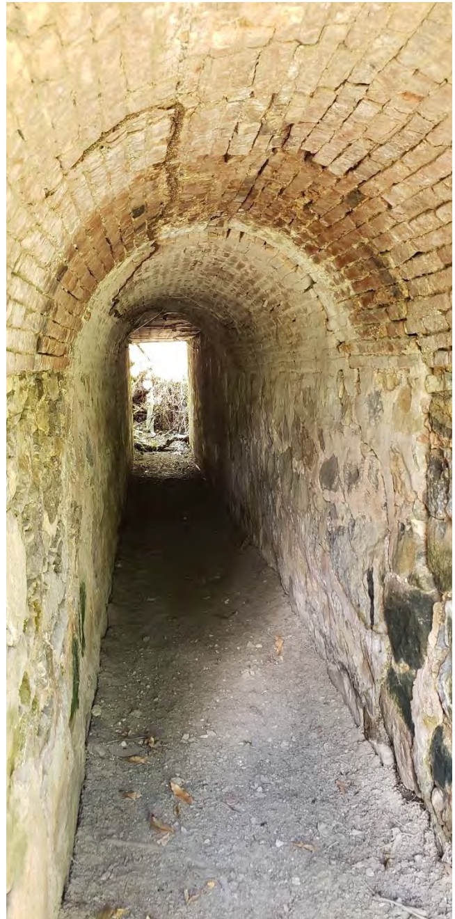
A wonderful brick and stone alcantarilla that expands the entire width of the road above, allowing water to run through it without causing any damages to the road. The tunnel like structure is located at PR-14, km. 18.0 in Juana Díaz.
