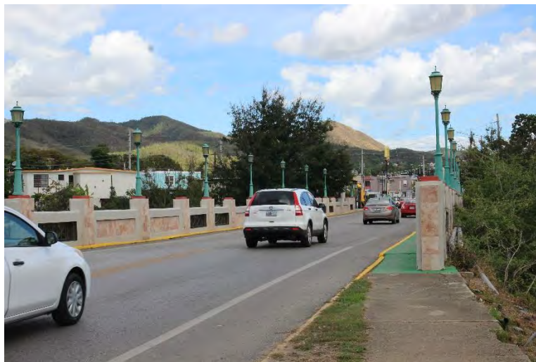
Figure 7. Three modern 1980-90s bridges in the Carretera Central. The first two are in PR-14, Ponce's jurisdiction. The last one is in PR-14, at Juana Díaz's urban center western entrance. In total, there are 24 bridges in the Carretera Central , out of which, eight are not contributing resources for the purpose of this nomination.
