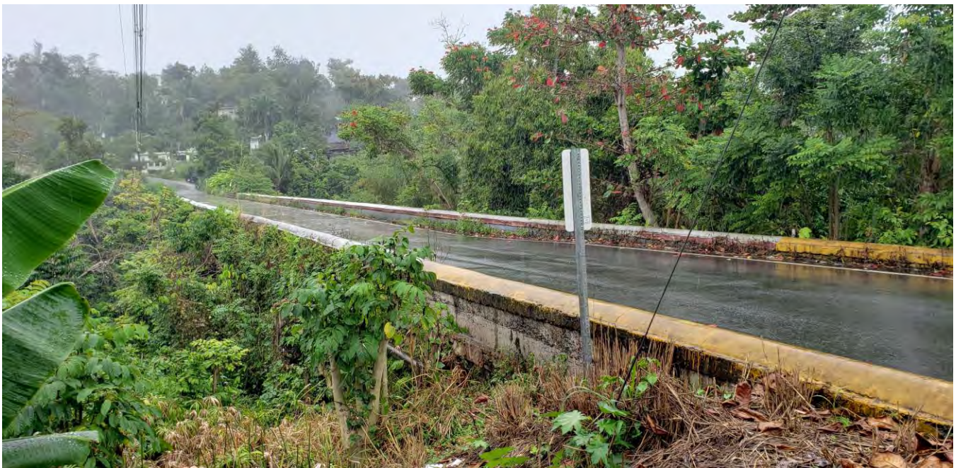
Puente de Norzagaray, San Juan, PR-873, Km. 0.8 (b. 1855)
