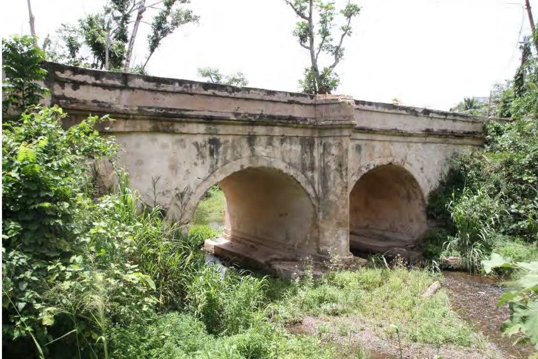
Pontón La Concepción, Caguas, PR-798, km. 1.0 (b. 1856)
