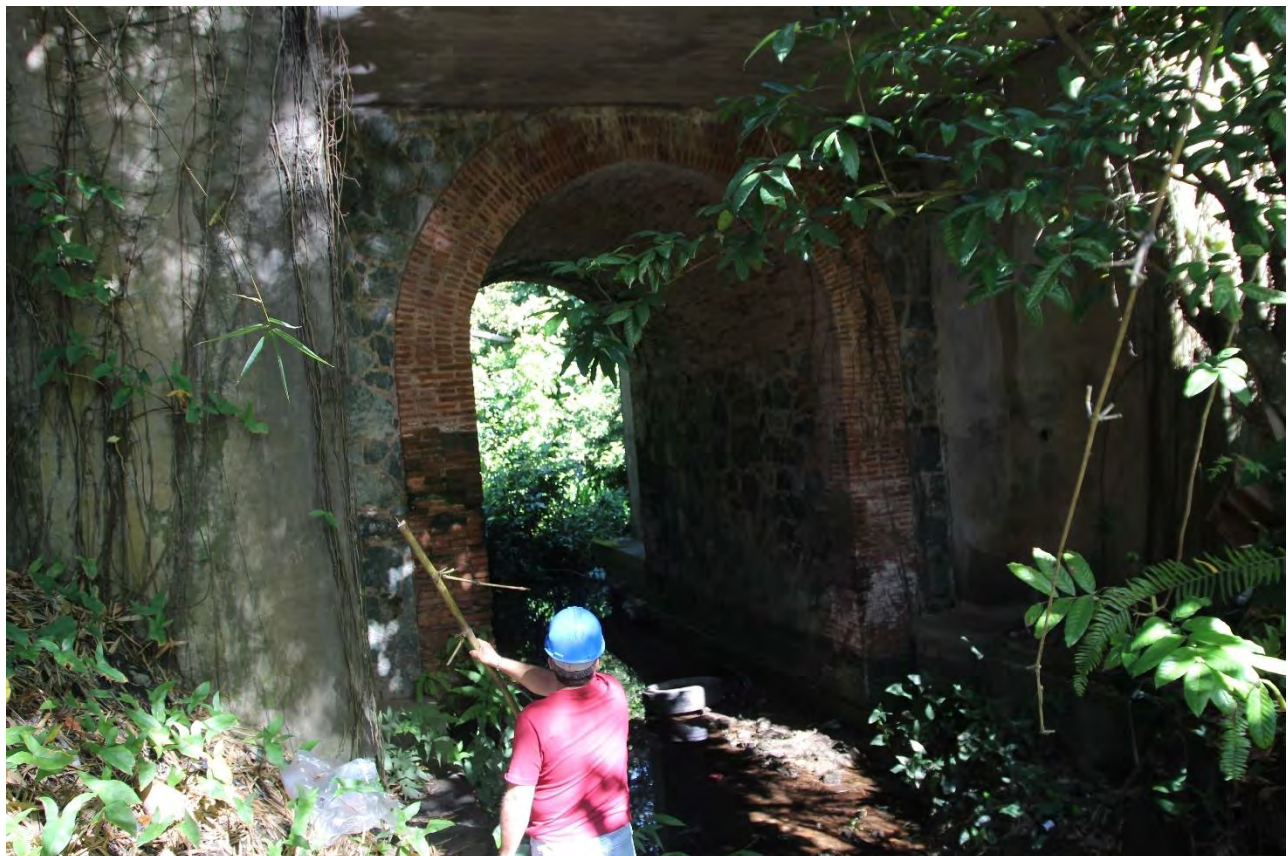
Alcantarilla, PR-1, 50.8, Cayey.
