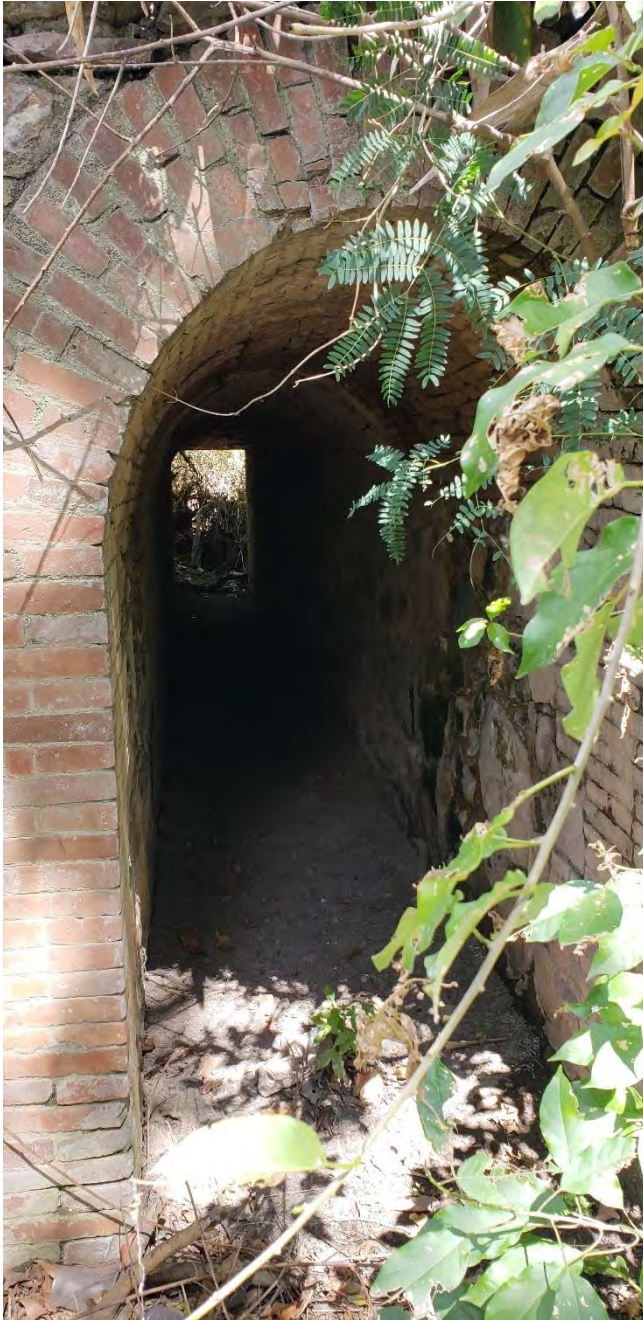
A wonderful brick and stone alcantarilla that expands the entire width of the road above, allowing water to run through it without causing any damages to the road. The tunnel like structure is located at PR-14, km. 18.0 in Juana Díaz.
