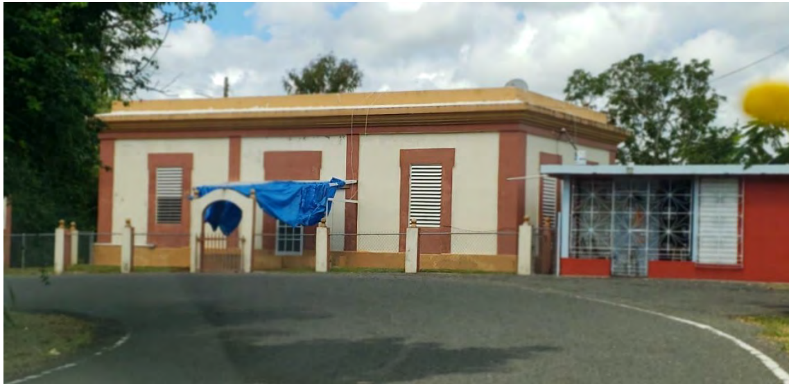
Casilla #7 . This casilla, a private dwelling today, is located in PR-14, km. 57.7, in the municipality of Aibonito. 10
