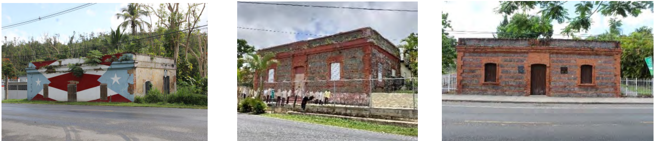
Figure 26. Three of the casillas de camineros built along the section Caguas-Cayey. The first two (from left to right) are located at PR-1, km. 40.9 and km. 47, respectively. The third one is located at PR-14, km.70.8
