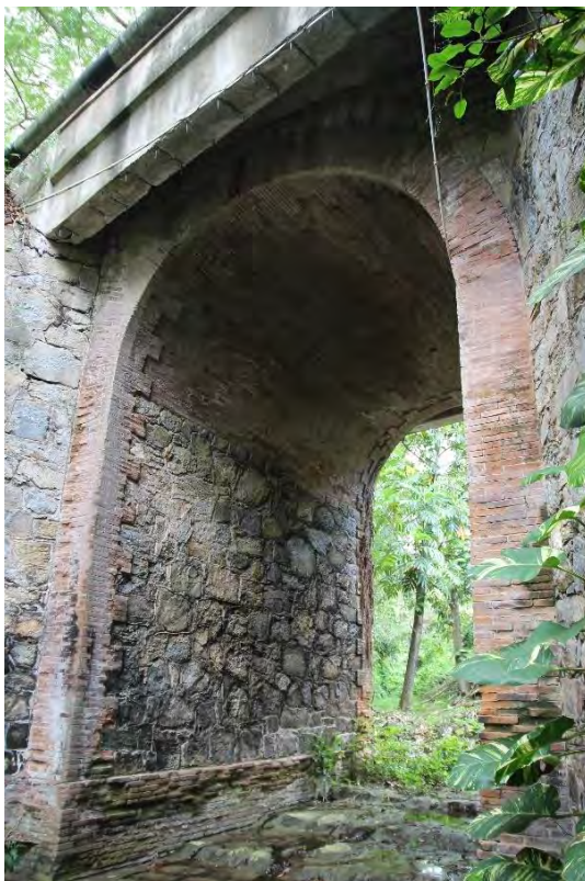
The top portion of this impressive pontón , in PR-14, Km. 40.3 in Coamo, was partially destroyed by the Spanish troops during the Spanish American War to delay the US Army advance using the Carretera Central on their way to San Juan (See, Section 8).
