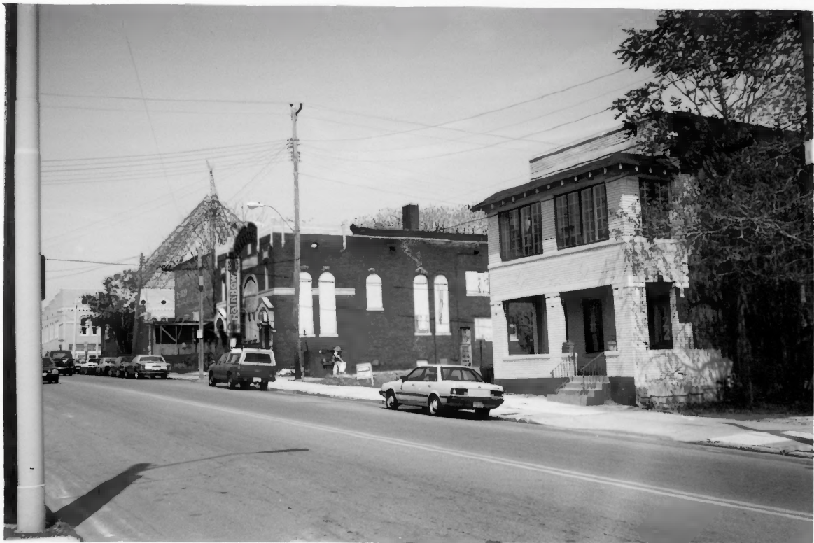
Pinch- North Main Commercial District Shelby Co TN
