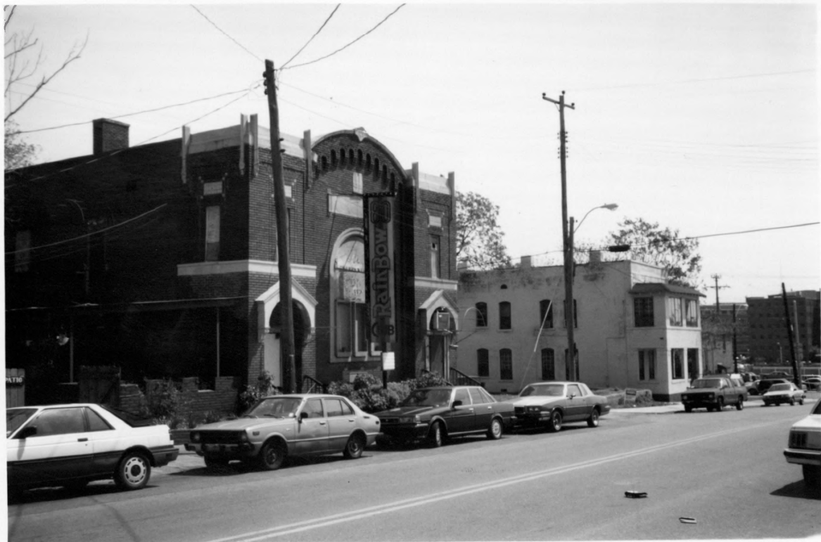
Pinch-North Main Commercial District Shelby Co TN
