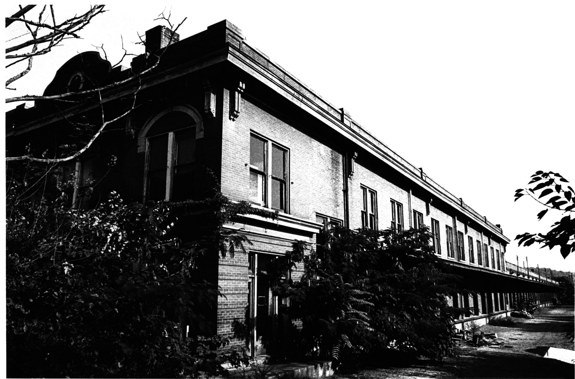
L. & N. Freight Depot Front-West Elevation August 1980
