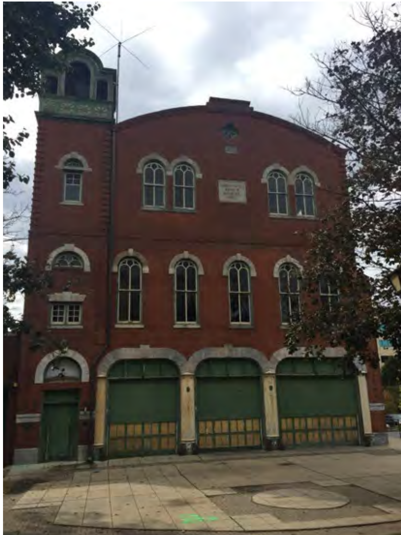
Figure 17: Washington Hose and Steam Fire Engine Company, No. 1 (PA SHPO Key No. 000581) – 15 West Hector Street, Conhohocken, Montgomery County, Pennsylvania. The firehouse was constructed in 1878, is Italianate in style, three bays wide, three stories in height, and features a prominent square hose tower with a wooden belfry. Although larger than the Humane Fire Engine Company No. 1, this is one of the most comparable National Register-listed firehouses in Pennsylvania (Photograph by Maureen McDougall 10/20/2018).
