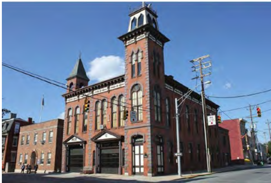
Figure 19: Laurel-Rex Fire Company House (PA SHPO Key No. 001055) – 41 South Duke Street, York, York County, Pennsylvania. The Laurel-Rex Fire Company House, constructed in 1878, is an example of an Italianate red brick firehouse with hose tower. The firehouse is more elaborately detailed than the Humane Fire Engine Company No. 1. The firehouse has two bell towers: a faux bell tower is located at its northwest corner, and a mansard-roofed belfry rises above the prominent hose tower located at its southwest corner (photograph by Steve Tinker, dated 12-18-2017, courtesy of https://www.theclio.com/web/entry?id=53136 ).
