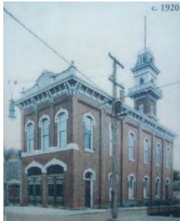
PHOTOGRAPH OF THE PHILLIES FIRE COMPANY CIRCA 1920, FACING SOUTH-SOUTHEAST (PHOTOGRAPH COURTESY OF THE PHILLIES FIRE COMPANY)
