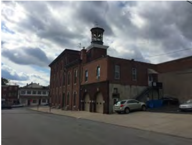
VIEW OF THE FAIRMOUNT FIRE COMPANY NO. 2, FACING SOUTHWEST (PHOTOGRAPH BY MAUREEN MCDUGALL, 10/20/2018)
