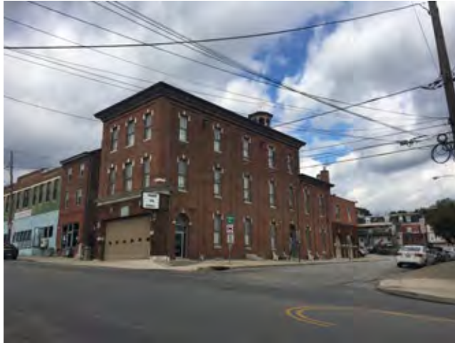
VIEW OF THE FAIRMOUNT FIRE COMPANY NO. 2, FACING NORTH-NORTHWEST (PHOTOGRAPH BY MAUREEN MCDUGALL, 10/20/2018)
