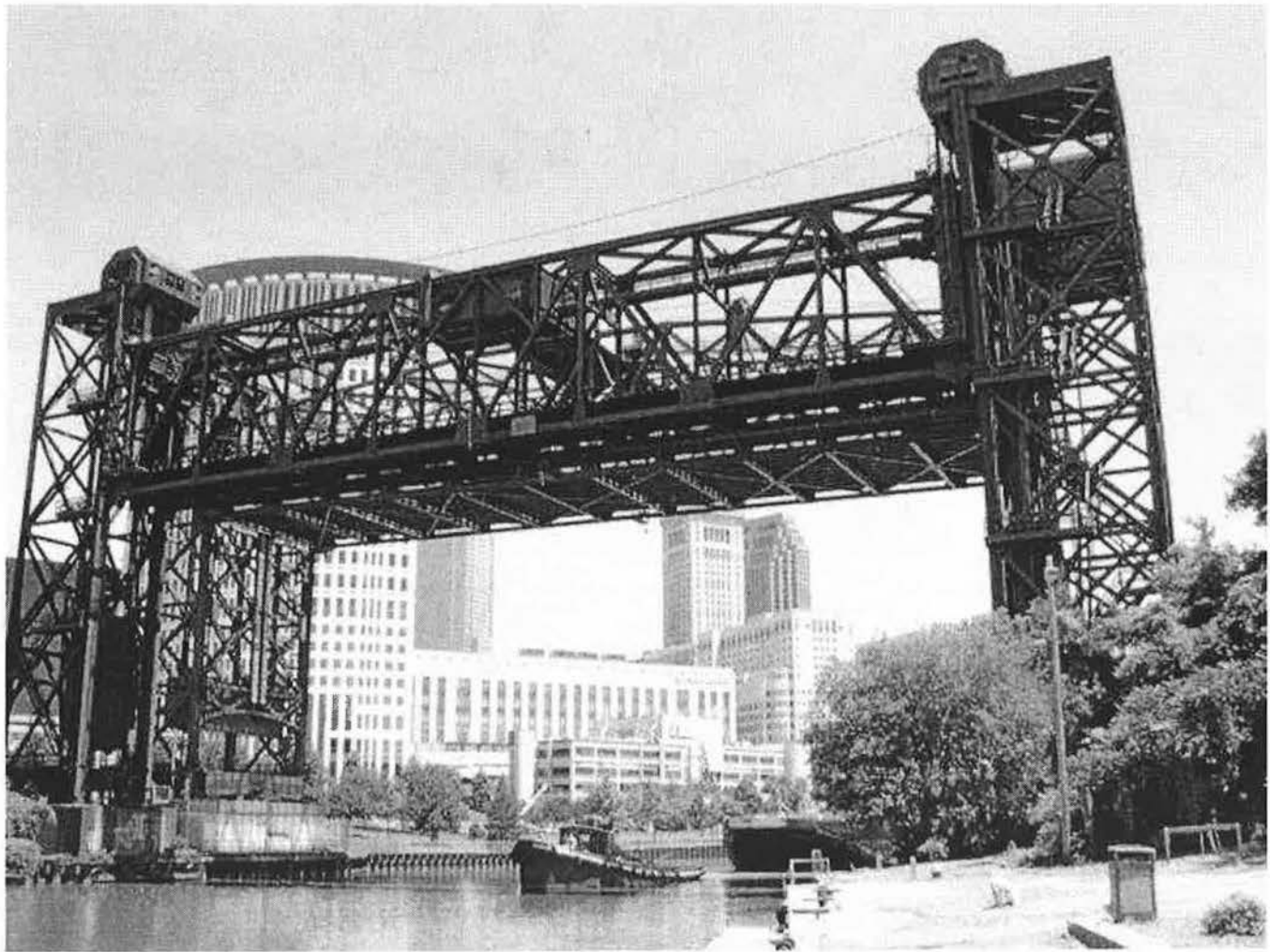
Figure 25. New York Central Main Line Bridge (adjacent to Carter Road Lift Bridge). (source: Nathan Holth photographer)
