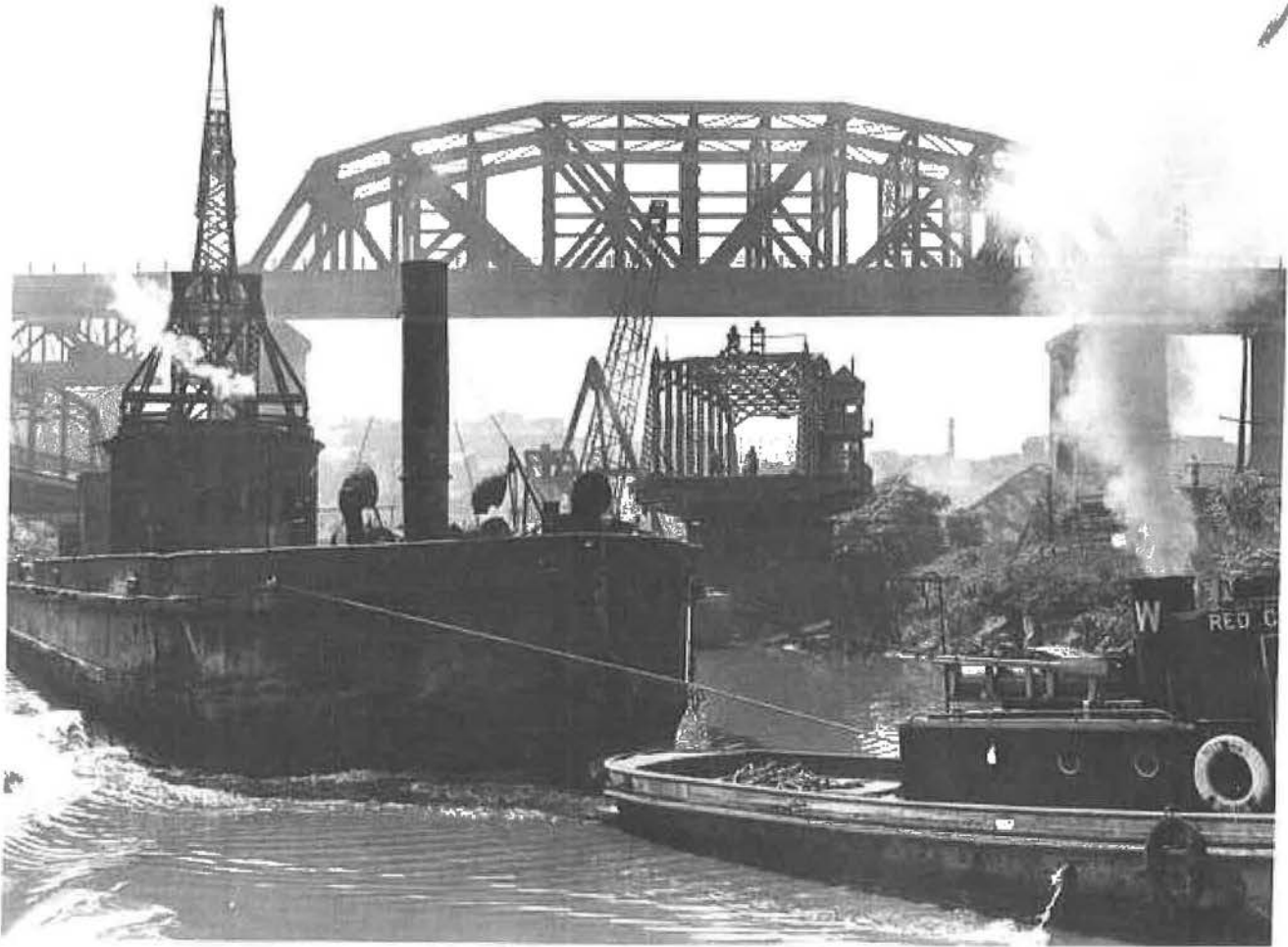
Figure 11. 20 th century photo of the 1895 twin swingspan Columbus Road Bridge before its replacement by a lift bridge in 1940. (source: www.clevelandmemory.org )
