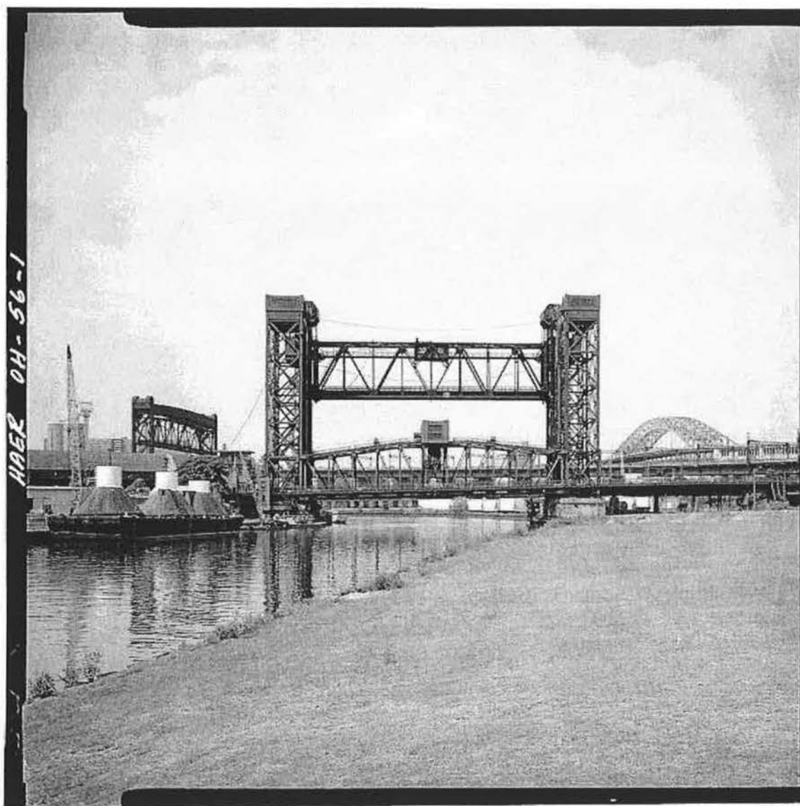
Figure 22. Carter Road Bridge in lowered position. Behind it is the New York Central RR Bridge in the raised position. In the background are the New York Central spur (now Flats Industrial RR Bridge) at left and the river span of the Detroit-Superior High Level Bridge at right. (source: HAER photo by Randal Gooden)
