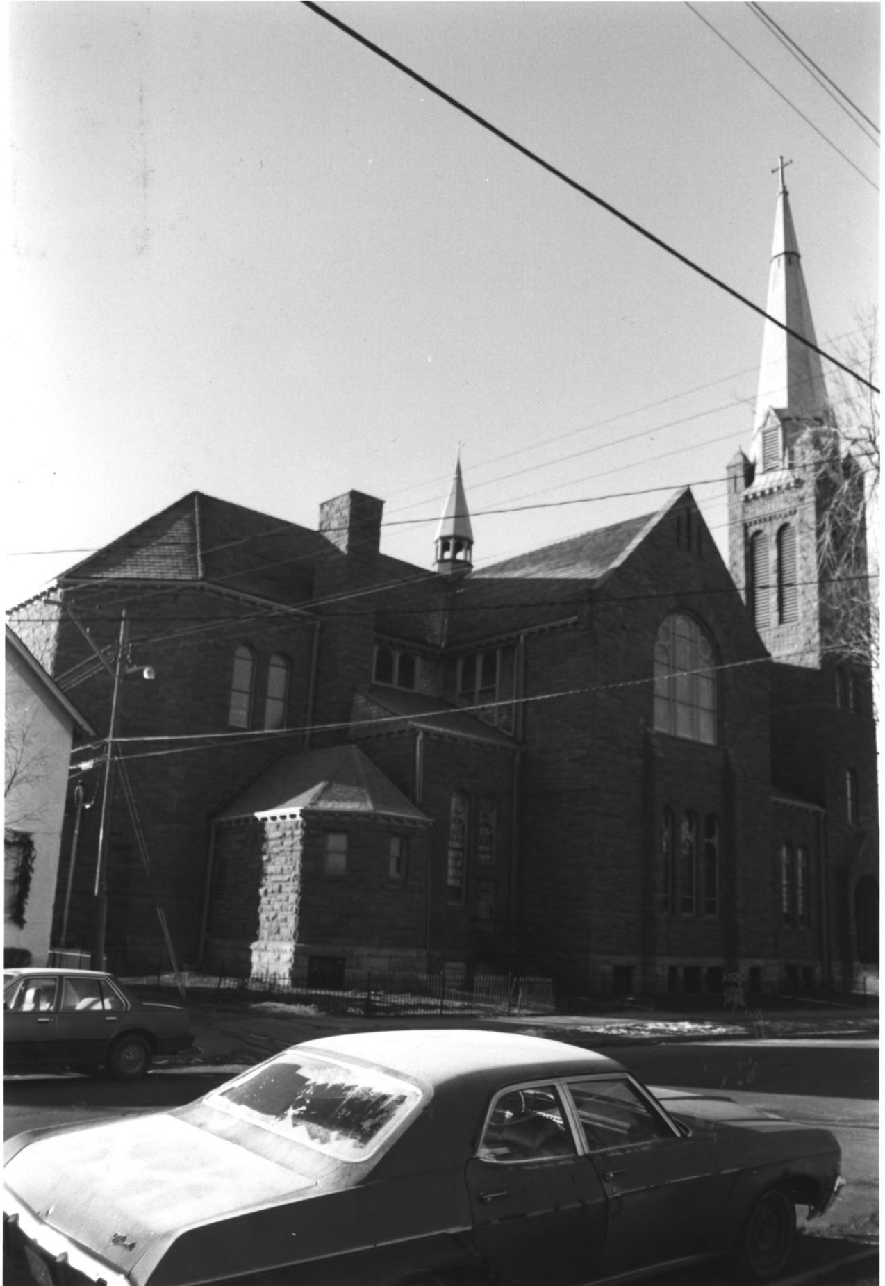
St. Stephen's Church Hennepin County, MN 010681-23A
