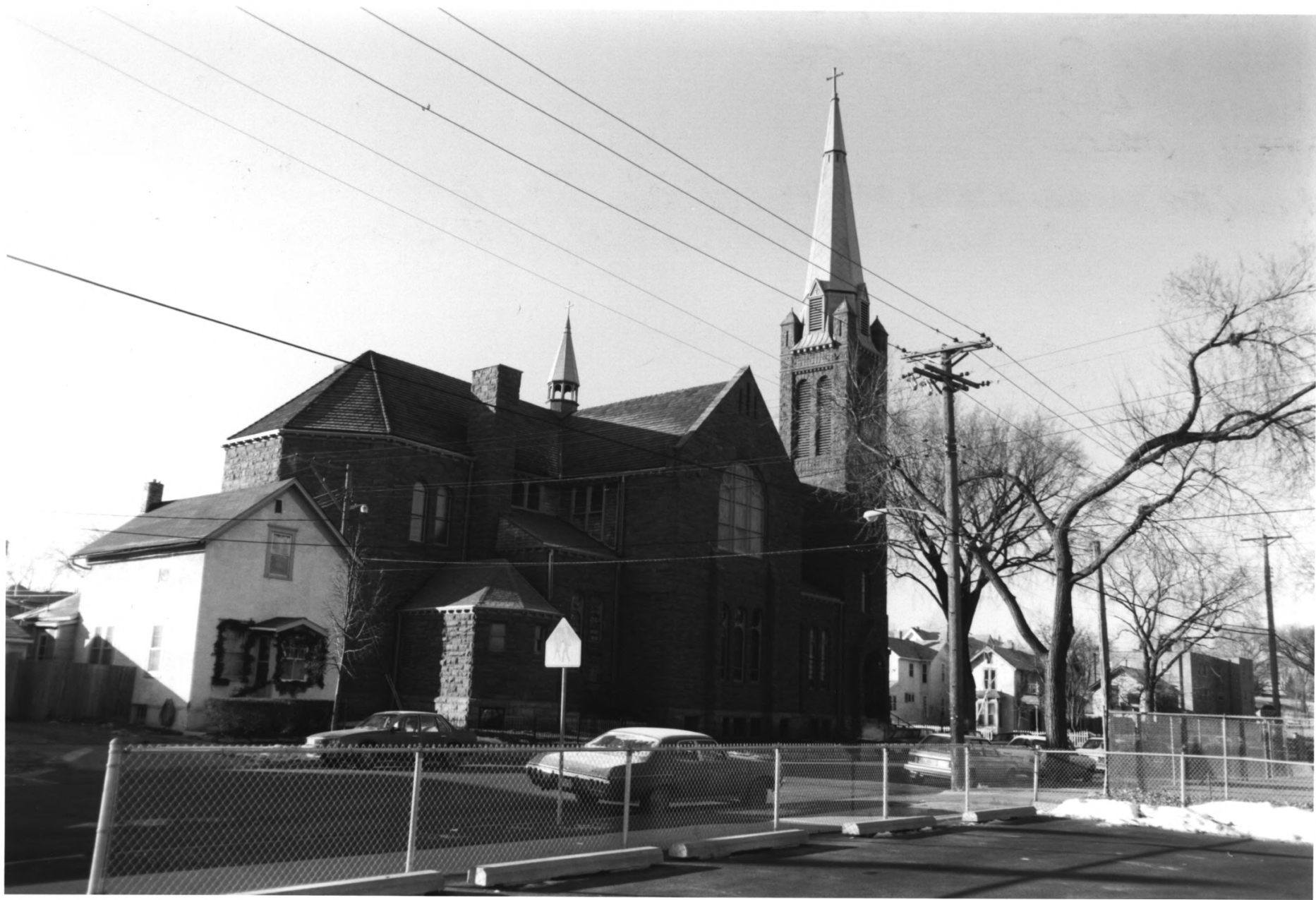
St. Stephen's Church Hennepin County, MN 010681-24A
