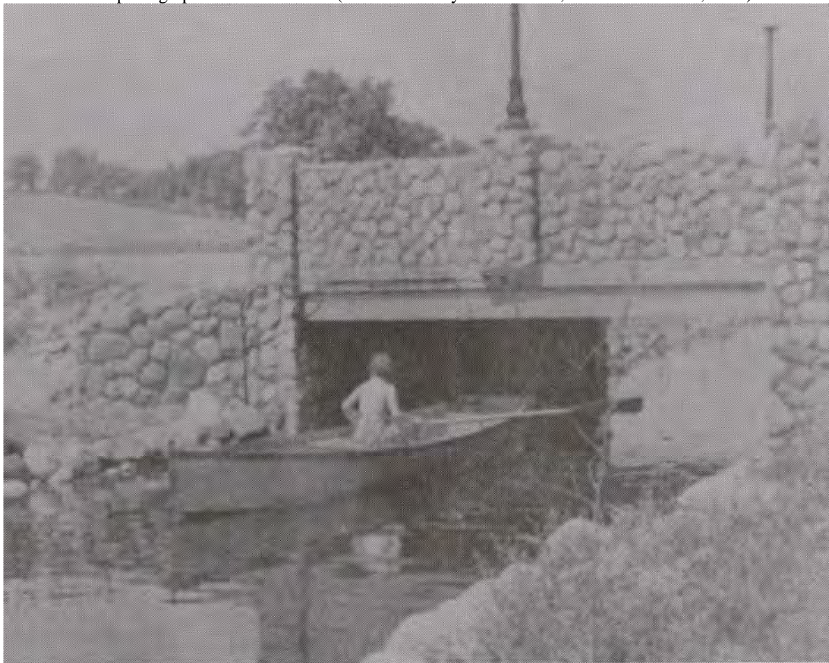
(Attachment D. Lime Lake-Lake Gage Channel and Bridge, c. 1938. Note metal lamps on central pillars of bridge walls (Munger, Lynn, Memories of Steuben County (Marceline, MO: Heritage House Publishing Co., 1997) 36
