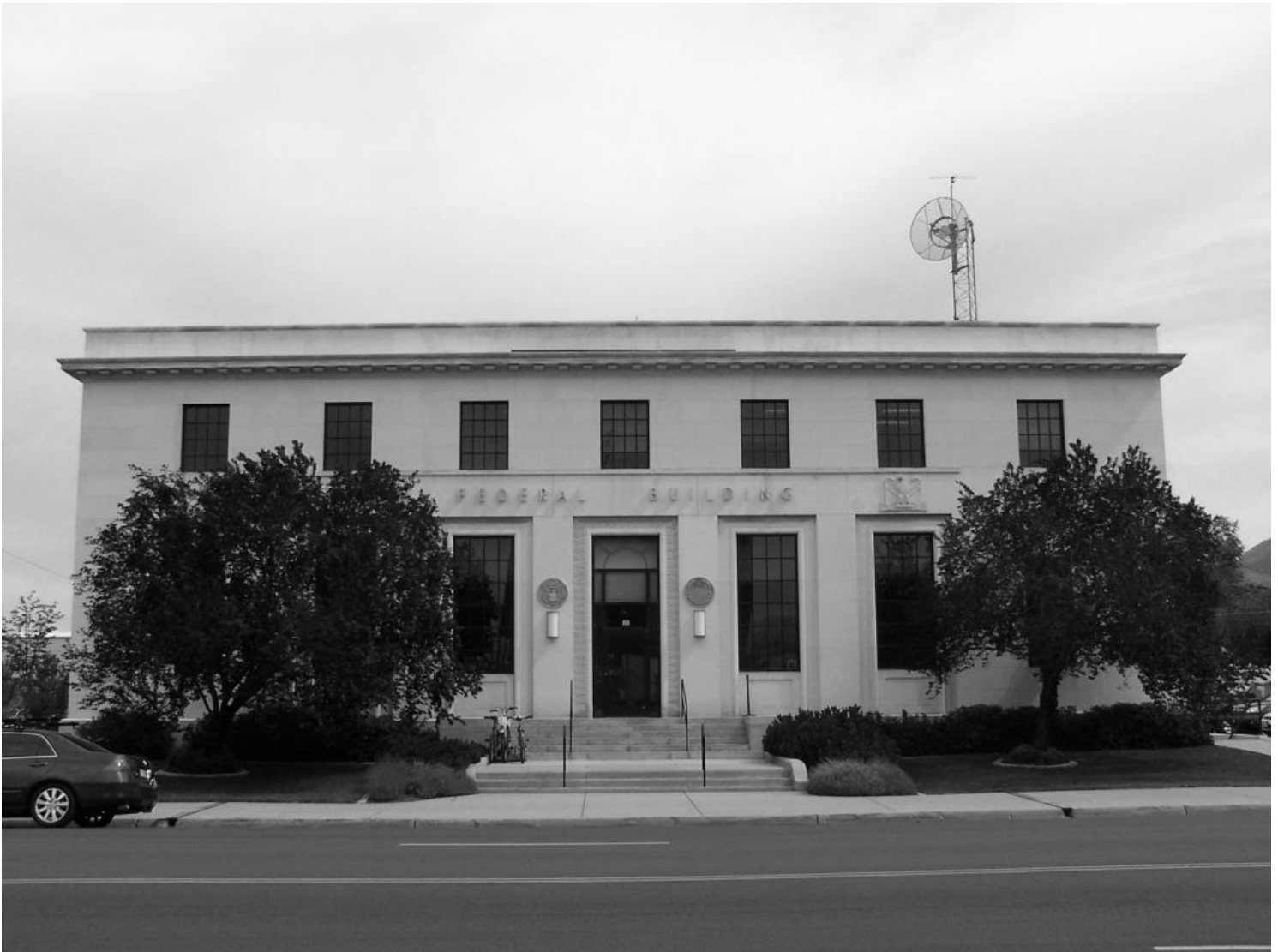
Exterior, primary (south) façade, view north
