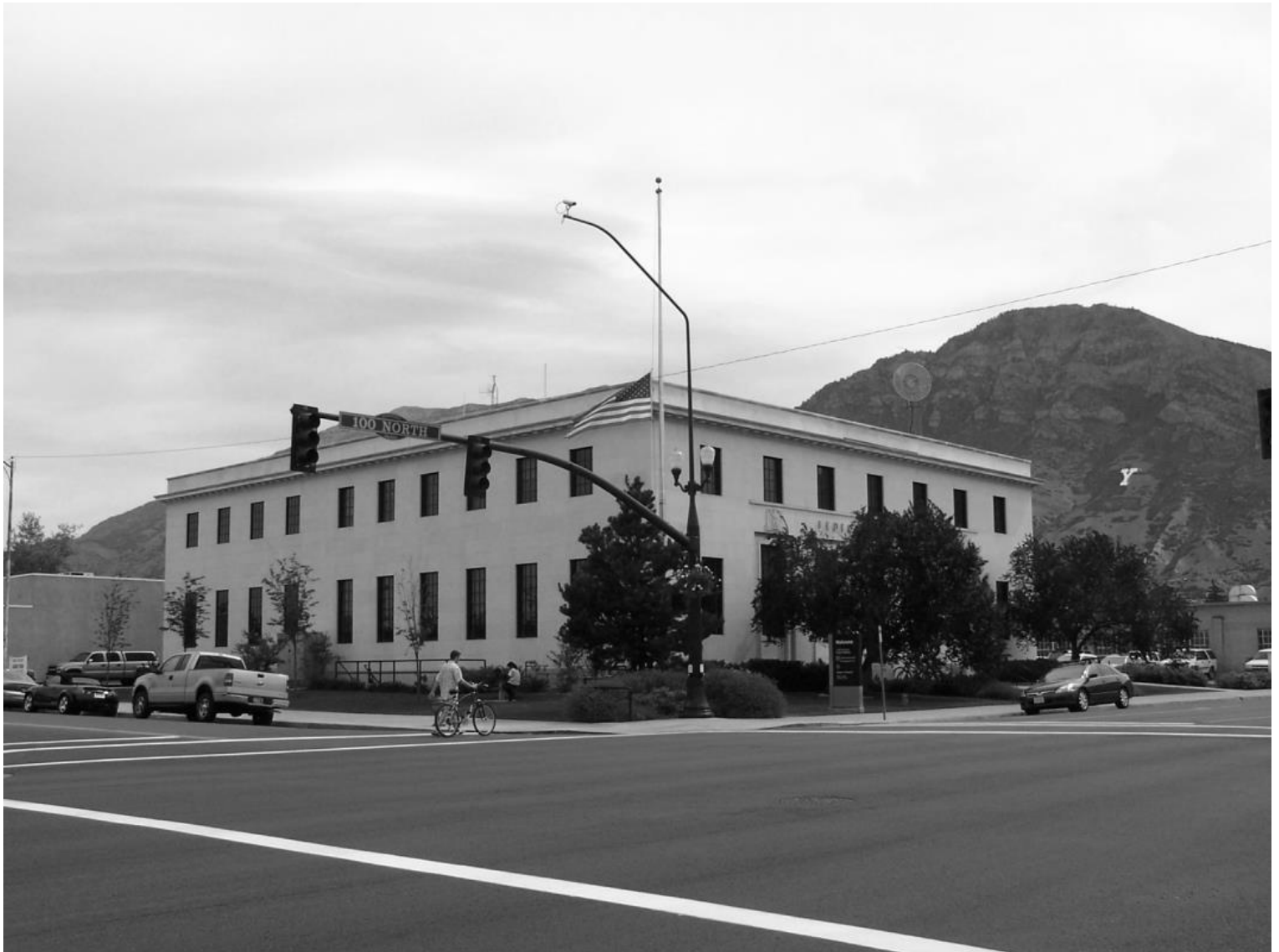
Exterior, southwest elevation, view northeast.
