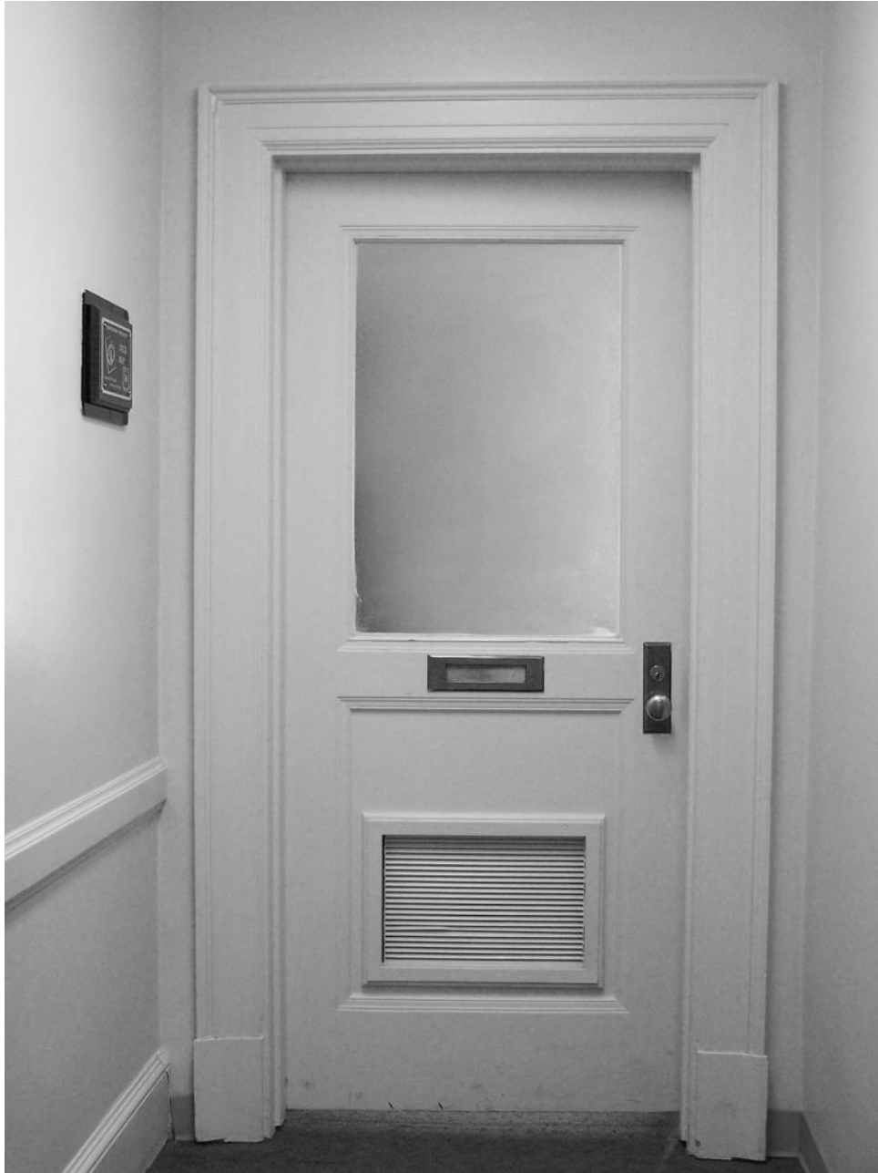
Interior, original wood and glass door
