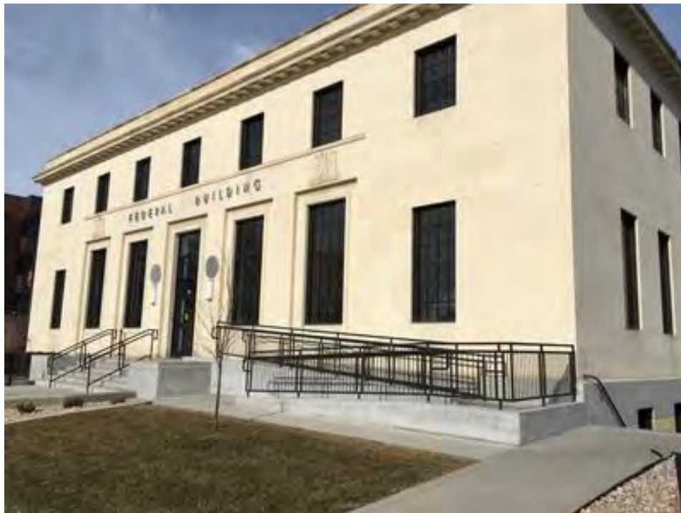
J. Will Robinson Federal Building, Provo, Utah, south elevation looking northwest showing switchback accessibility ramp design with compatible materials, as completed in 2015.
