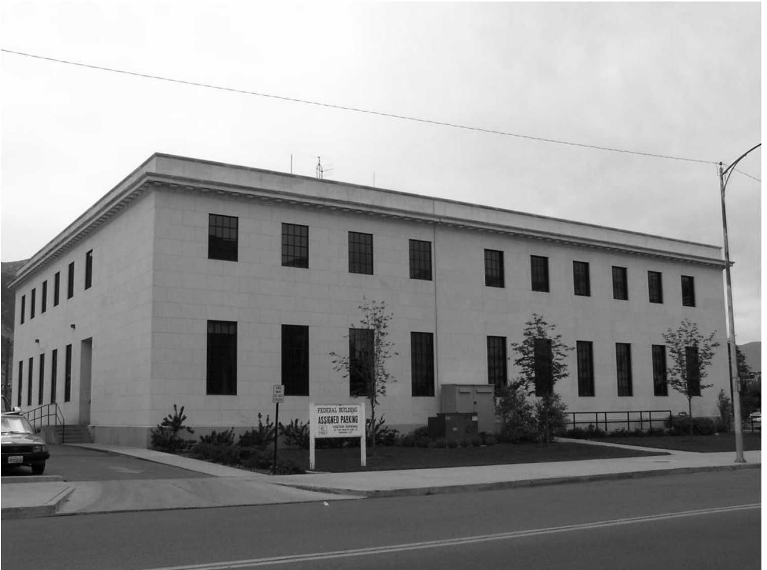
Exterior, west elevation, view east
