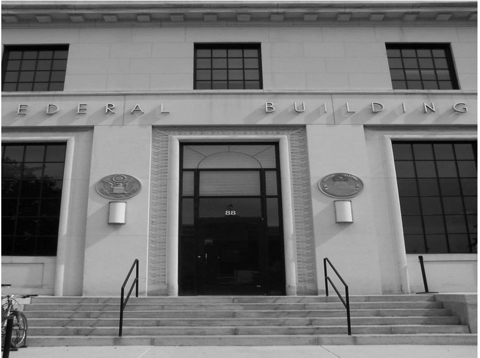
Exterior, detail of entrance on south façade.
