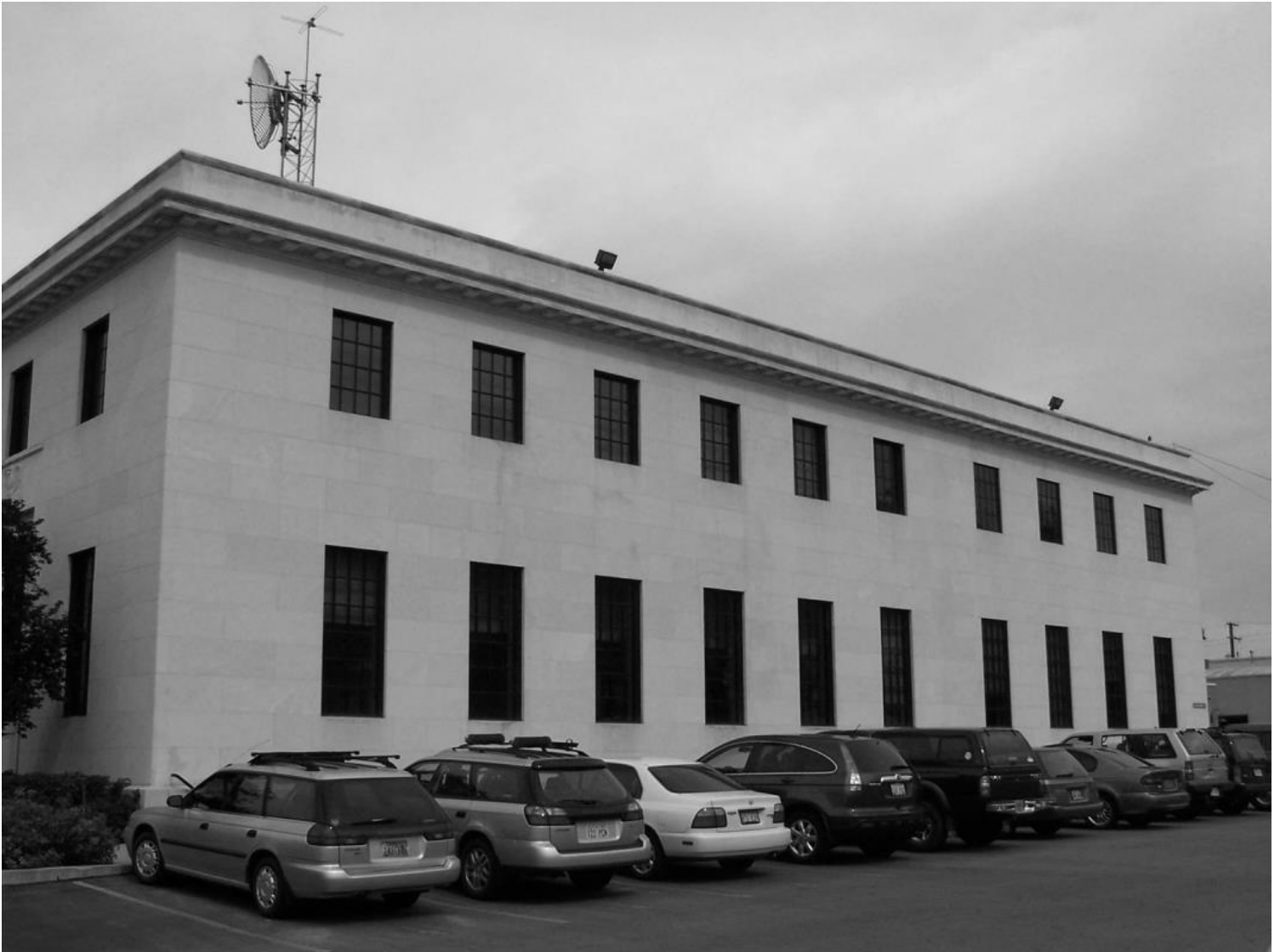
Exterior, east elevation, view west.
