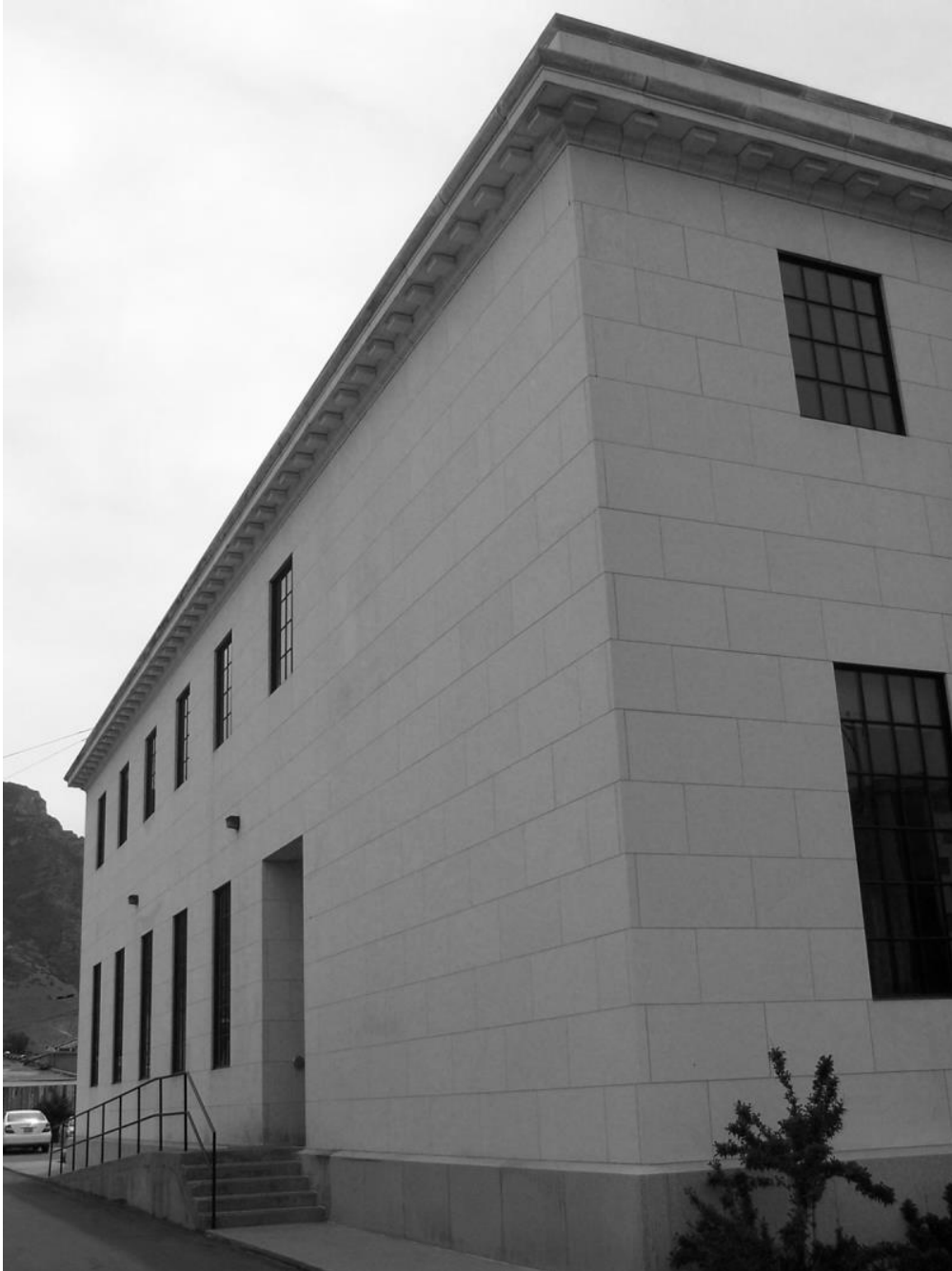
Exterior, rear (north) elevation, view southeast.
