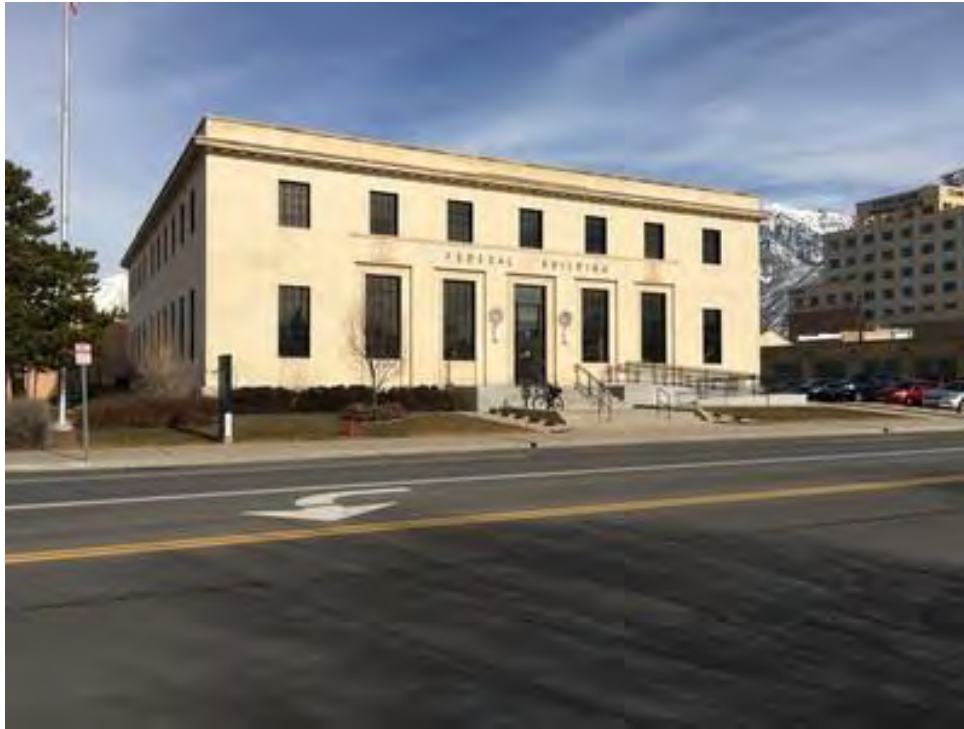
J. Will Robinson Federal Building, Provo, Utah, south elevation looking northeast and showing accessibility ramp as completed in 2015.
