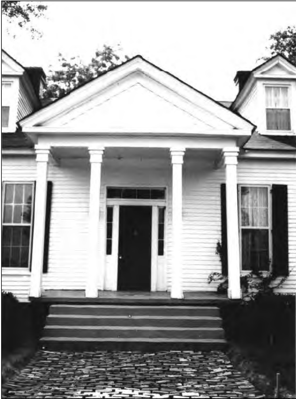
Figure 2: Cedar Grove Front Porch and Door Detail, August 1979. From Cedar Grove National Register Nomination, 1980.
