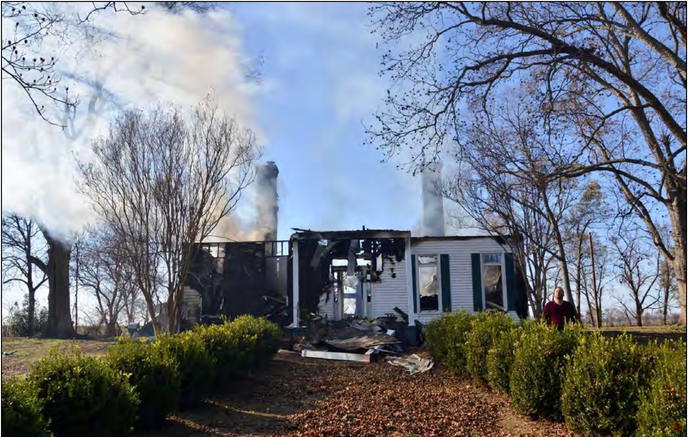
Figure 3: Cedar Grove after a fire, view to the west. Photo from the Brownsville Press , November 29, 2017.
