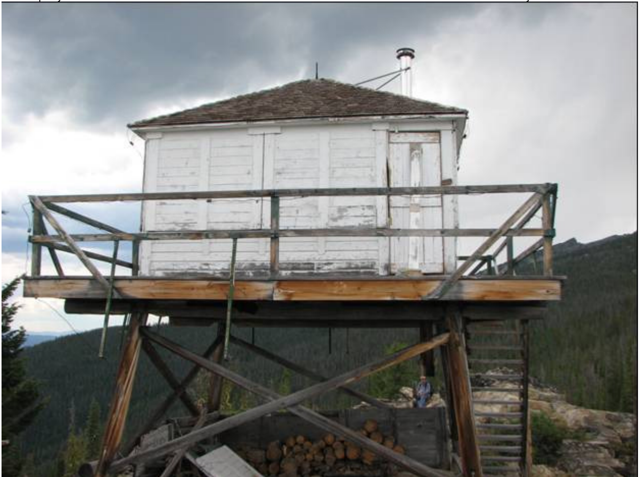
MT_RavalliCounty_BoulderPointLookout_0002. Looking west to the east (front) wall of the lookout.
