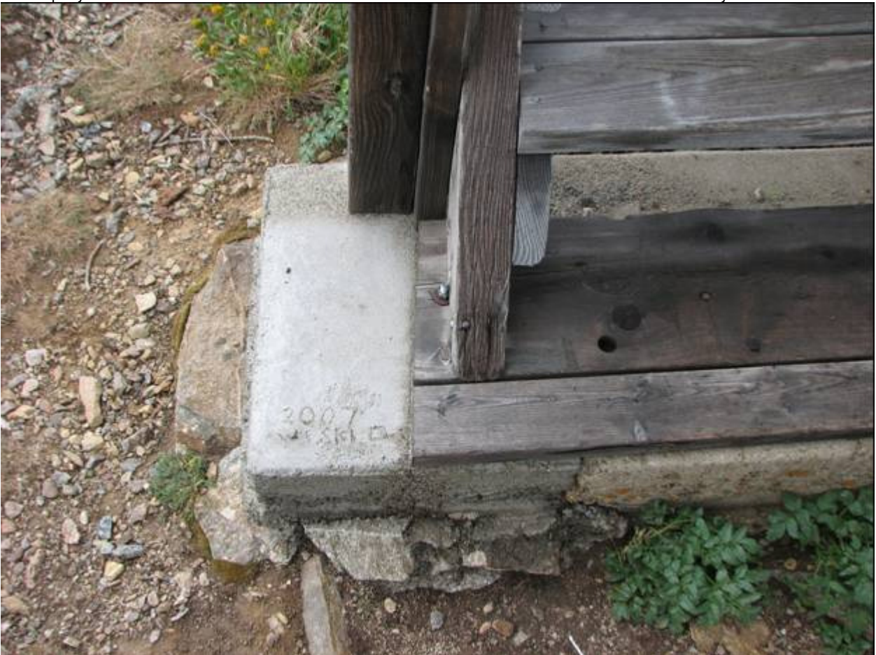
MT_RavalliCounty_BoulderPointLookout_0004. Detail of 2007 concrete footing work done by volunteers.
