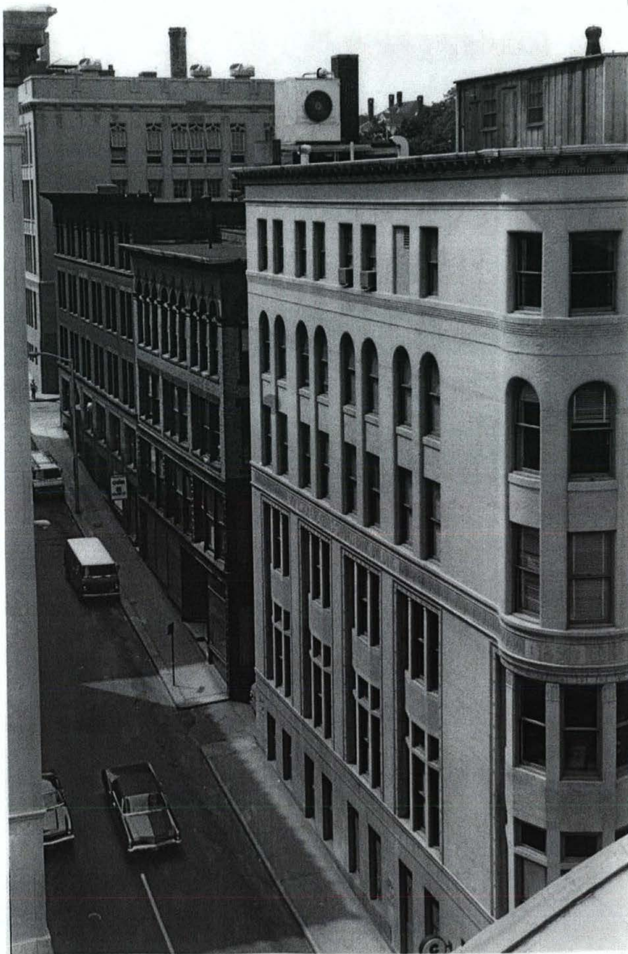
2. Day Building. View of buildings on Walnut Street. (Photographer: Ronald White, 1978)
