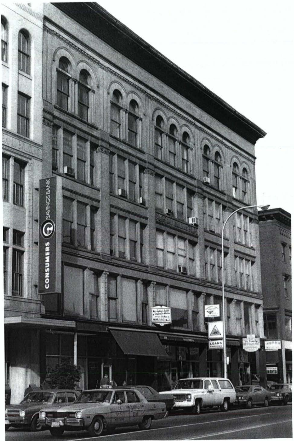
1. Day Building. View of Main Street facade. (Photographer: Ronald White, 1978)
