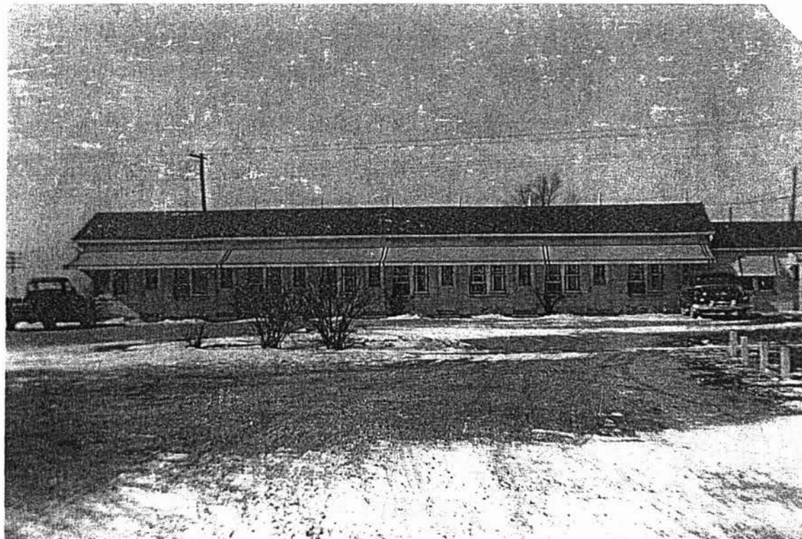
Figure 5: Belevidere Motel after remodeling, ca. 1955 (Photo courtesy of Jean Kranich Heyen).
