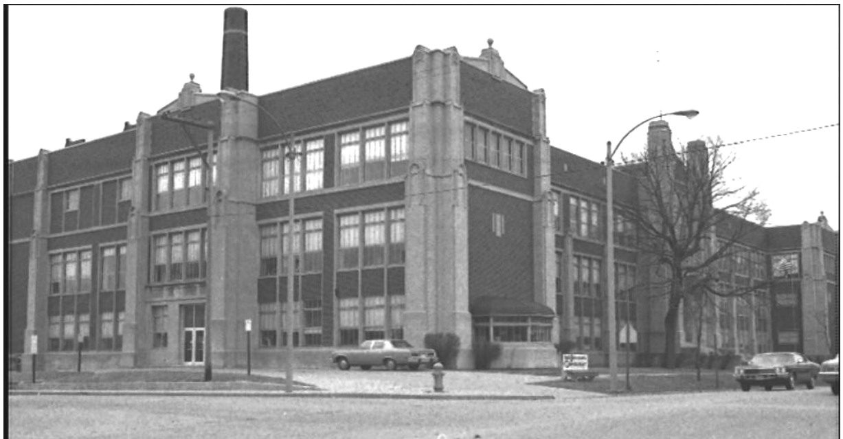
Figure 37: An Illinois State Structures Survey photograph of the Bloomington High School (then the Bloomington Junior High School) looking northeast, circa 1971-1975 (from HARGIS).
