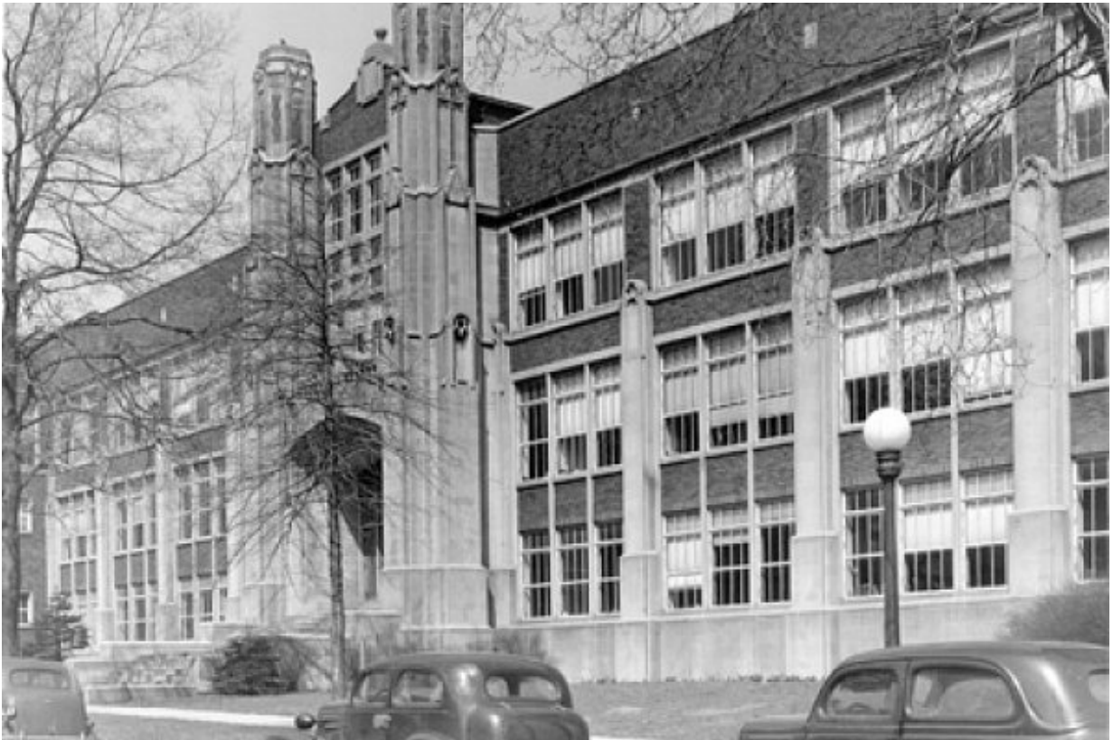
Figure 36: The Bloomington High School, looking northwest, circa 1940s (from www.mchistory.org ; accessed August 20, 2017).
