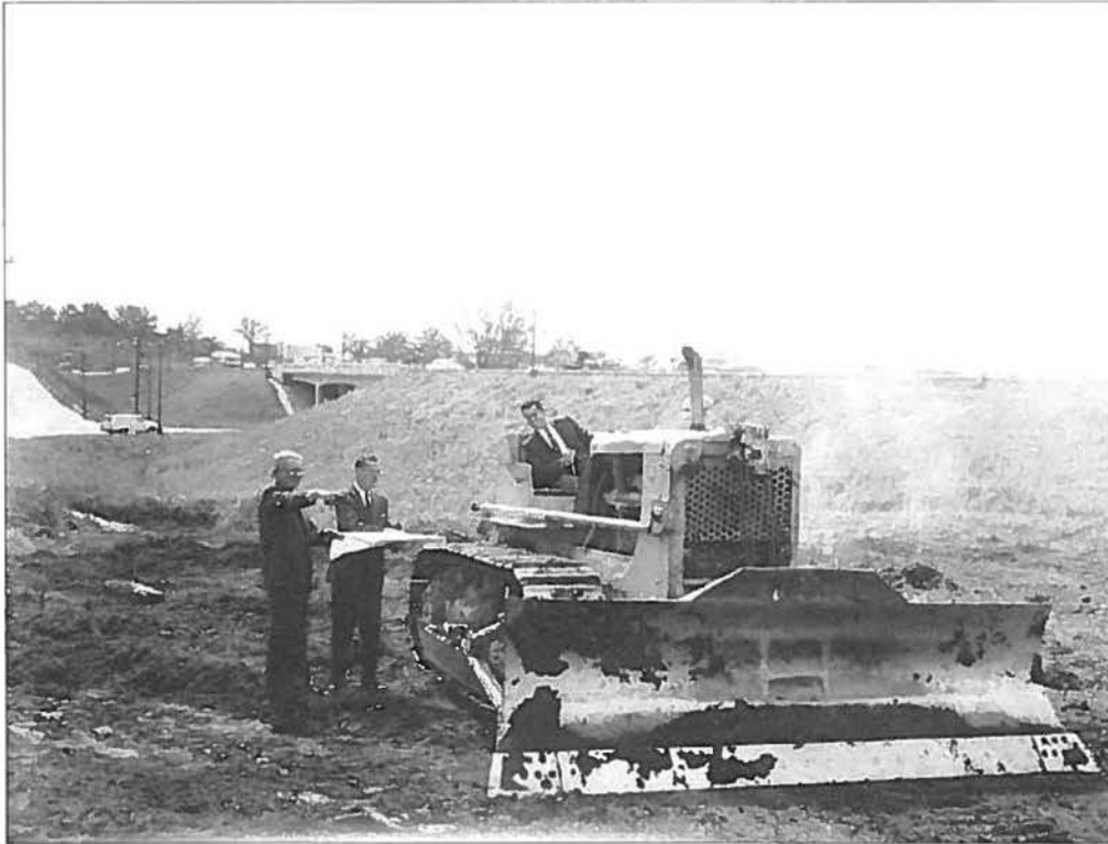
Figure 8. Ground Breaking on Monroe Drive branch, Atlanta, Georgia, May 15, 1961. LBCB108-042a, Lane Brothers Commercial Photographers Photographic Collection, 1920-1976. Photographic Collection, Special Collections and Archives, Georgia State University Library.
