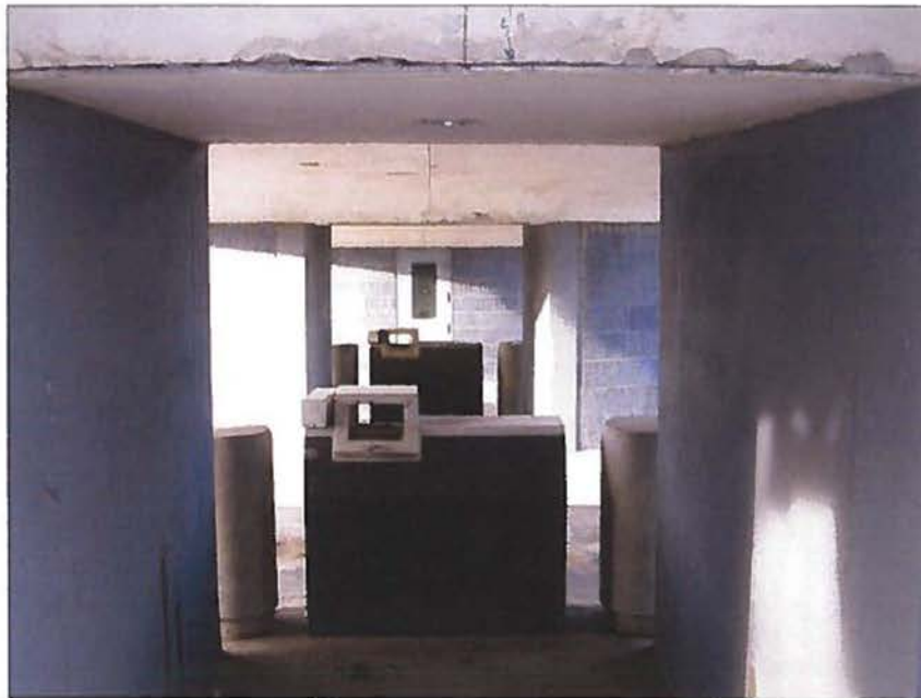
Figure 19. View west through altered teller kiosks, c. 2004 The two nearest kiosks have been adapted for use with a pneumatic tube system connecting customers with the main building teller window. Photo from www.atlantatimemachine.com (Greg Germani).
