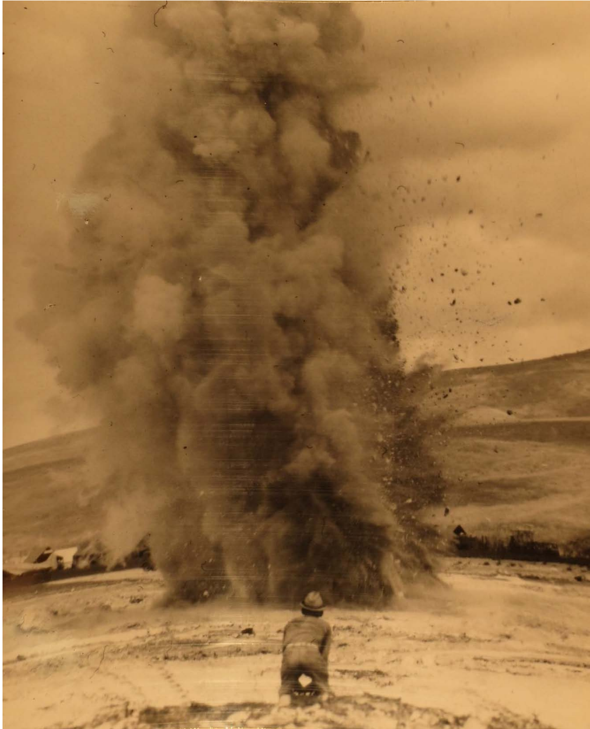
Figure 7 of 42 – Blasting Trees for Ewa Runway (Source: NARA)
