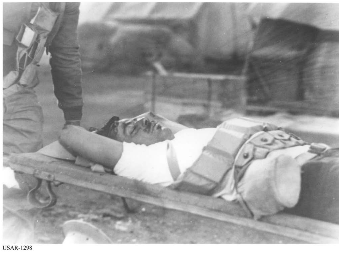
Figure 39 of 42 – Injured Ewa Marine, December 7, 1941 (Source: NPS)
