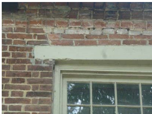
Photo 5: Flemish Bond brickwork
