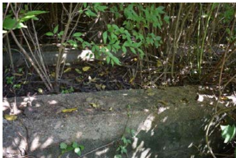
Poured Concrete Cistern--Photo 29
