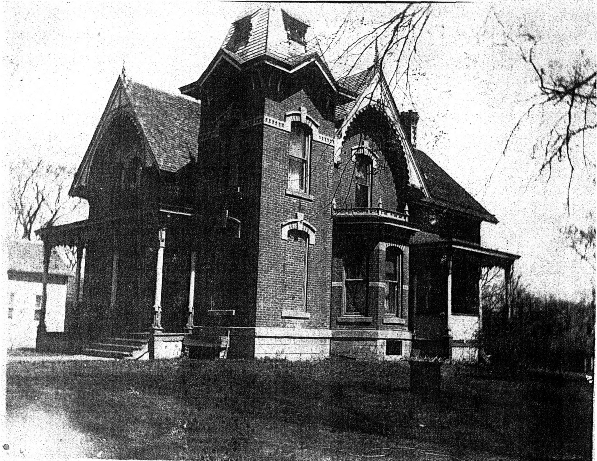
C.H. Norton House Avoca, Pottawattamie County, Iowa Source: Private collection of Brian McCutchen Circa 1920
