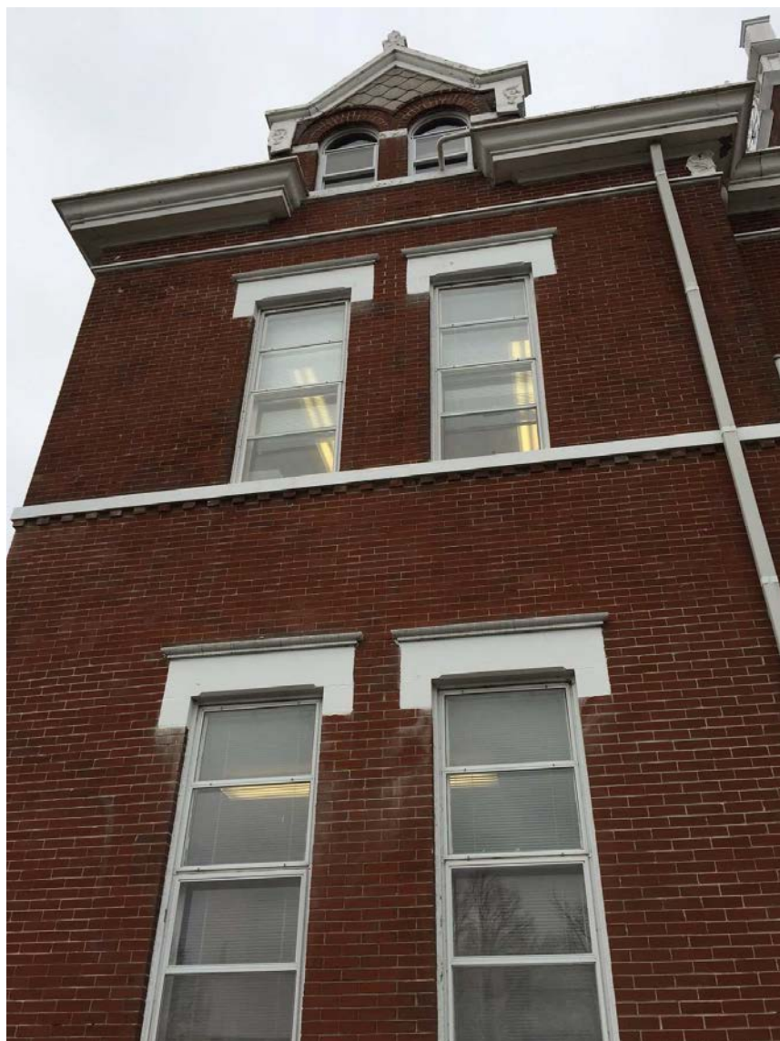
Figure 23. Photograph showing west bay of north elevation of courthouse. Source: Rachel Barnhart, March 2016.
