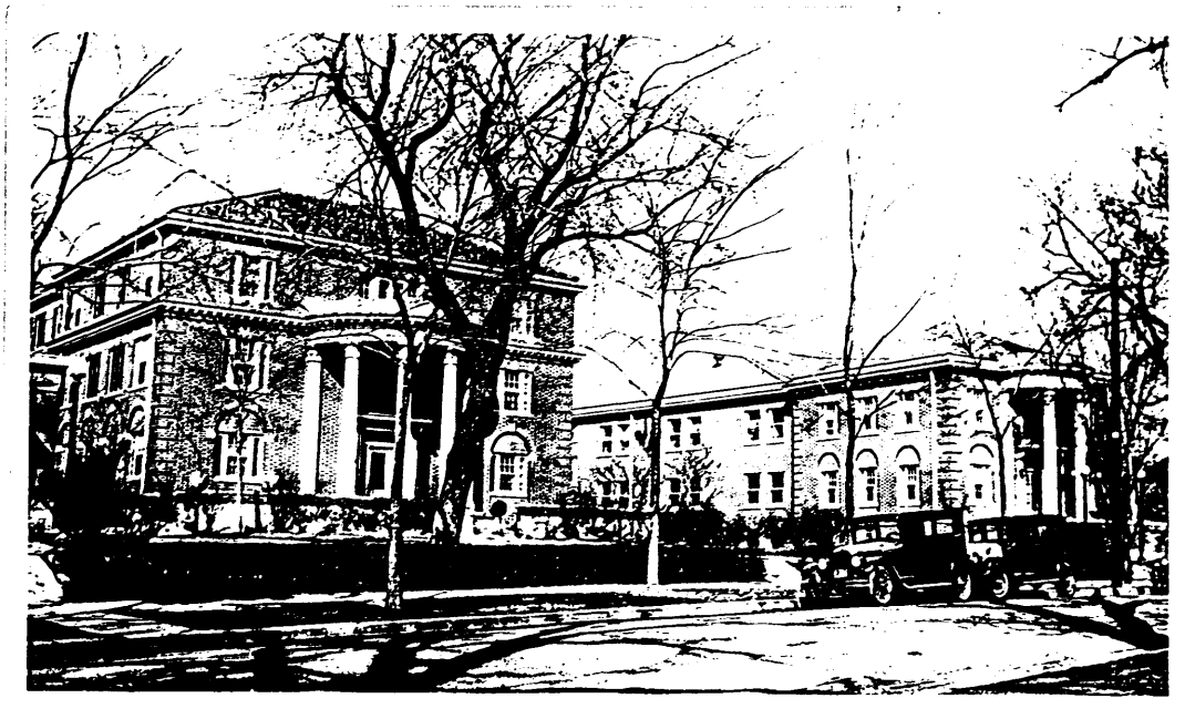
Figure 5. The Patient Apartment Building (left) and Clinical Building appear in this circa 1926-27 view northwest across Grove Street from Highland Park. SOURCE: Arthur Vos, Jr., photographic collection, Denver, Colorado.
