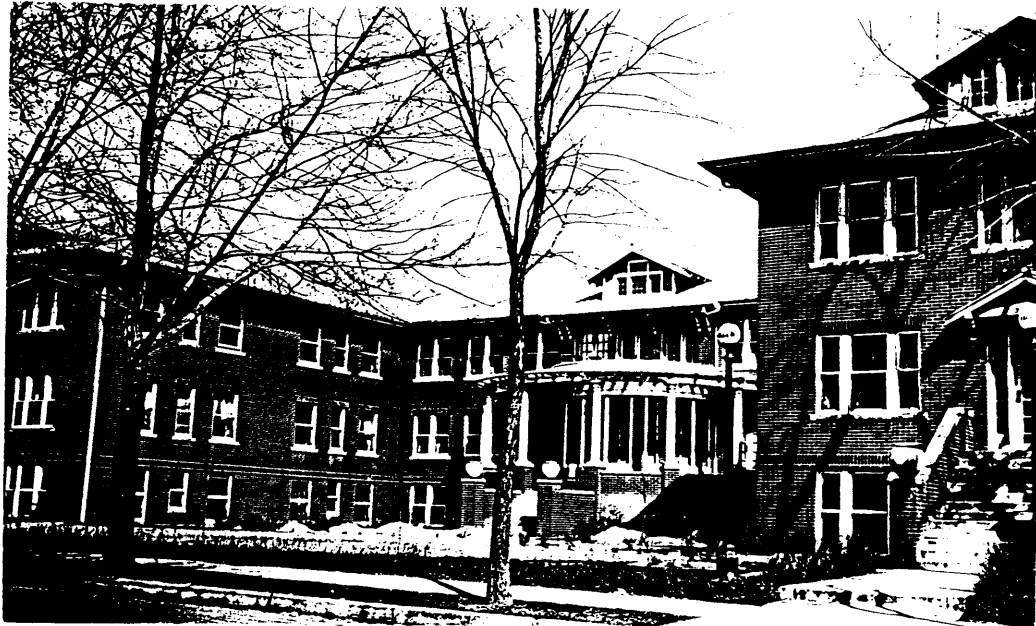
Figure 3. The construction details of the western sunroom are illustrated in this circa 1924 view north of the Main Building. SOURCE: Arthur Vos, Jr., photographic collection, Denver, Colorado.
