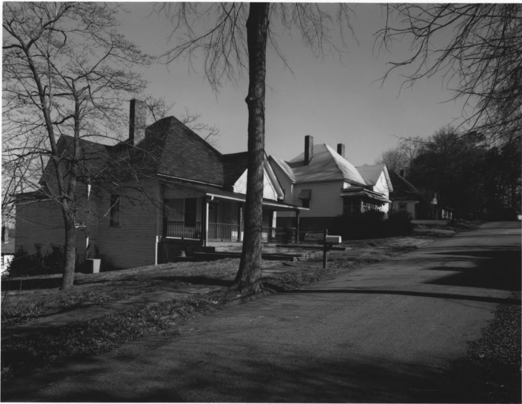
WHITTIER MILLS HISTORIC DISTRICT ATLANTA, FULTON COUNTY, GEORGIA PHOTOGRAPH 20 OF 23
