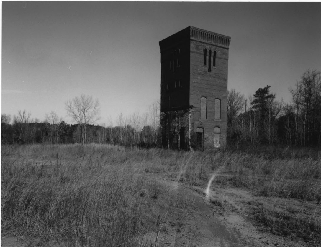
WHITTIER MILLS HISTORIC DISTRICT ATLANTA, FULTON COUNTY, GEORGIA PHOTOGRAPH 11 OF 23
