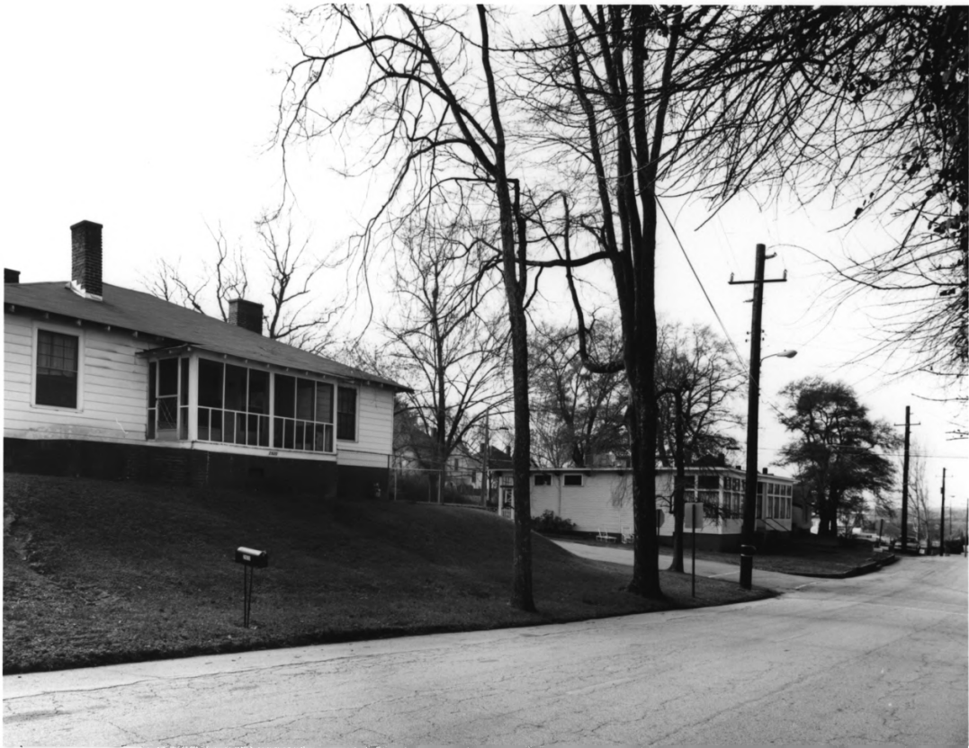
WHITTIER MILLS HISTORIC DISTRICT ATLANTA, FULTON COUNTY, GEORGIA PHOTOGRAPH 18 OF 23
