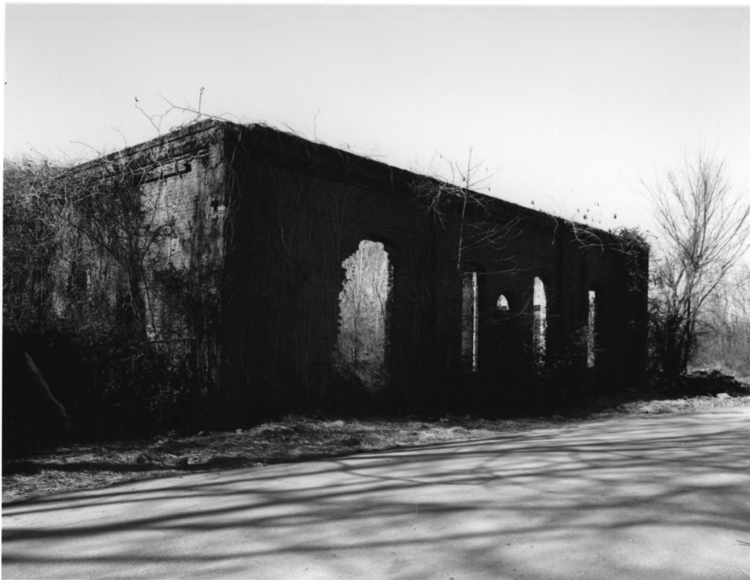
WHITTIER MILLS HISTORIC DISTRICT ATLANTA, FULTON COUNTY, GEORGIA PHOTOGRAPH 12 OF 23
