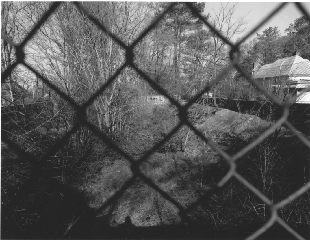
WHITTIER MILLS HISTORIC DISTRICT ATLANTA, FULTON COUNTY, GEORGIA PHOTOGRAPH 21 OF 23
