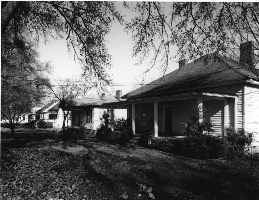
WHITTIER MILLS HISTORIC DISTRICT ATLANTA, FULTON COUNTY, GEORGIA PHOTOGRAPH 7 OF 23
