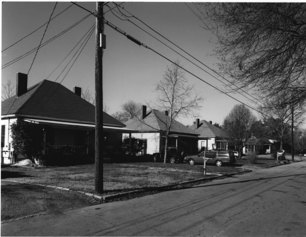
WHITTIER MILLS HISTORIC DISTRICT ATLANTA, FULTON COUNTY, GEORGIA PHOTOGRAPH 8 OF 23
