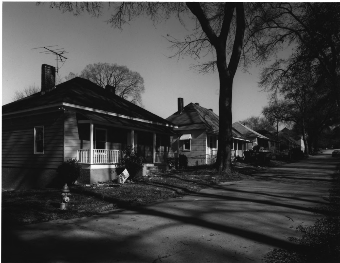
WHITTIER MILLS HISTORIC DISTRICT ATLANTA, FULTON COUNTY, GEORGIA PHOTOGRAPH 13 OF 23
