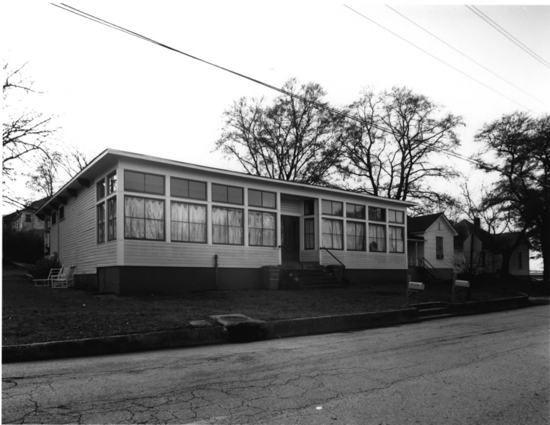
WHITTIER MILLS HISTORIC DISTRICT ATLANTA, FULTON COUNTY, GEORGIA PHOTOGRAPH 16 OF 23
