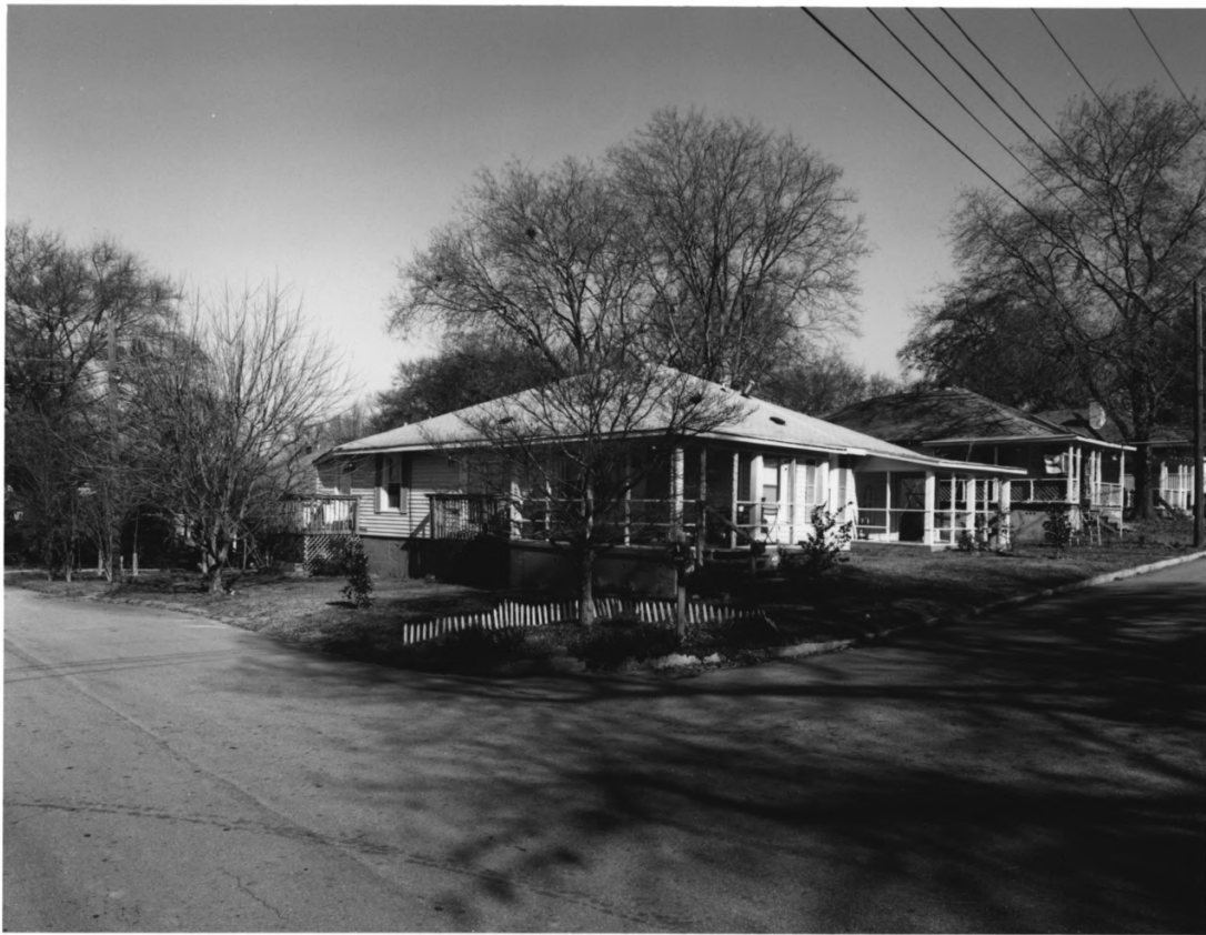
WHITTIER MILLS HISTORIC DISTRICT ATLANTA, FULTON COUNTY, GEORGIA PHOTOGRAPH 6 OF 23
