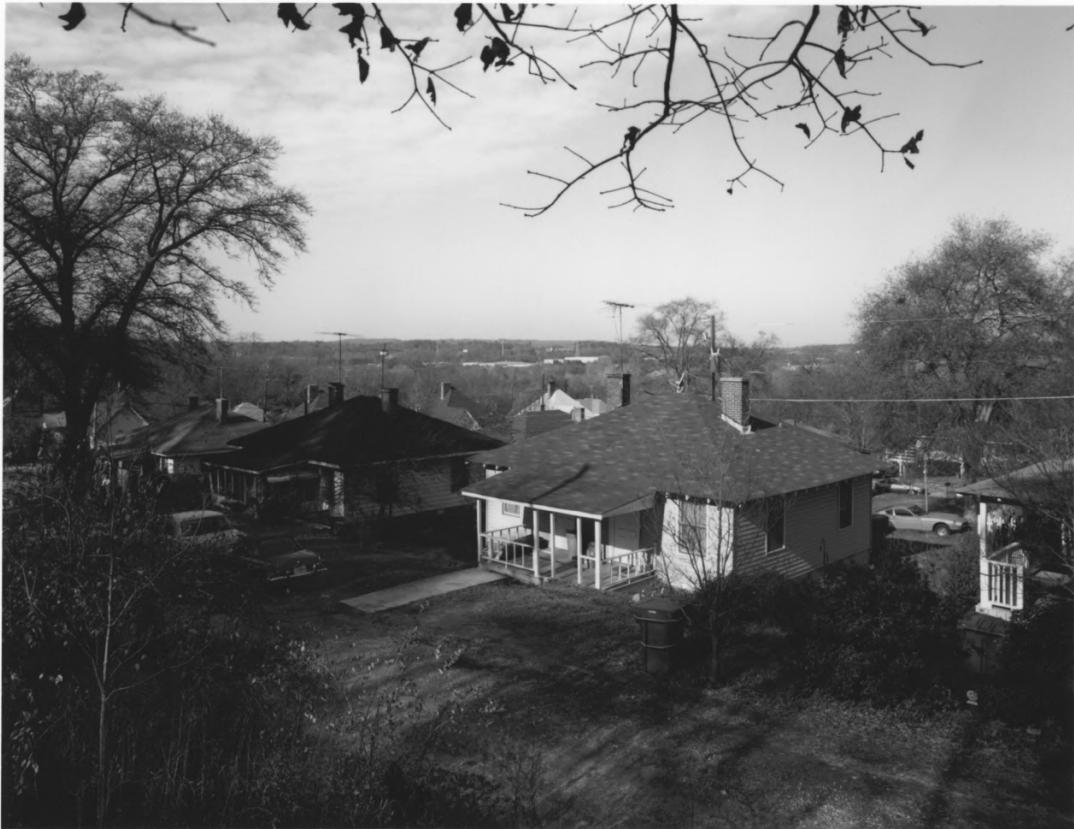
WHITTIER MILLS HISTORIC DISTRICT ATLANTA, FULTON COUNTY, GEORGIA PHOTOGRAPH 3 OF 27
