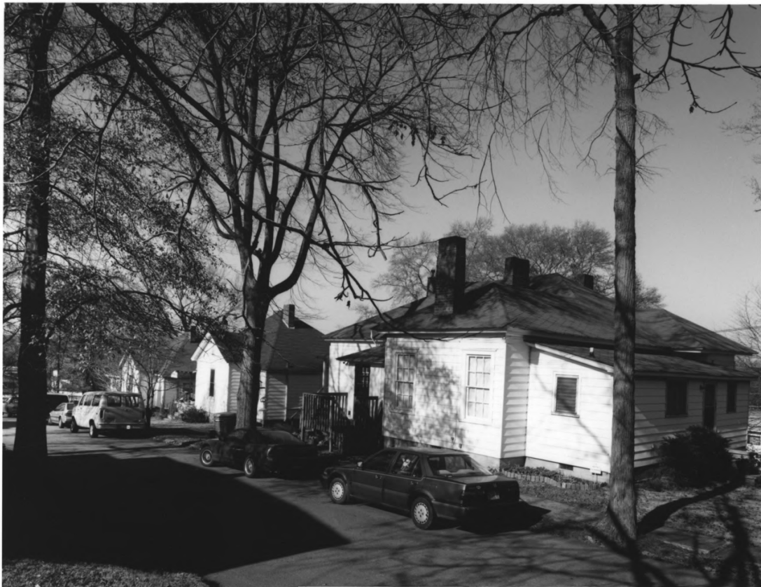
WHITTIER MILLS HISTORIC DISTRICT ATLANTA, FULTON COUNTY, GEORGIA PHOTOGRAPH 19 OF 23
