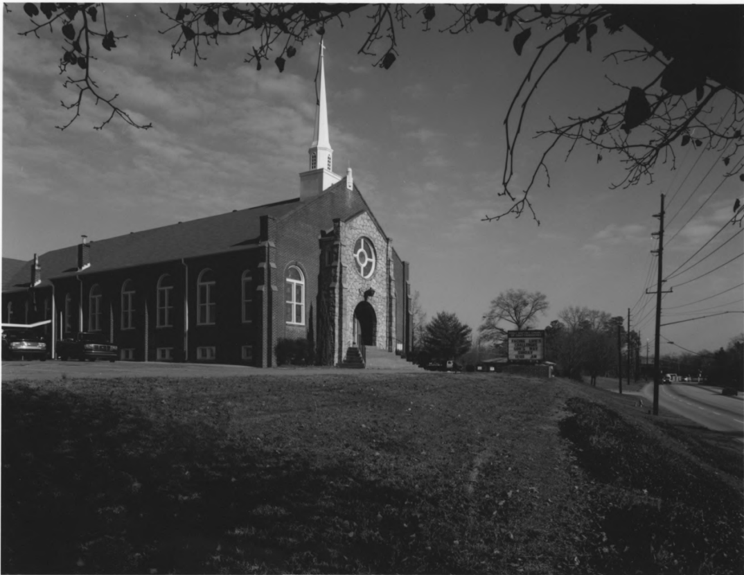
WHITTIER MILLS HISTORIC DISTRICT ATLANTA, FULTON COUNTY, GEORGIA PHOTOGRAPH 1 OF 23
