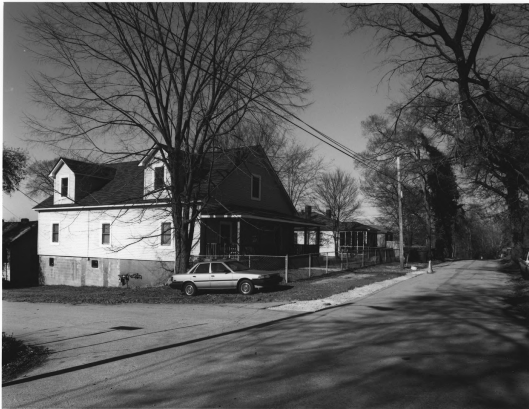
WHITTIER MILLS HISTORIC DISTRICT ATLANTA, FULTON COUNTY, GEORGIA PHOTOGRAPH 10 OF 23
