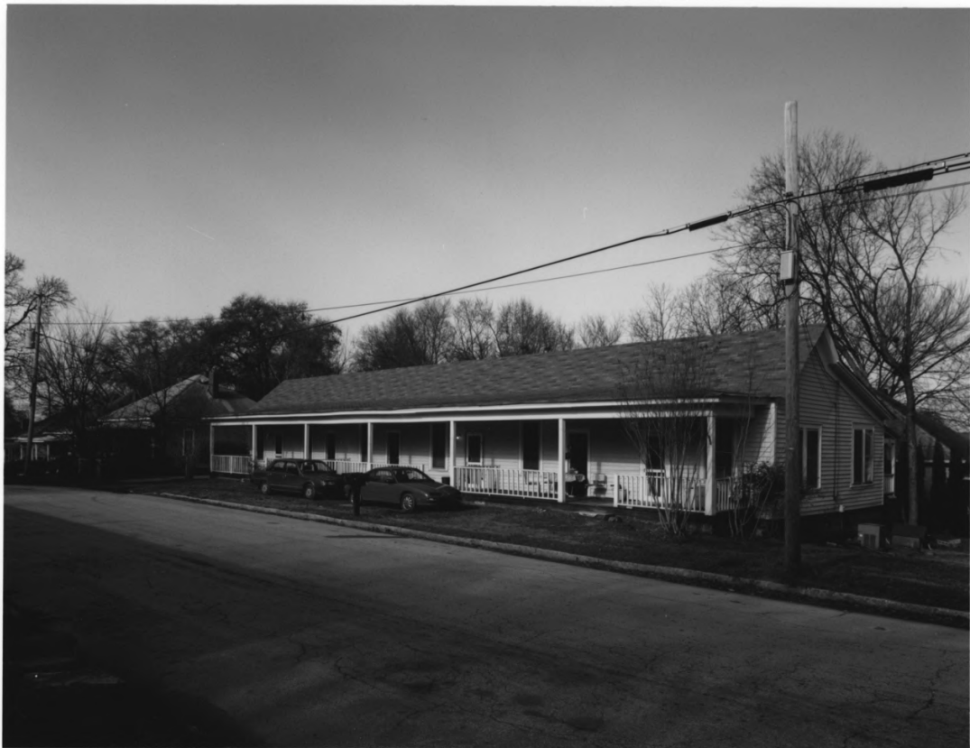
WHITTIER MILLS HISTORIC DISTRICT ATLANTA, FULTON COUNTY, GEORGIA PHOTOGRAPH 17 OF 23
