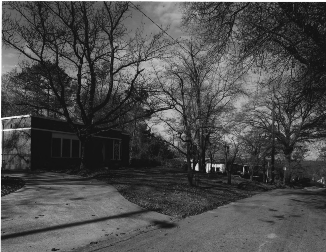
WHITTIER MILLS HISTORIC DISTRICT ATLANTA, FULTON COUNTY, GEORGIA PHOTOGRAPH 2 OF 23
