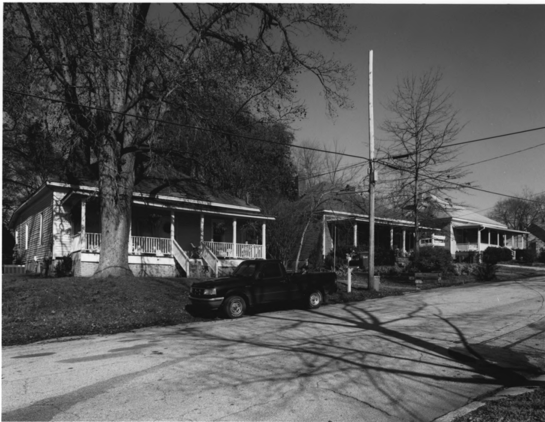
WHITTIER MILLS HISTORIC DISTRICT ATLANTA, FULTON COUNTY, GEORGIA PHOTOGRAPH 15 OF 23
