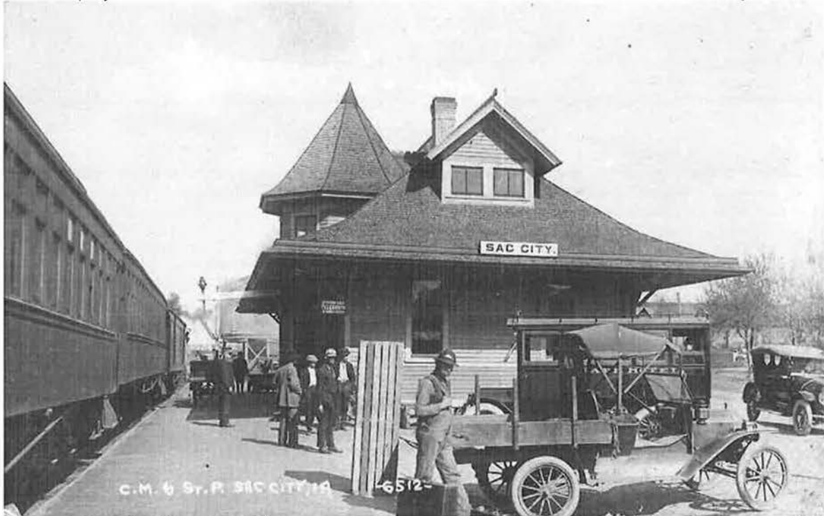
Image 16: Building the Chicago, Milwaukee, and St. Paul depot in Sac City provided some of the impetus for C & NW to upgrade their depot. (non-extant) (Photo Perry Collection)
