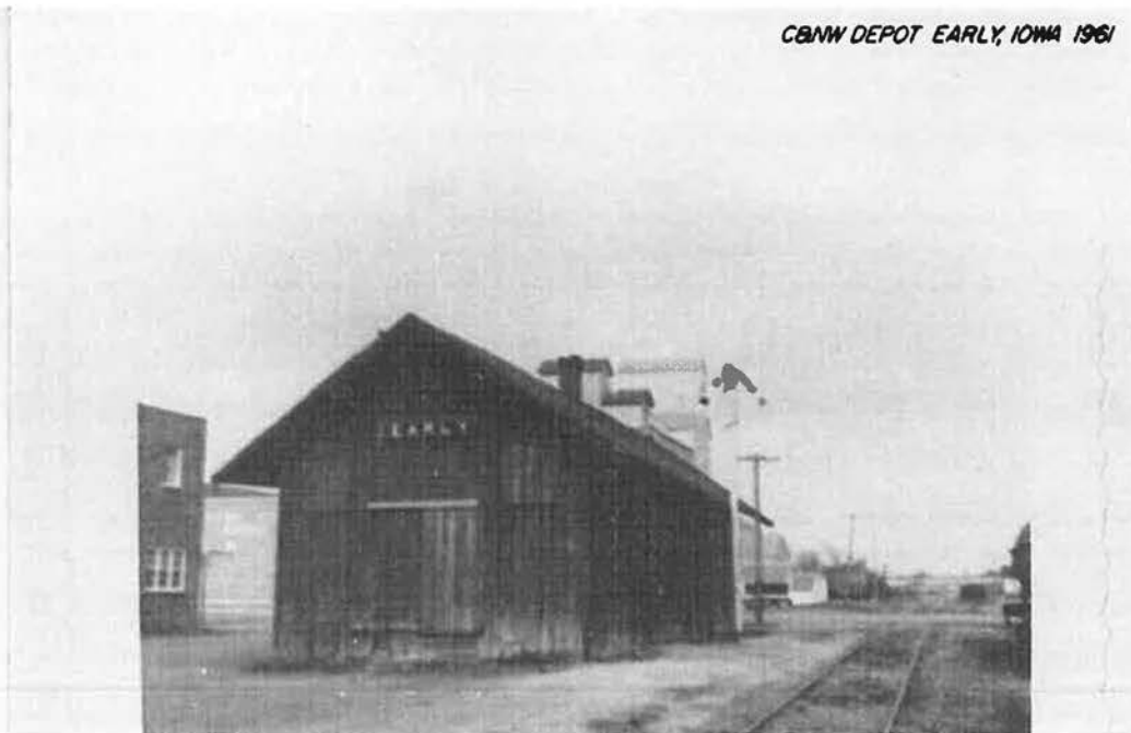
(Image 23) Chicago & North Western Depot in Early, IA, was constructed ca. 1900. The simple design is typical of many early depots in rural Iowa. Photo 1961. (non-extant) (Perry Photo Collection)
