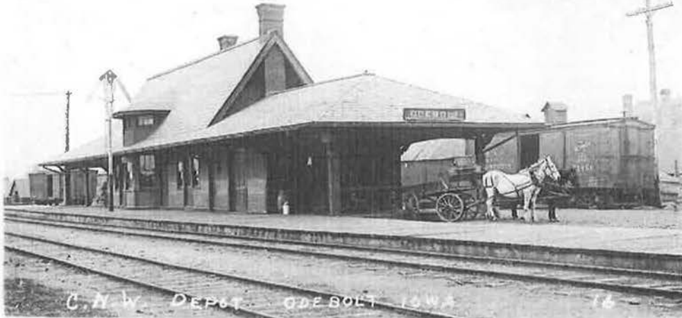
(Image 22) Chicago & North Western Depot in Odebolt, IA ca. 1910. The older design did not feature the characteristic roof line of the standard plan depots. (non-extant) (Photo Perry Collection)
