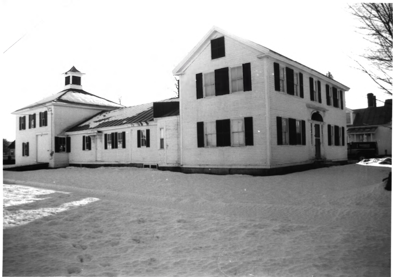
WHITNEY, CAPT JOEL, HOUSE; FRANKLIN CO; MAINE
