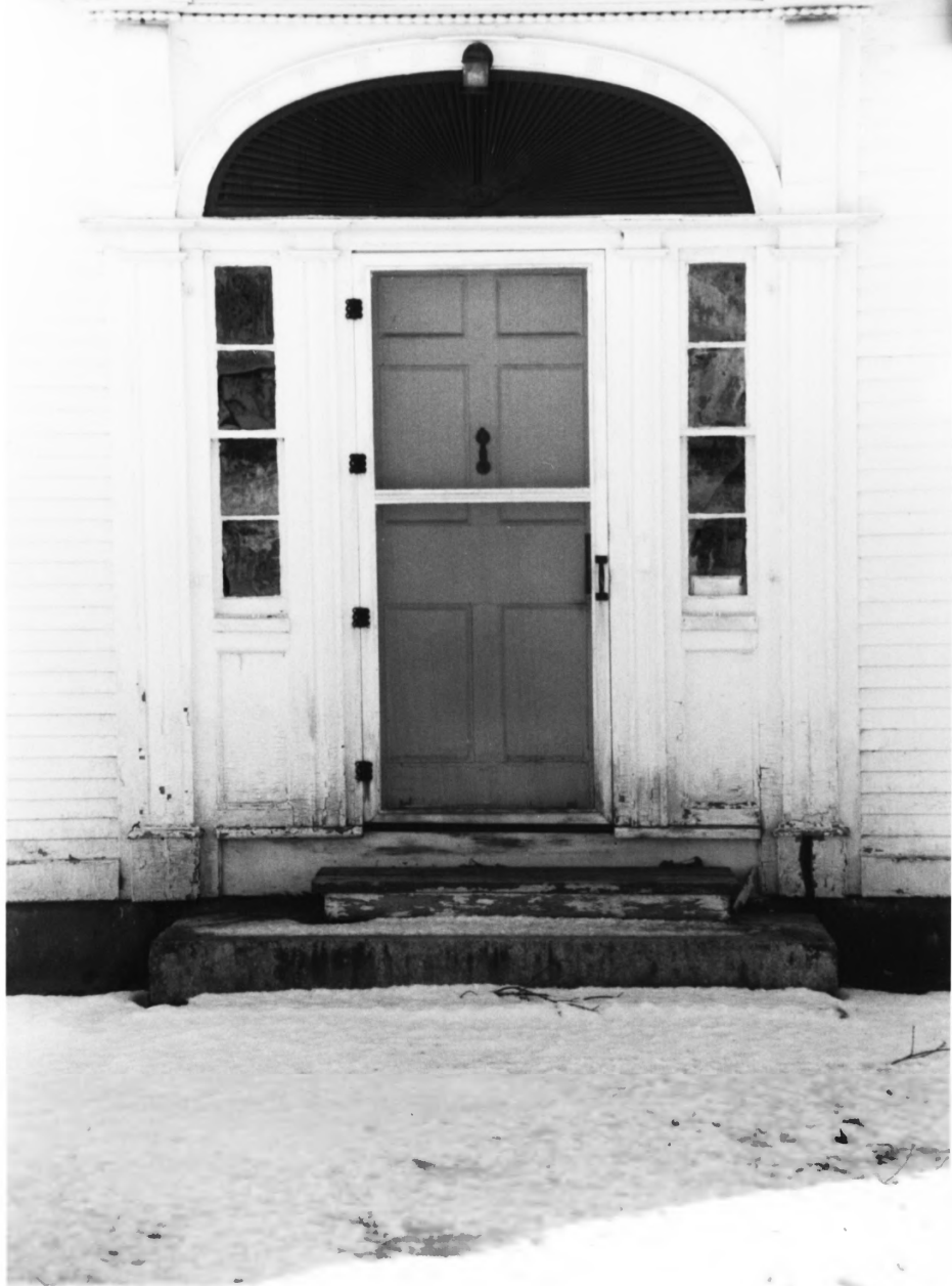
WHITNEY, CAPT. JOEL, HOUSE; FRANKLIN CO., MAINE
