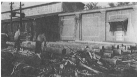
Historic Photograph 2. Minnesota Historical Society log cabin on fair grounds, 1925; men stripping and peeling the logs during construction of the cabin (Minnesota Historical Society).
