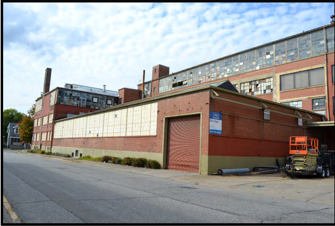
Figure 12. South elevation/Primary facade looking west from Grandview. The east elevation of the 1924 portion of the building can be seen in the background. The ca 1946 one-story addition is visible in the foreground. (Photo 0004).
