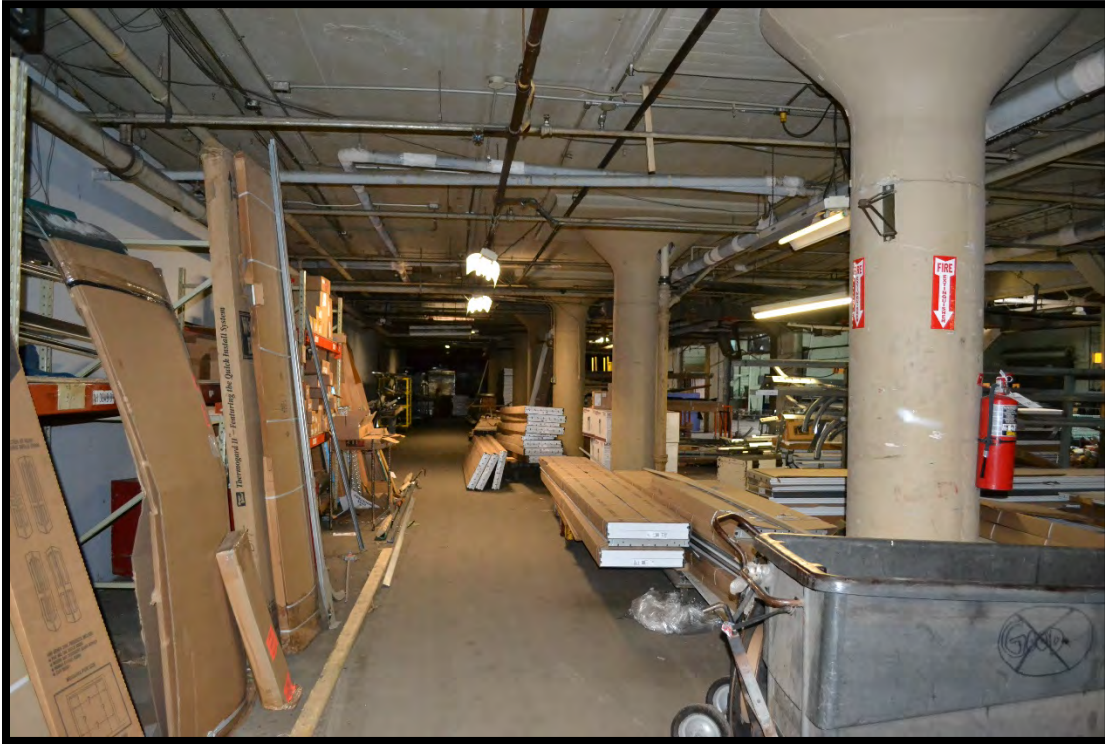
Figure 25. First floor warehouse space, looking east toward 1925/1946 addition. Note the distinctive poured concrete columns found throughout the 1924 and 1925/1946 portions of the building. (Photo 0011).
