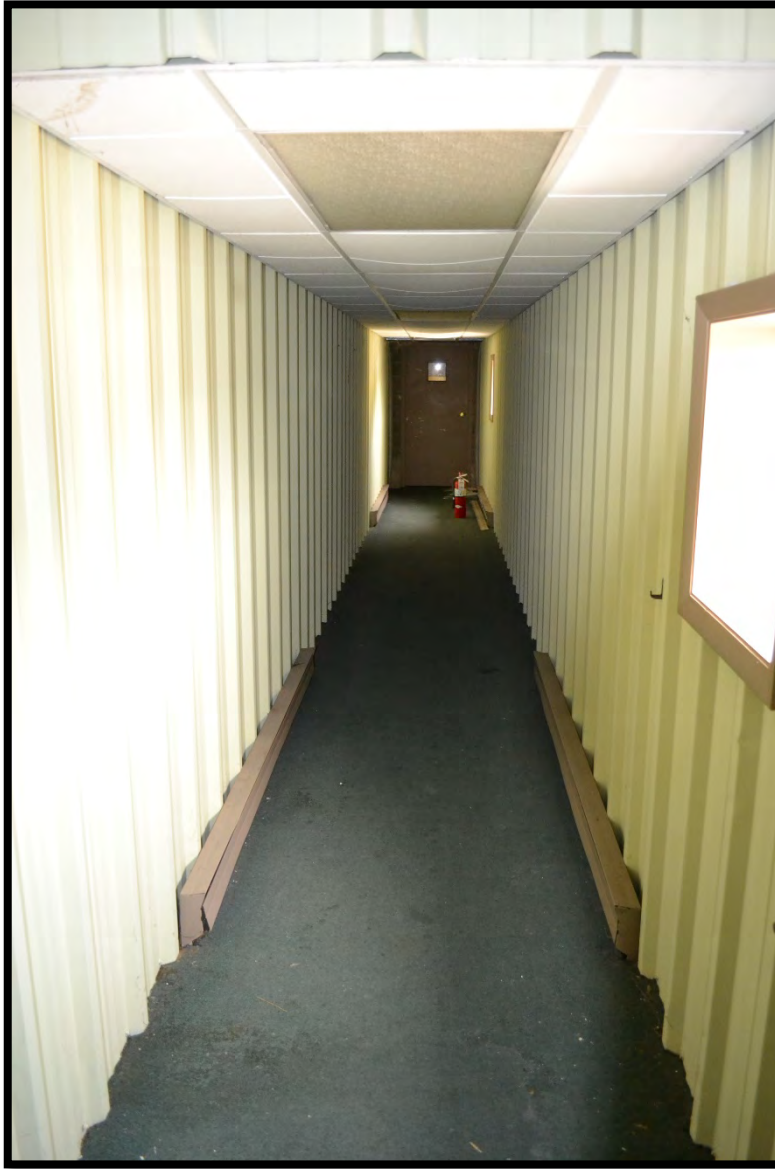
Figure 39. Metal hyphen that formerly connected the second floor of the Grote Building to the second floor of the circa 1970 Kent Company Building, looking east. (Photo 0023). Access is no longer available from this connector structure.
