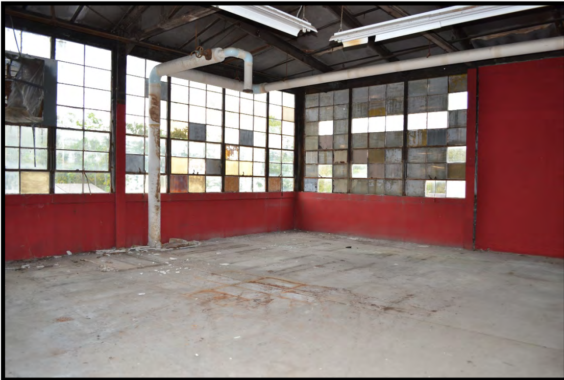
Figure 28. Third floor of 1924 building looking southeast toward rear of this portion of the building. (Photo 0014).
