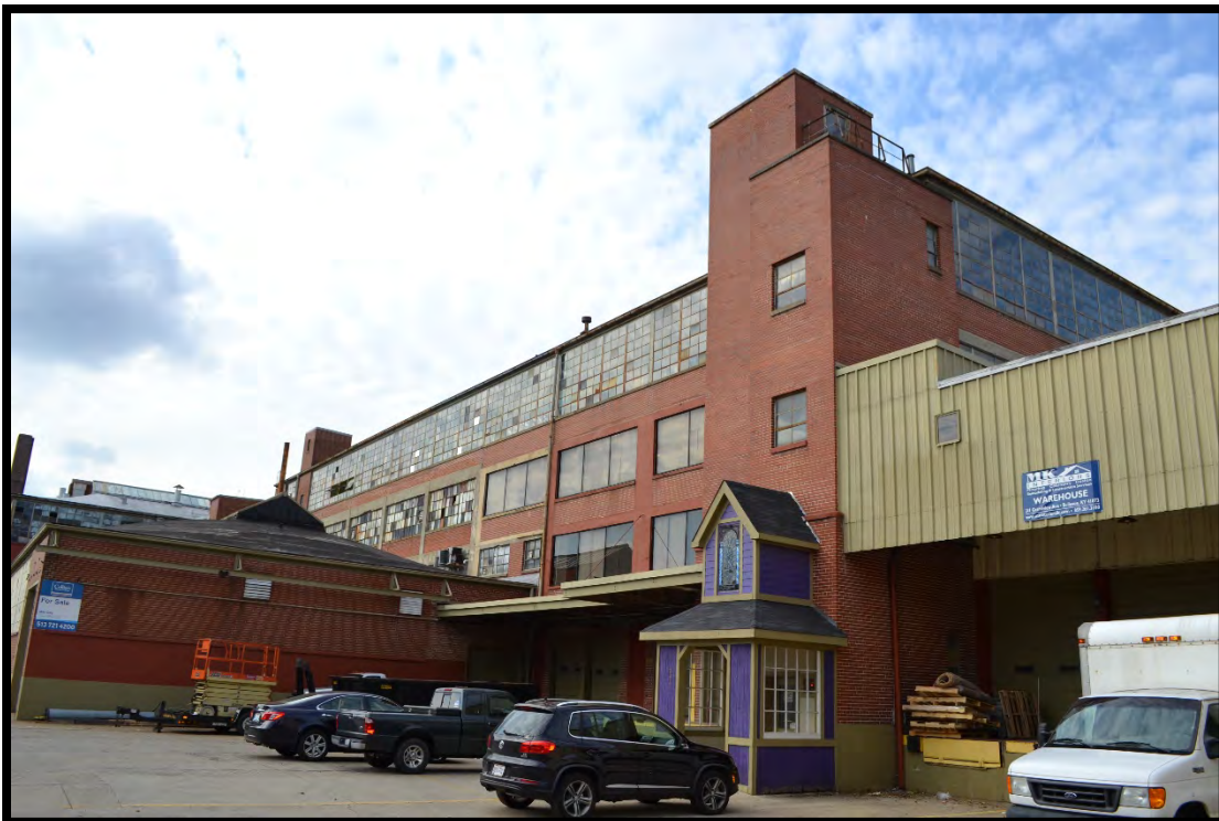
Figure 13. South elevation/Primary façade showing 1925/1946 addition (left in photo) and Kent Co. addition, constructed circa 1980. (Photo 0005).
