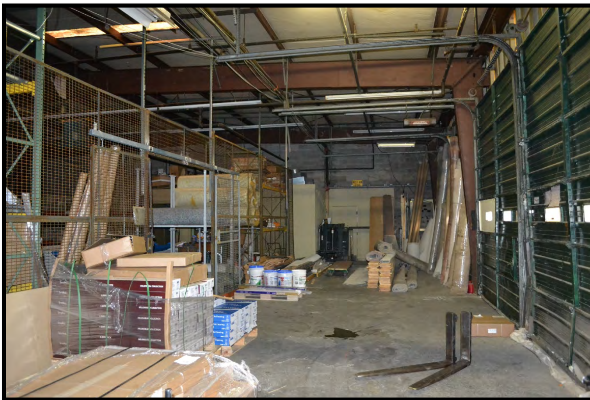
Figure 37. Interior of circa 1980 one-story concrete block building on the first floor, looking east. (Photo 0021).
