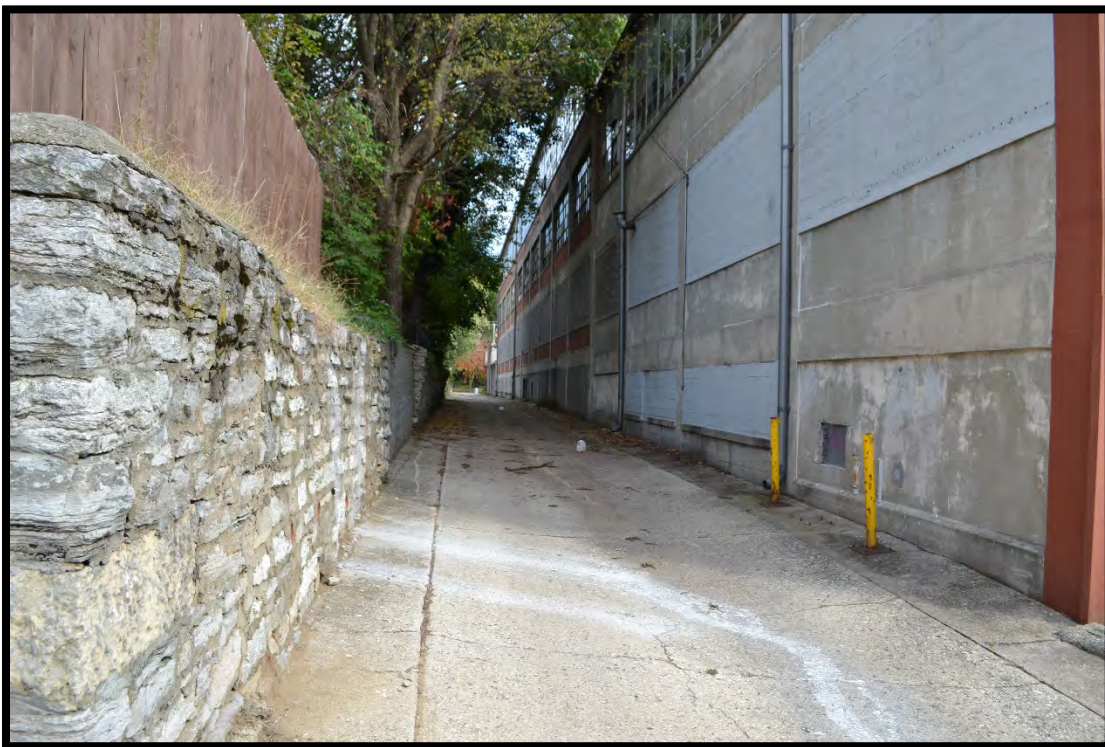
Figure 17. View of rear (north elevation) from intersection of alleyway with Lafayette Avenue, looking east. The 1925/1946 addition is visible in the background. (Photo 0009).
