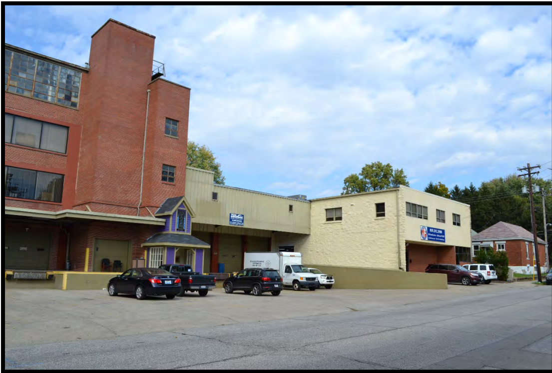
Figure 14. East corner of south elevation/primary facade looking NE. The circa 1980 Kent Co. addition (D) will be kept and utilized as part of this project. There is no longer access between the circa 1980 Kent Co building (middle right) and the circa 1970 commercial building (far right in this photo). (Photo 0006), as described in the text above.
