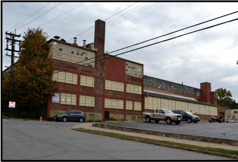
Figure 10. South elevation/Primary facade of Grote building. The 1924 portion of the building is left in this photo (A in Figure 2). The circa 1946 one-story addition can be seen to the right (C in Figure 2). The fourth floor of the 1925/1946 addition is visible directly above the 1946 one-story building (B and C in Figure 2). (Photo 0003).
