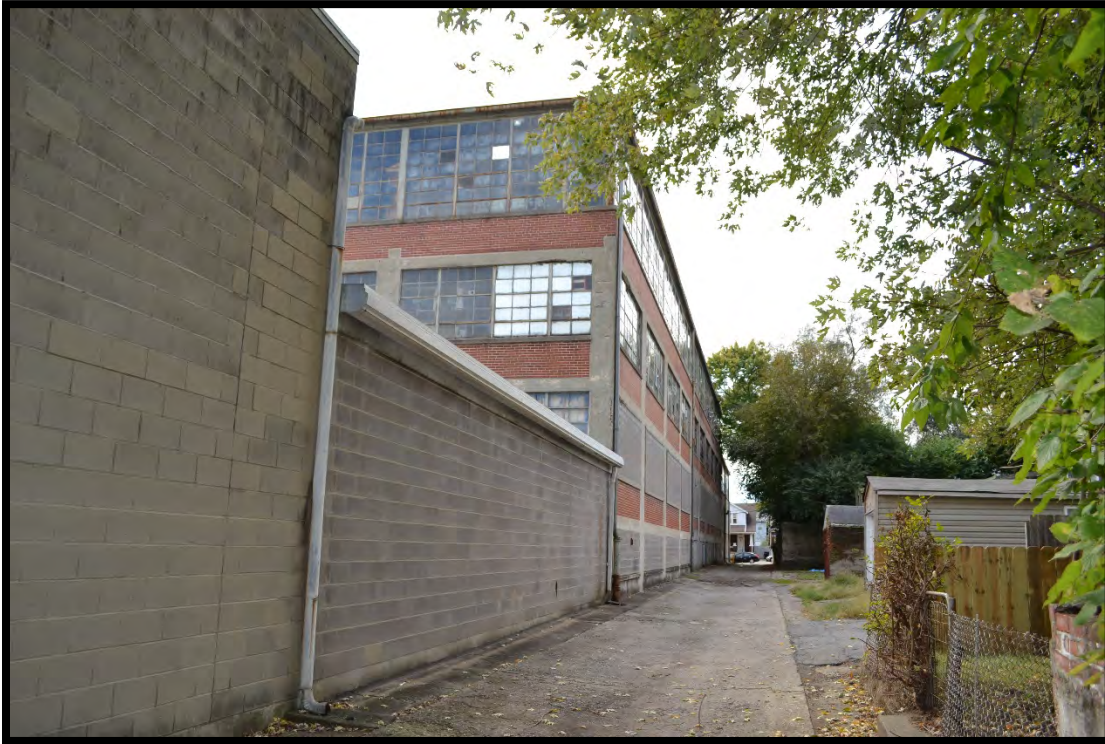
Figure 16. View of rear (north elevation) of 1925/1946 addition and the circa 1980 Kent Co. Building, looking SW. (Photo 0008).
