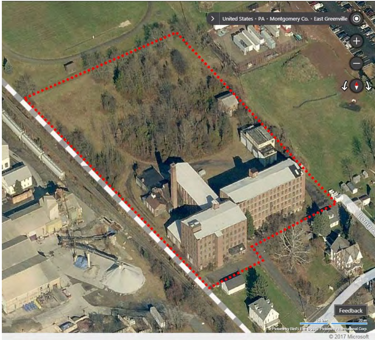
Figure 1 – Bird’s Eye aerial photograph w/ NR boundary, south view. https://www.bing.com/maps . Accessed on August 28, 2017.
