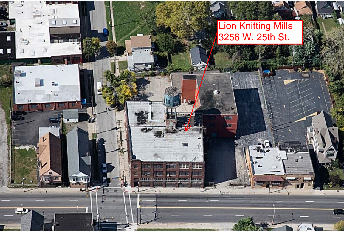
Aerial view from East - West 25th Street & Meyer Avenue
