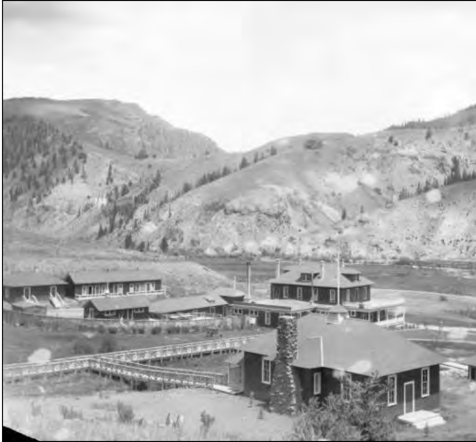
H3. Undated photograph looking northeast. Shows the Palmer House (constructed in 1905) in the foreground and the Laundry and Bird's Nest buildings in the background at the left. The Ice House and the building that would be part of the Owner's Cabin/Powder Mag is also visible. The Lodge in the center-right of the photo was replaced in 1948. Denver Public Library/History Colorado Photo CHS.X5212.
