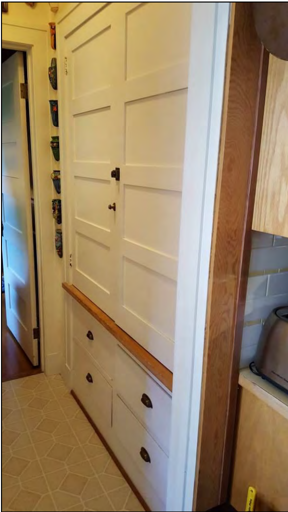
18 of 26 WA_Spokane County_Warner House_0018.tiff An original 1916 linen closet located in the service hall by the kitchen, looking south in 2019
