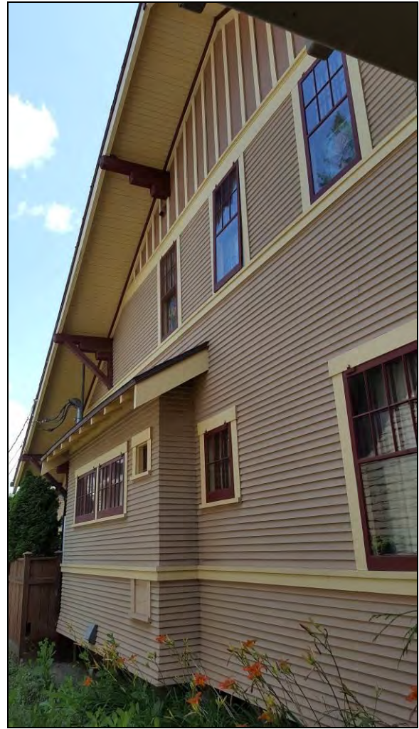
5 of 26 WA_Spokane County_Warner House_0005.tiff North face of Warner House in 2019
