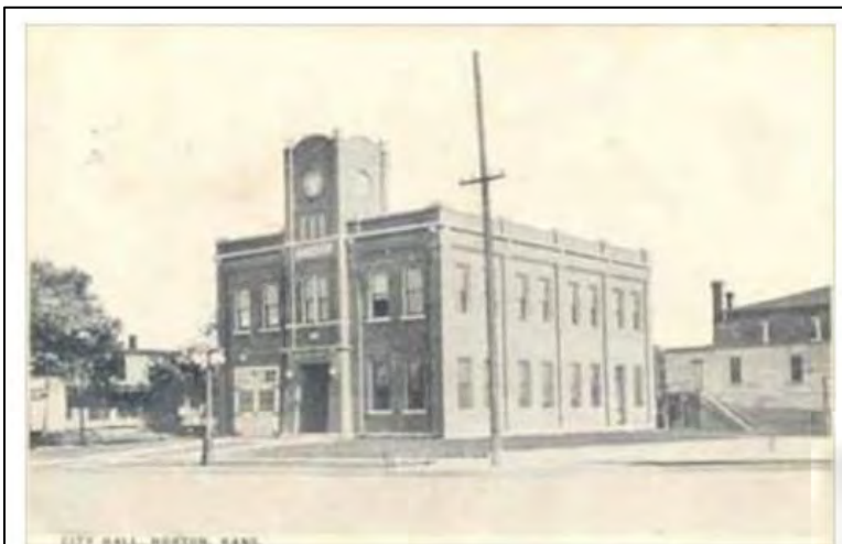
Figure 6: Horton City Hall, photo taken after its opening
