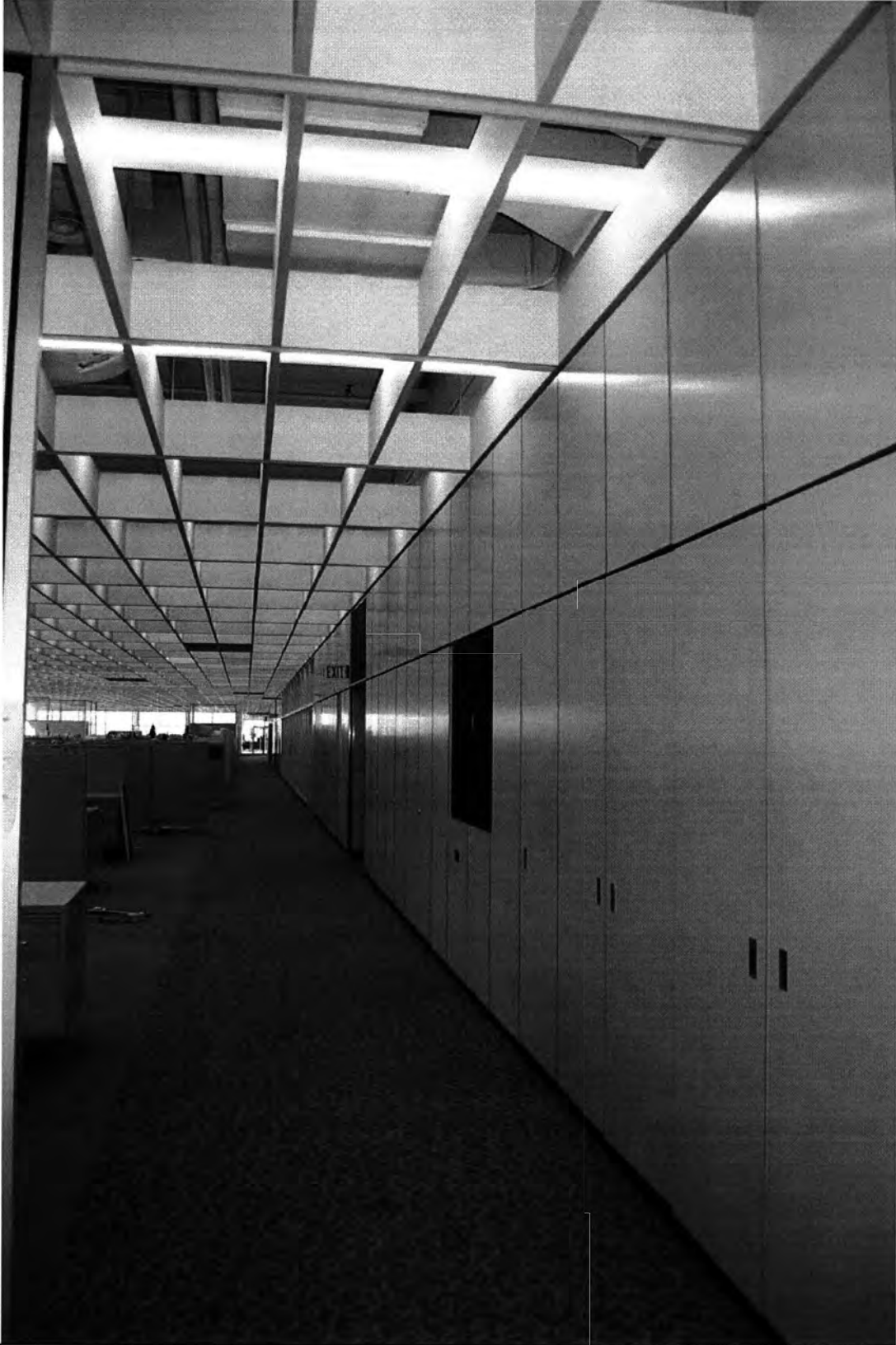
19. Third floor northwest quadrant, view looking south along utility cores
