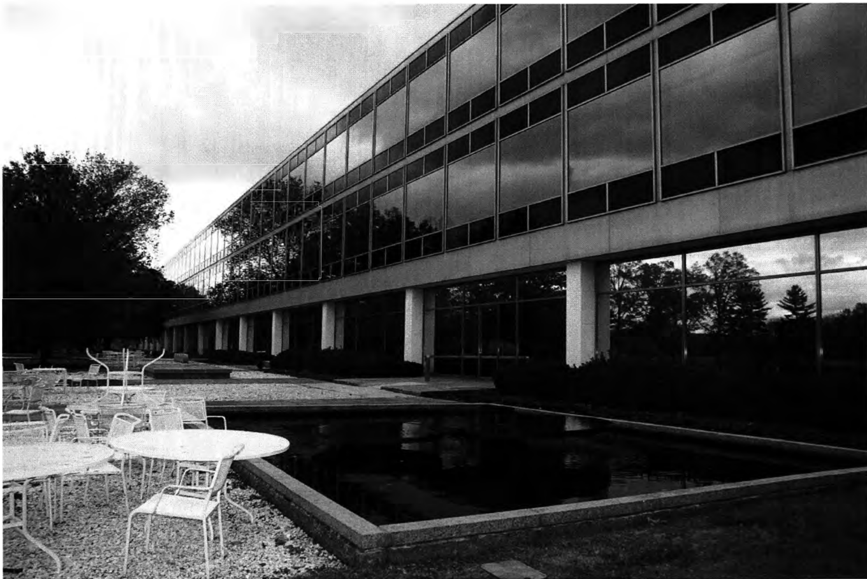
26. South terrace showing south elevation and water feature at right, view northwest
