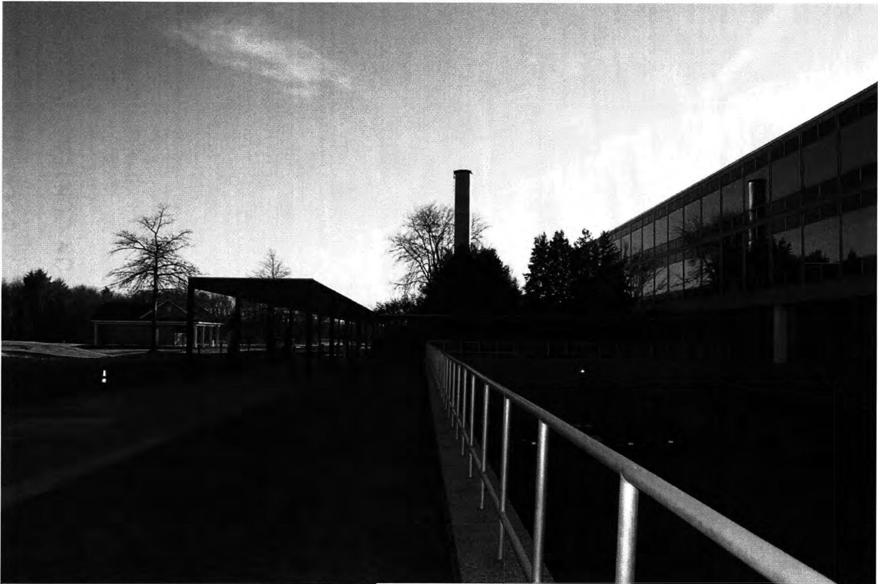
6. View looking south toward loading dock
