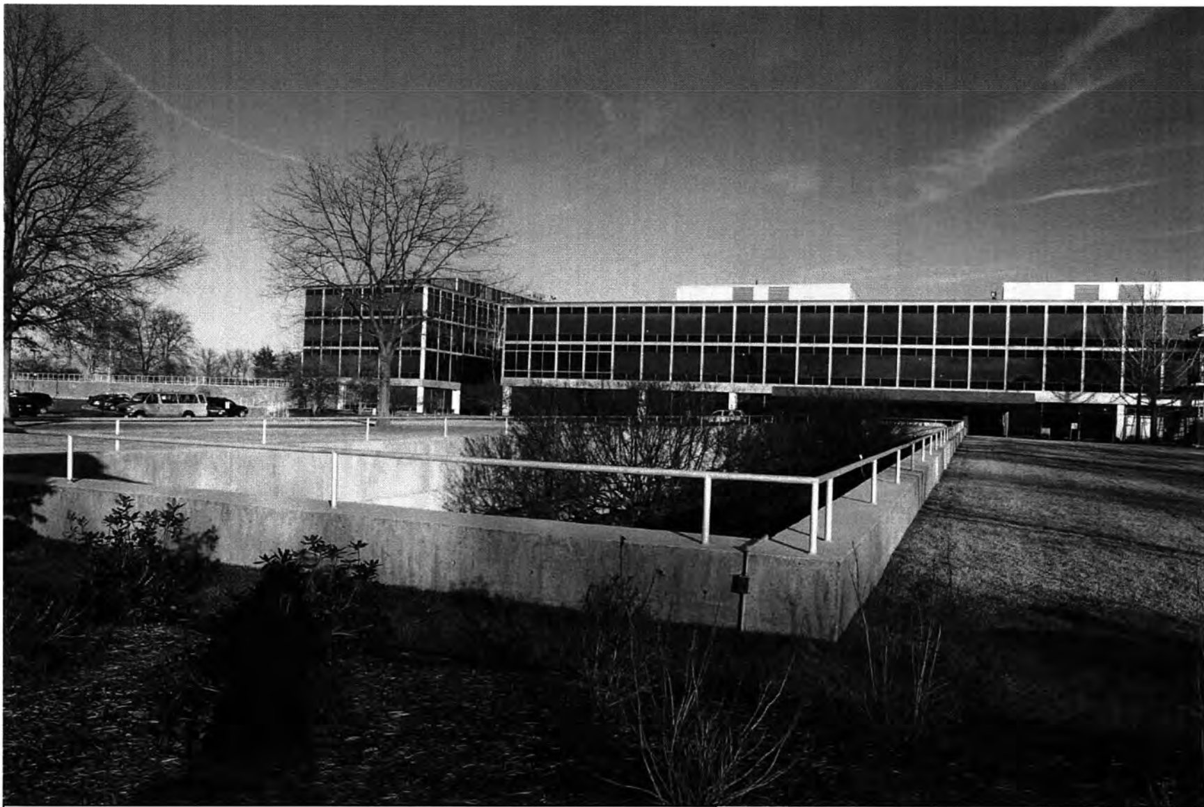
9. West elevation, view looking northeast across pedestrian walkway
