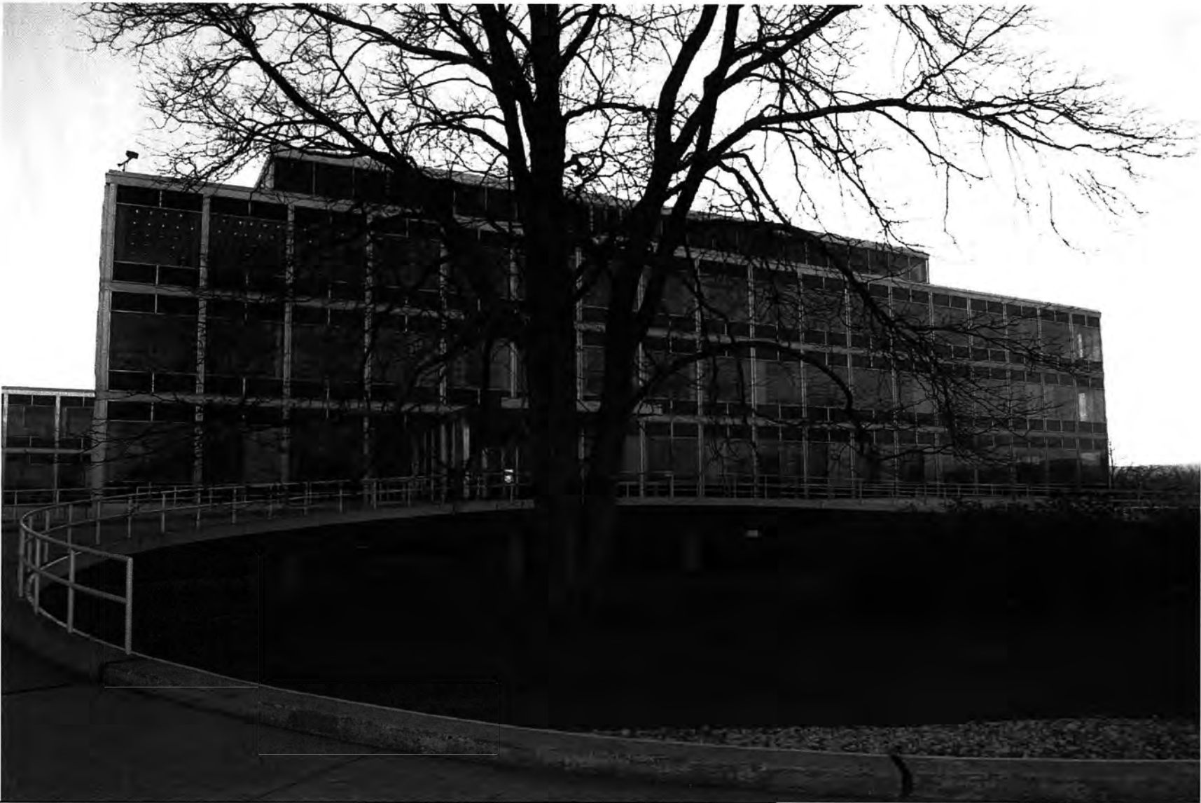
7. North elevation of North Wing and main building, view looking southwest
