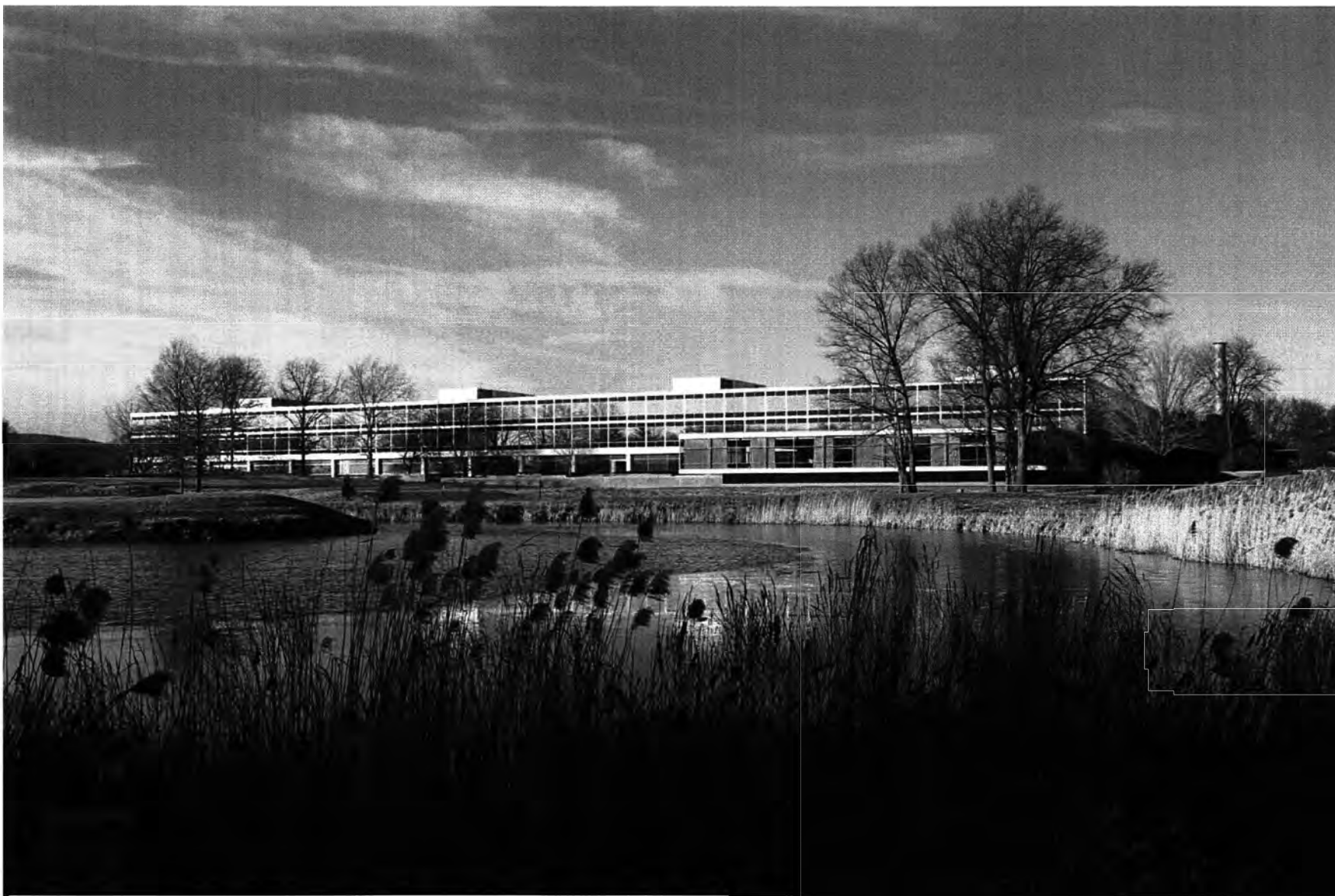
1. South elevation, view looking north from golf course; remaining portion of cooling feature (pond) in foreground
