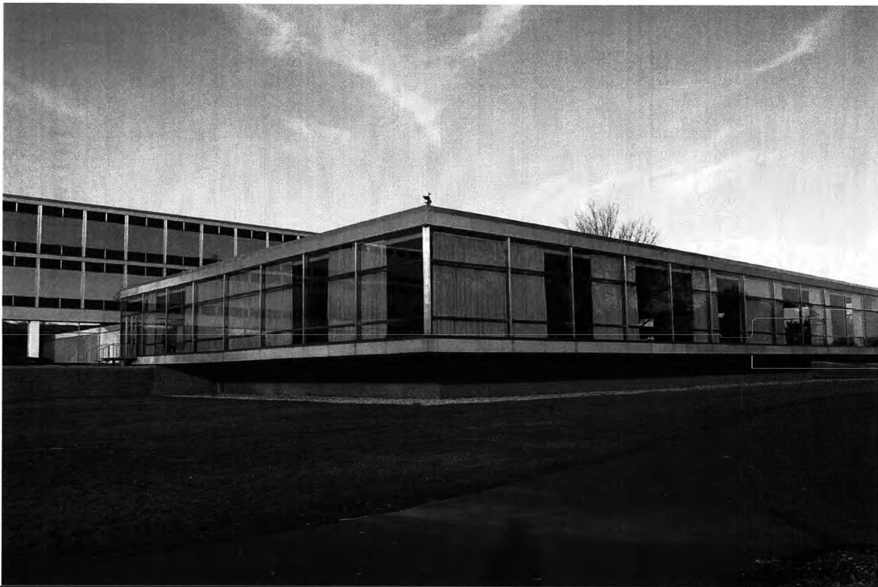
2. West and south elevations of cafeteria, view looking northeast
