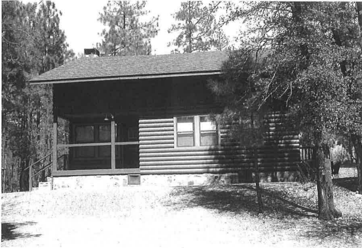
Photo to East: 8/31/2012
