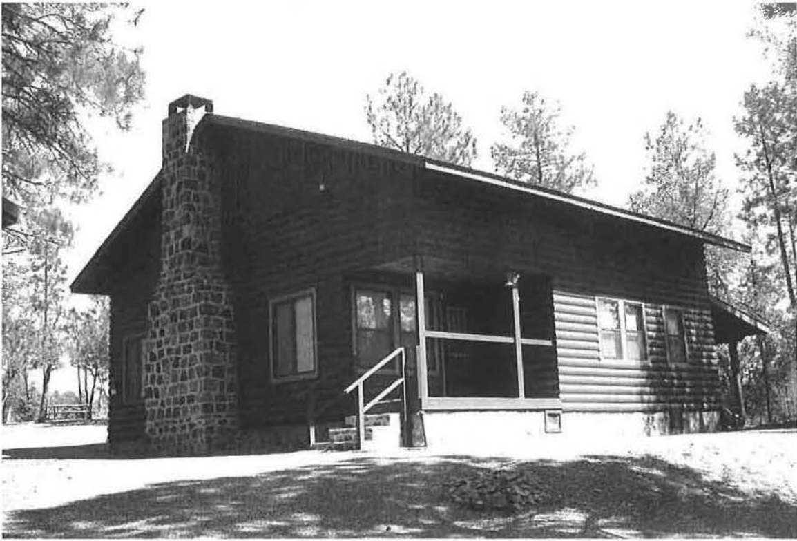
Photo to Southeast: 8/31/2012
