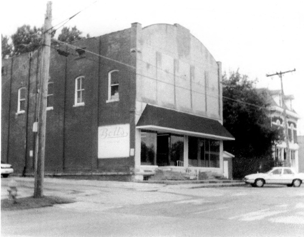
Building at time of sale/purchase in 1997 (Miller files)
