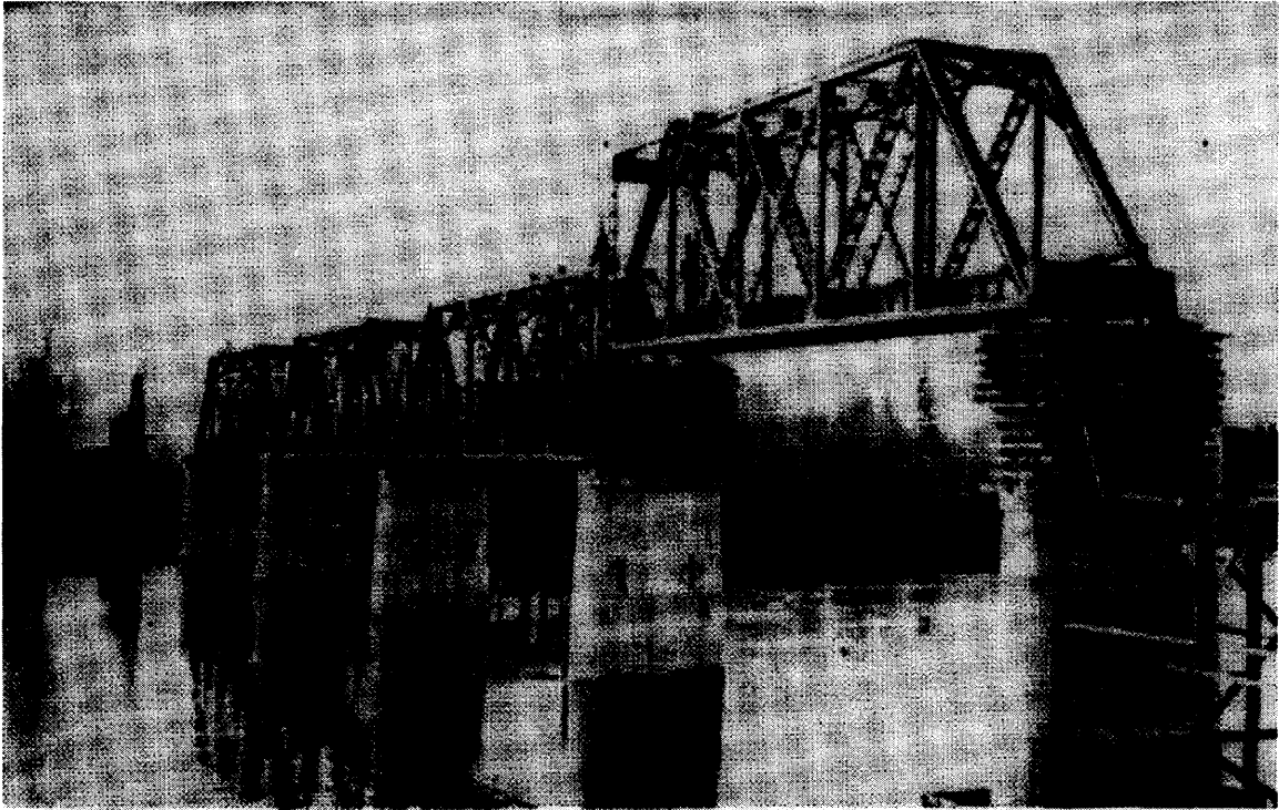
Railroad bridge spanning the Willamette under construction in 1912
