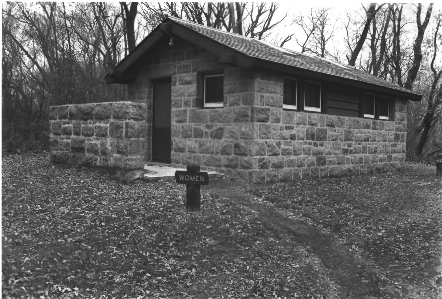
FORT RIDGELY STATE PARK NICOLLET CO. MN BLDG # 10 PHOTO I.D. 09113 # 10
