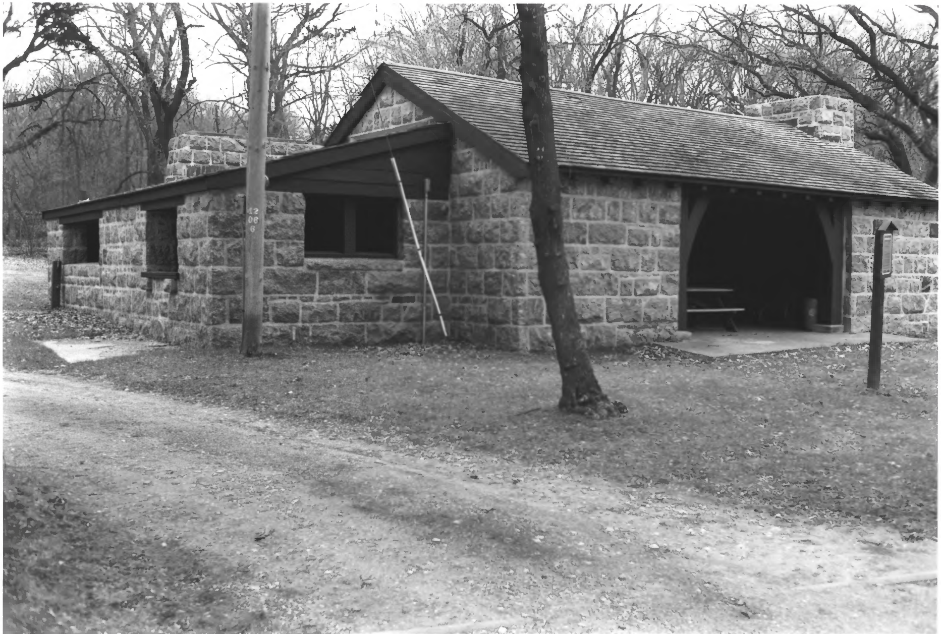
FORT RIDGELY STATE PARK NICOLLET CO. MN BLDG # 1, PHOTO I.D. 09114 #9
