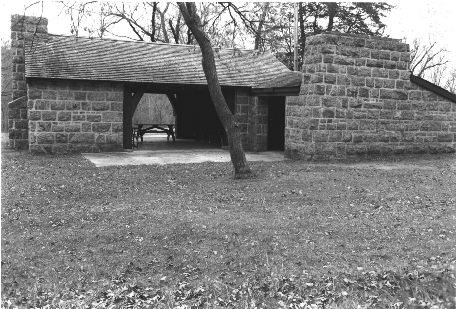
FORT RIDGELY STATE PARK NICOLLET CO., MN BLDG #1 PHOTO I.D. 19114 #8
