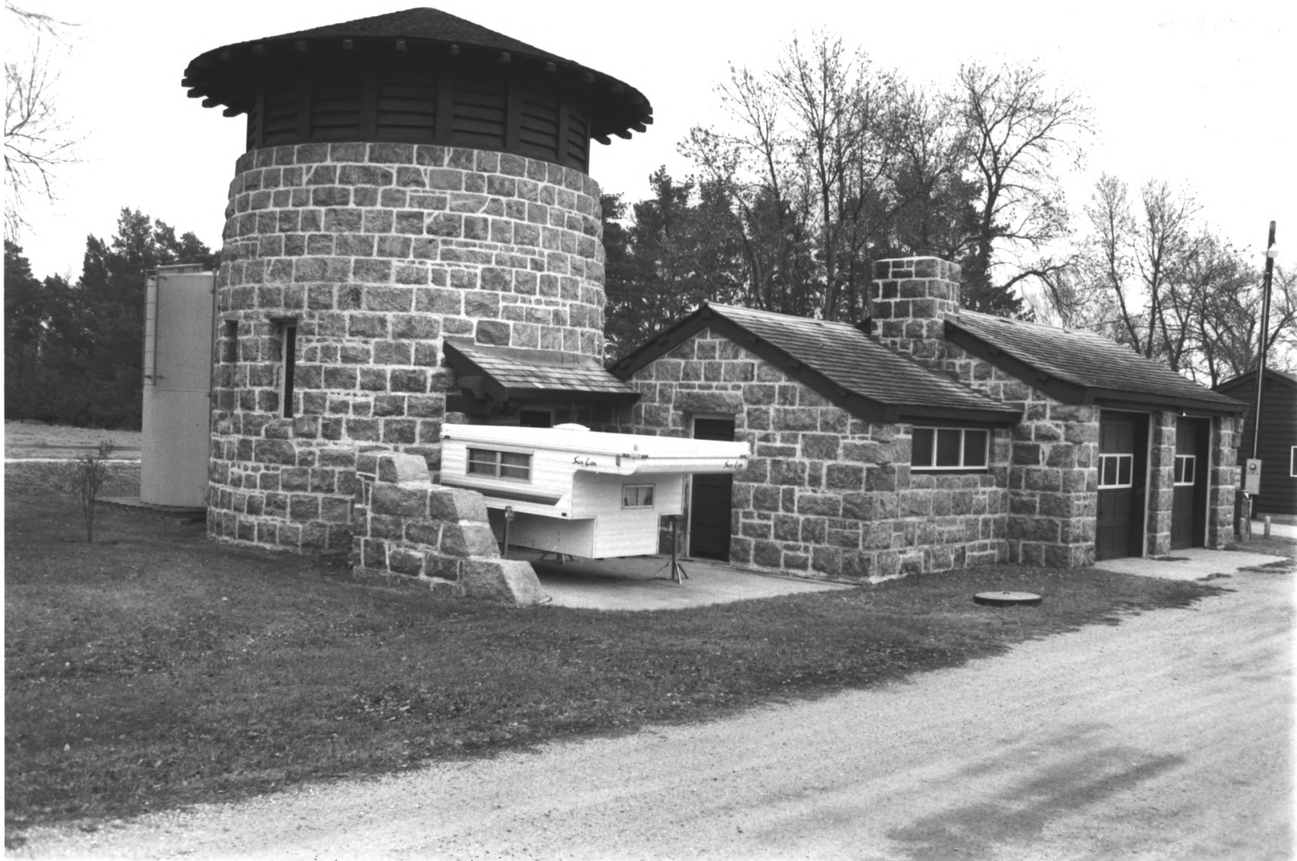
FORT RIDGELY STATE PARK NICOLLET CO., MN BLDG #18 PHOTO I.D. 09113 #15
