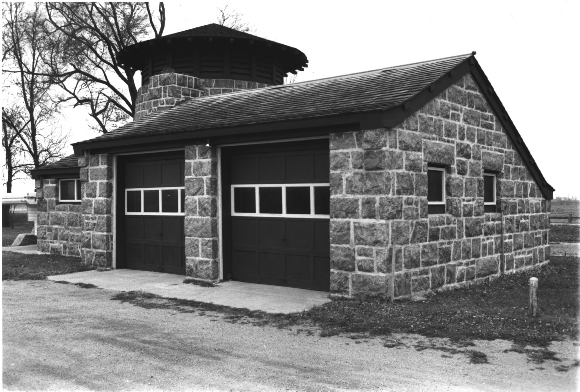
FORT RIDGELY STATE PARK NICOLLET CO., MN BLDG # 18 PHOTO I.D. 09113 # 14
