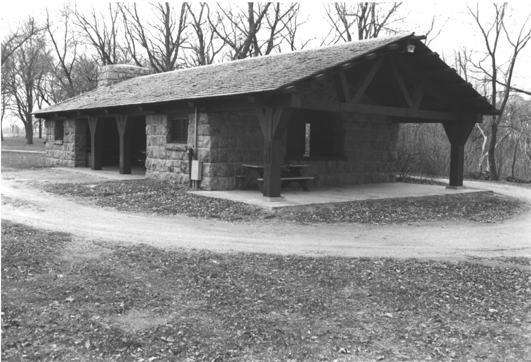
FORT RIDGELY STATE PARK NICOLLET CO., MN BLDG # 9 PHOTO I.D. 09113 # 7
