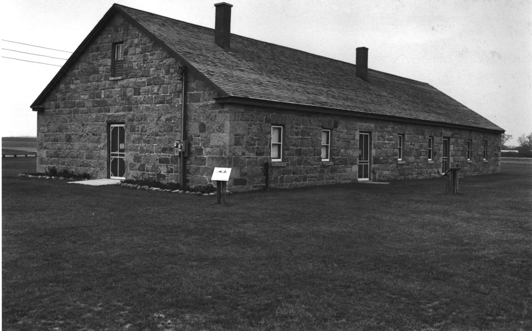
FORT RIDGELY STATE PARK NICOLLET CO. MN BLDG# 13 PHOTO I.D. 09113#20
