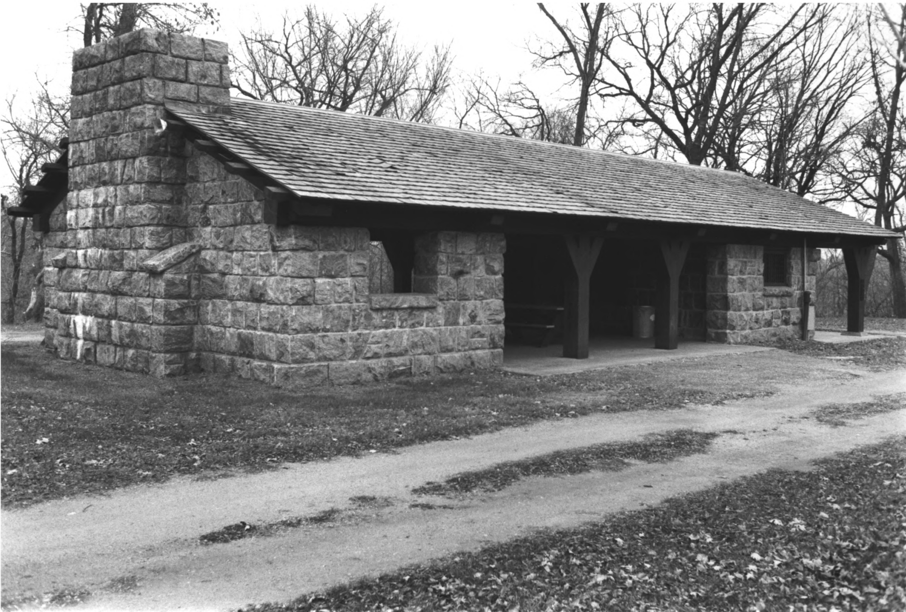
FORT RIDGELY STATE PARK NICOLLET CO. MN BLDG # 9 PHOTO I.D. 09113#8
