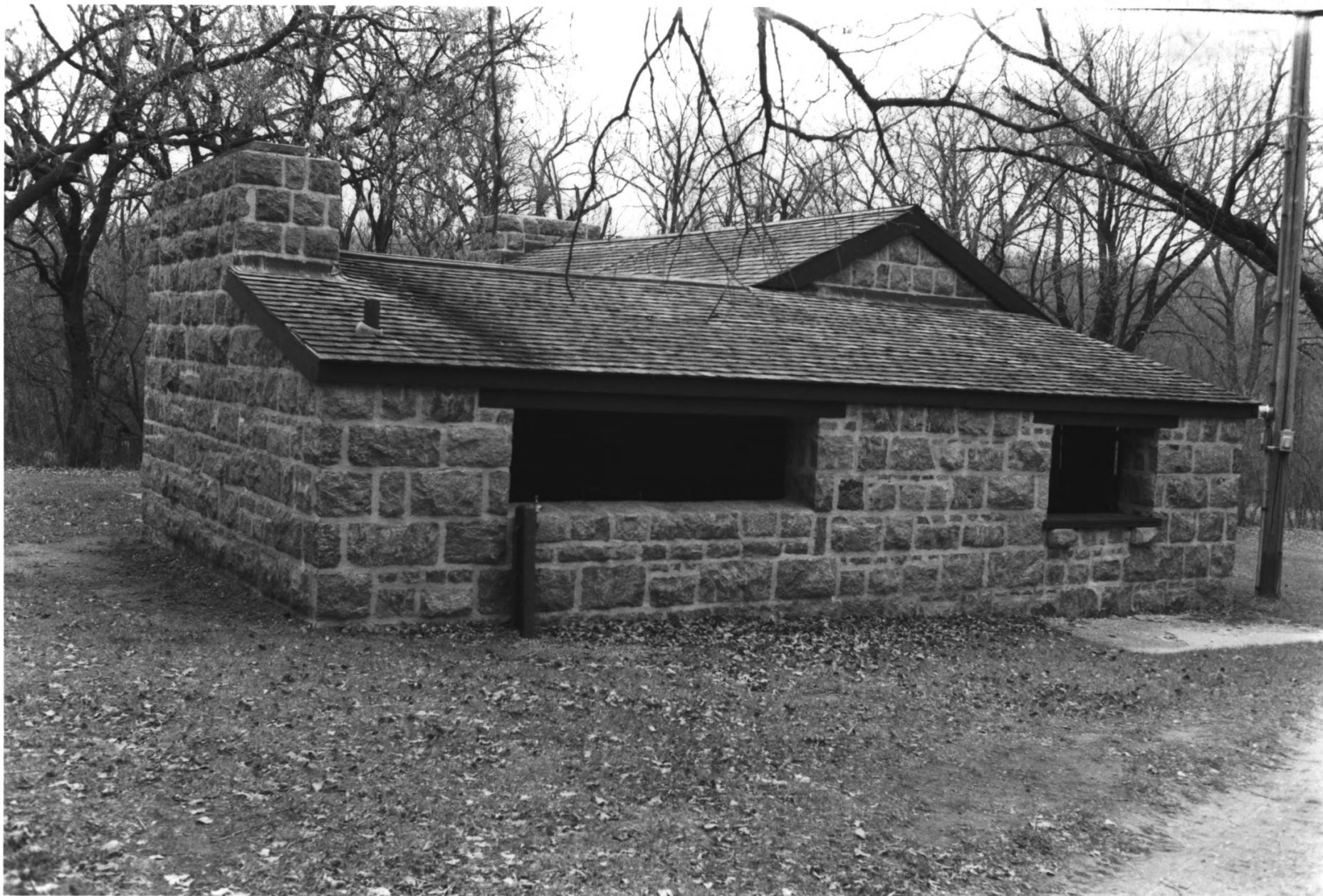
FORT RIDGELY STATE PARK NICOLLET CO., MN BLDG #1, PHOTO I.D. 09114 #10
