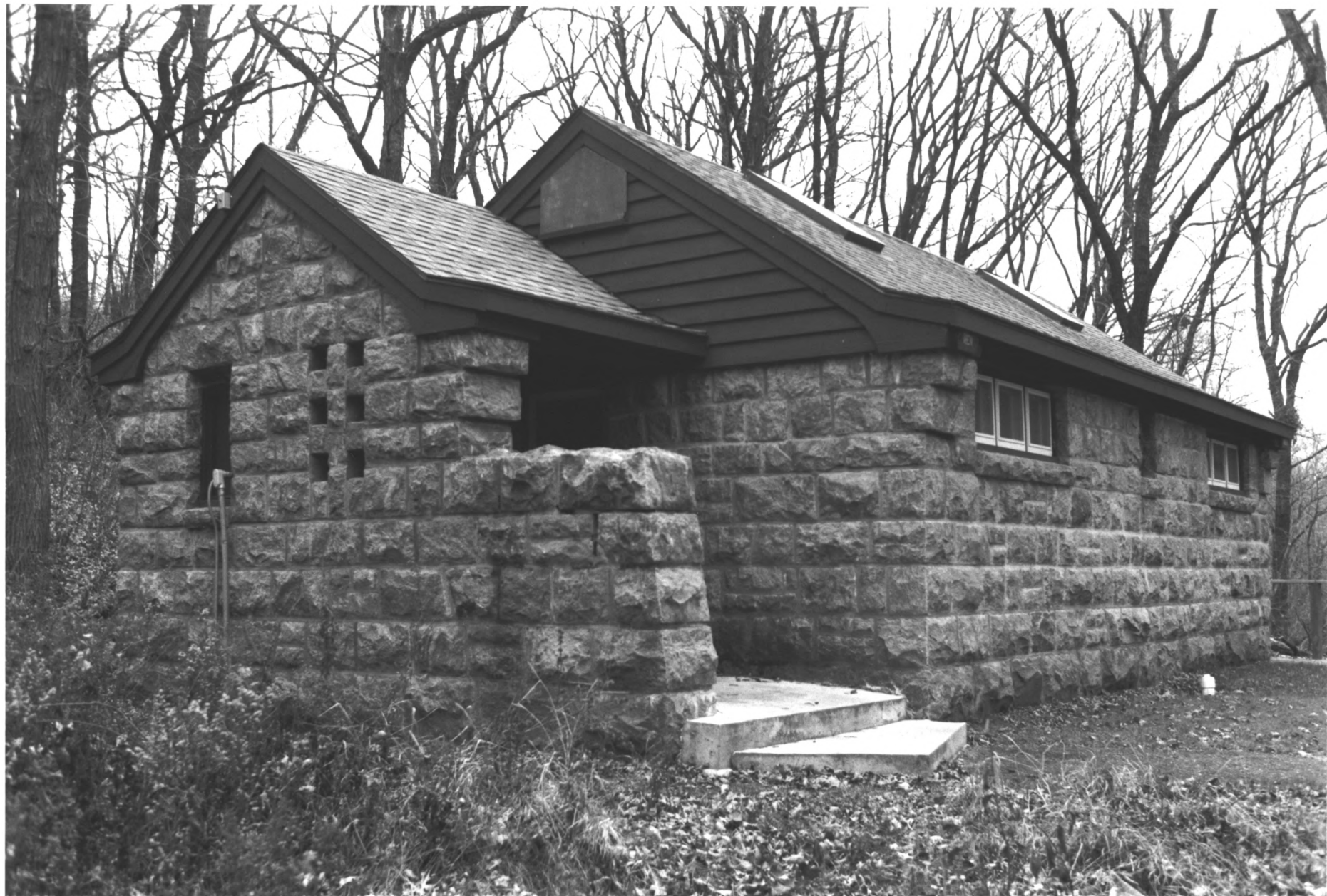
FORT RIDGELY STATE PARK NICOLLET CO., MN BLDG # 7 PHOTO I.D. 09114 #16
