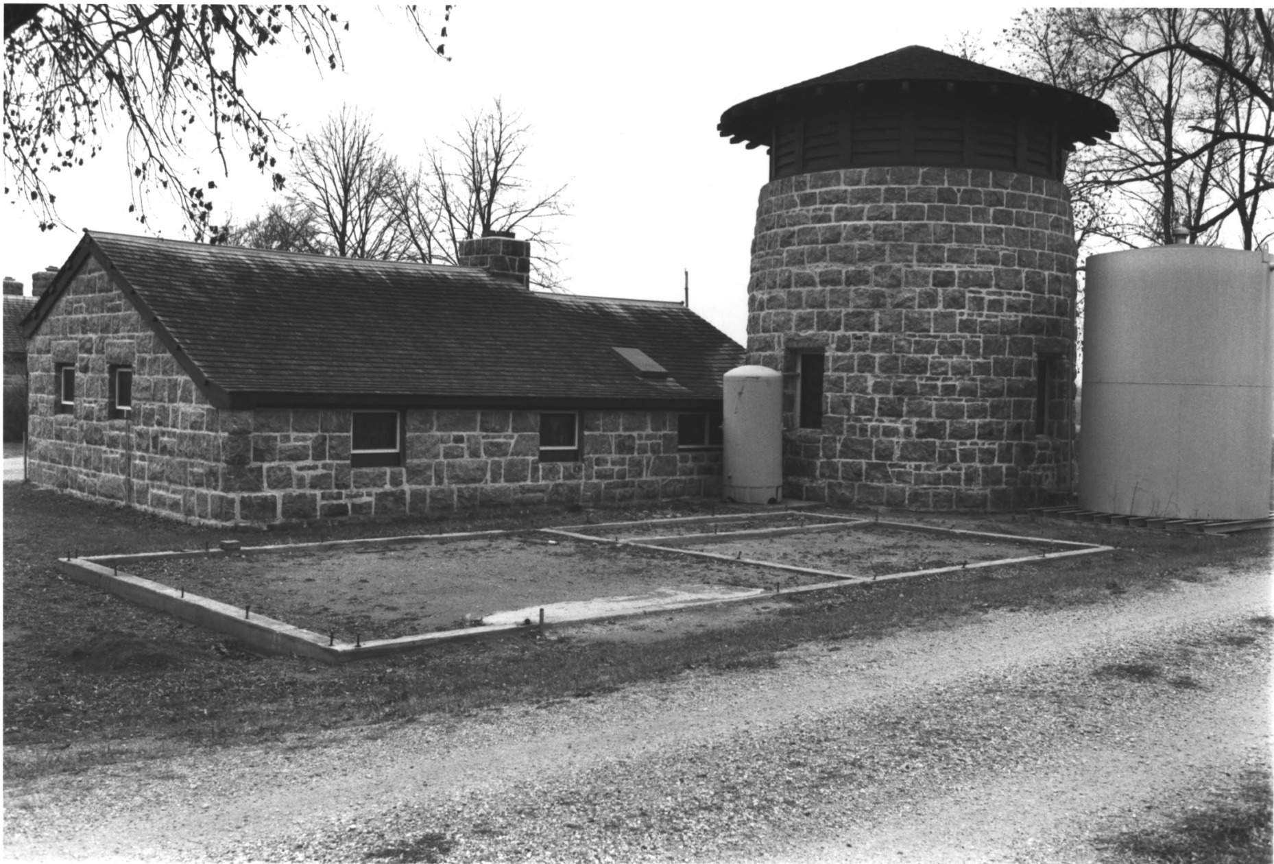
FORT RIDGELY STATE PARK NICOLLET CO. MN BLDG # 18 PHOTO I.D. 09113 # 16
