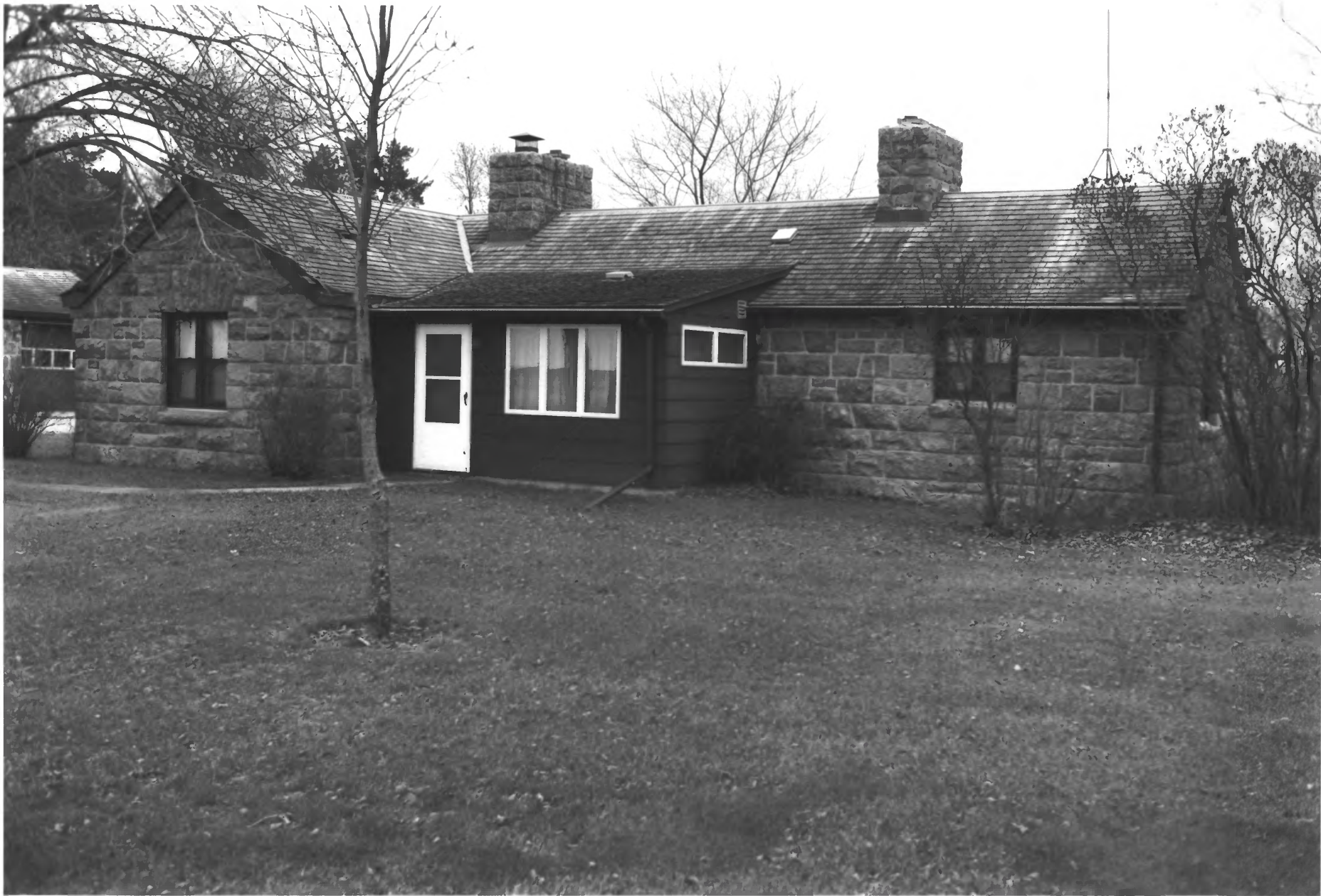
FORT RIDGELY STATE PARK NICOLLET CO., MN BLDG # 17 PHOTO I.D. 09113 #12
