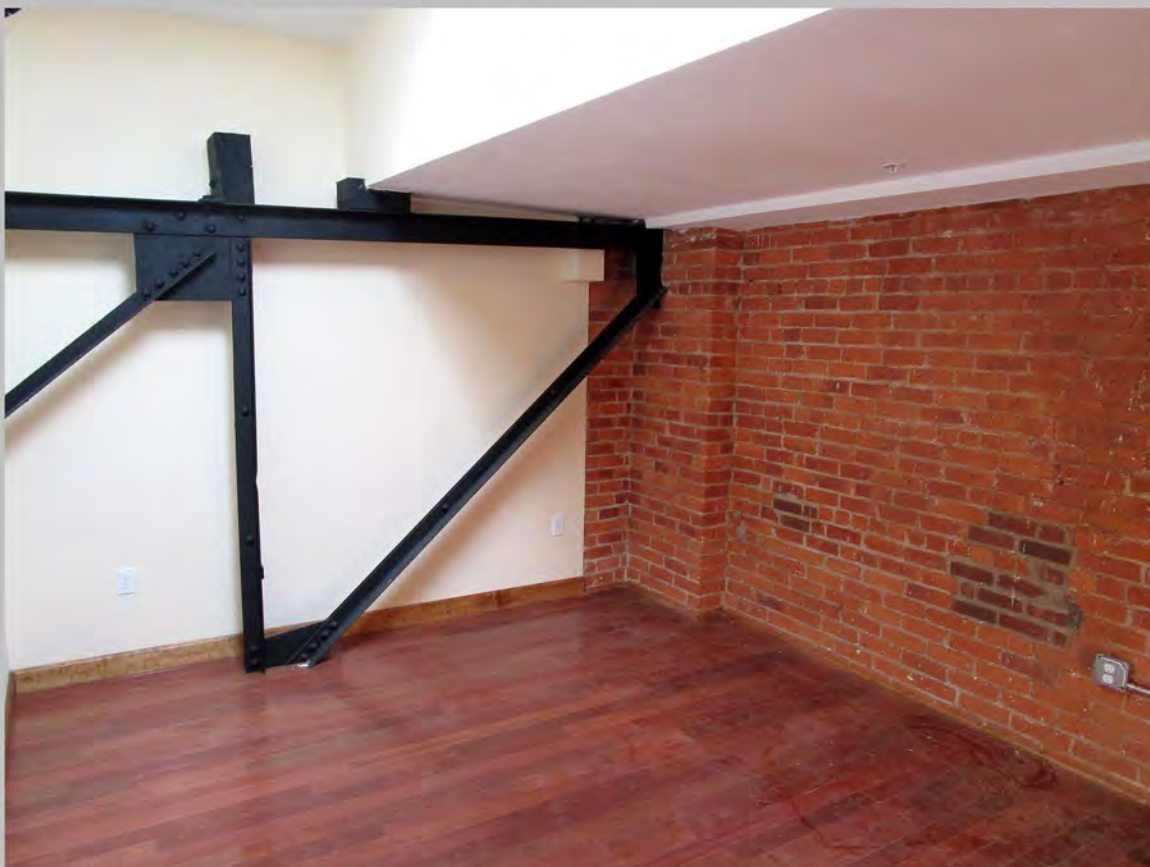
6. Interior, detail of truss and brick wall
