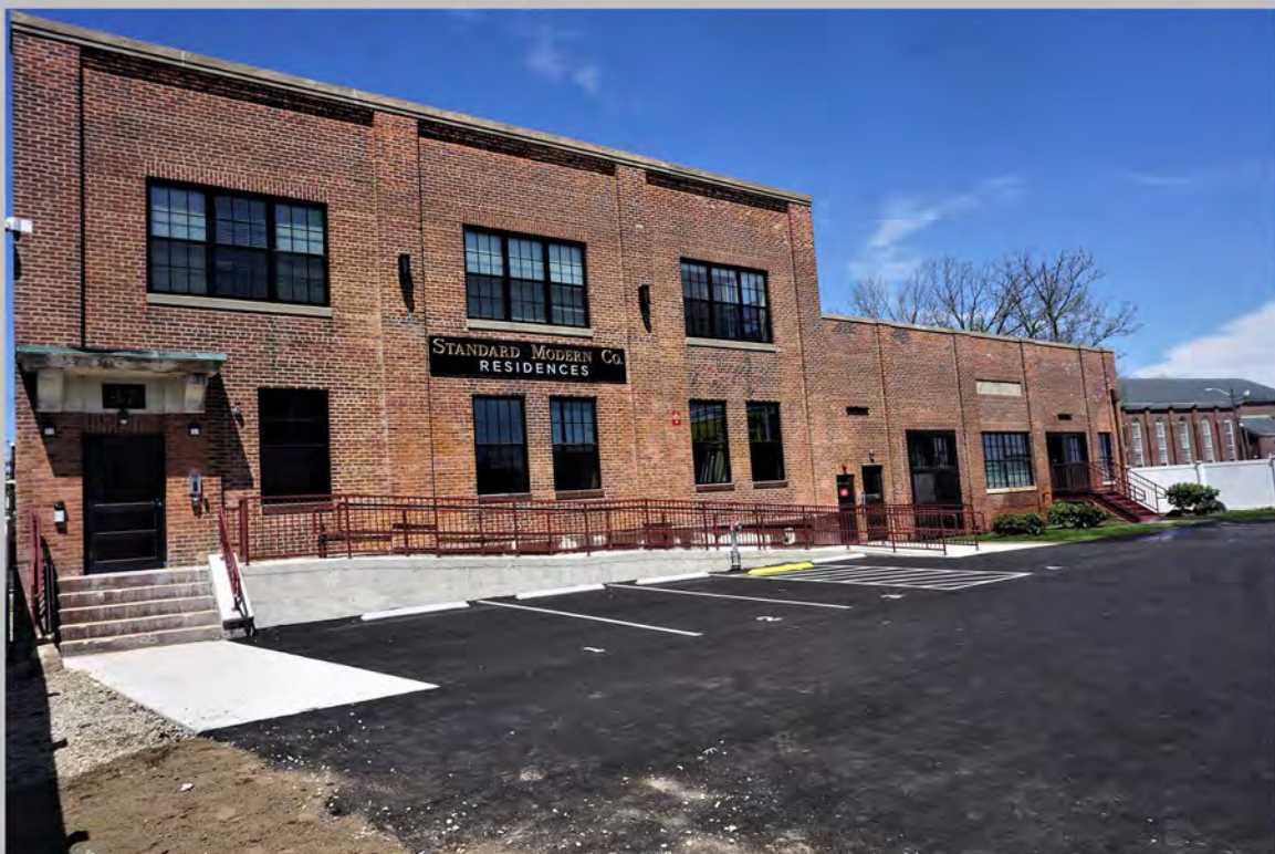
2. View northeast of south and west elevations
