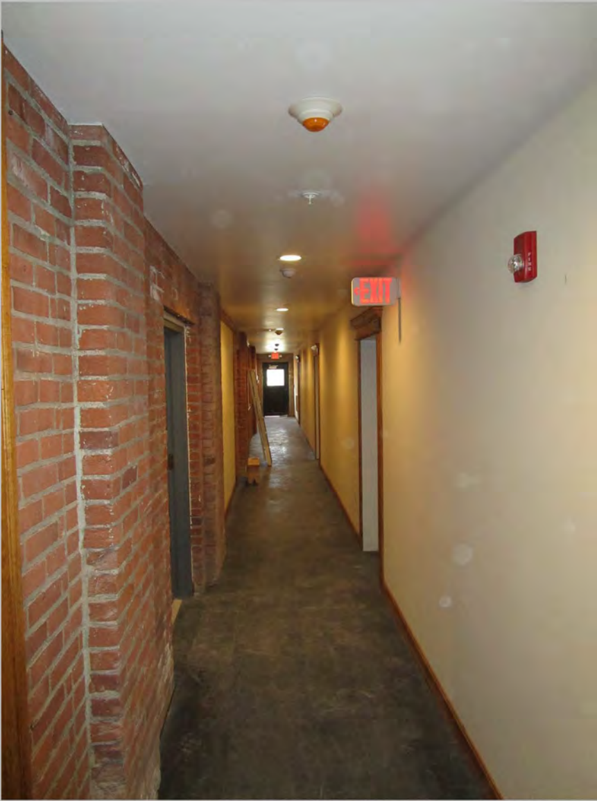
7. Interior, view west of corridor showing exposed brick and concrete
