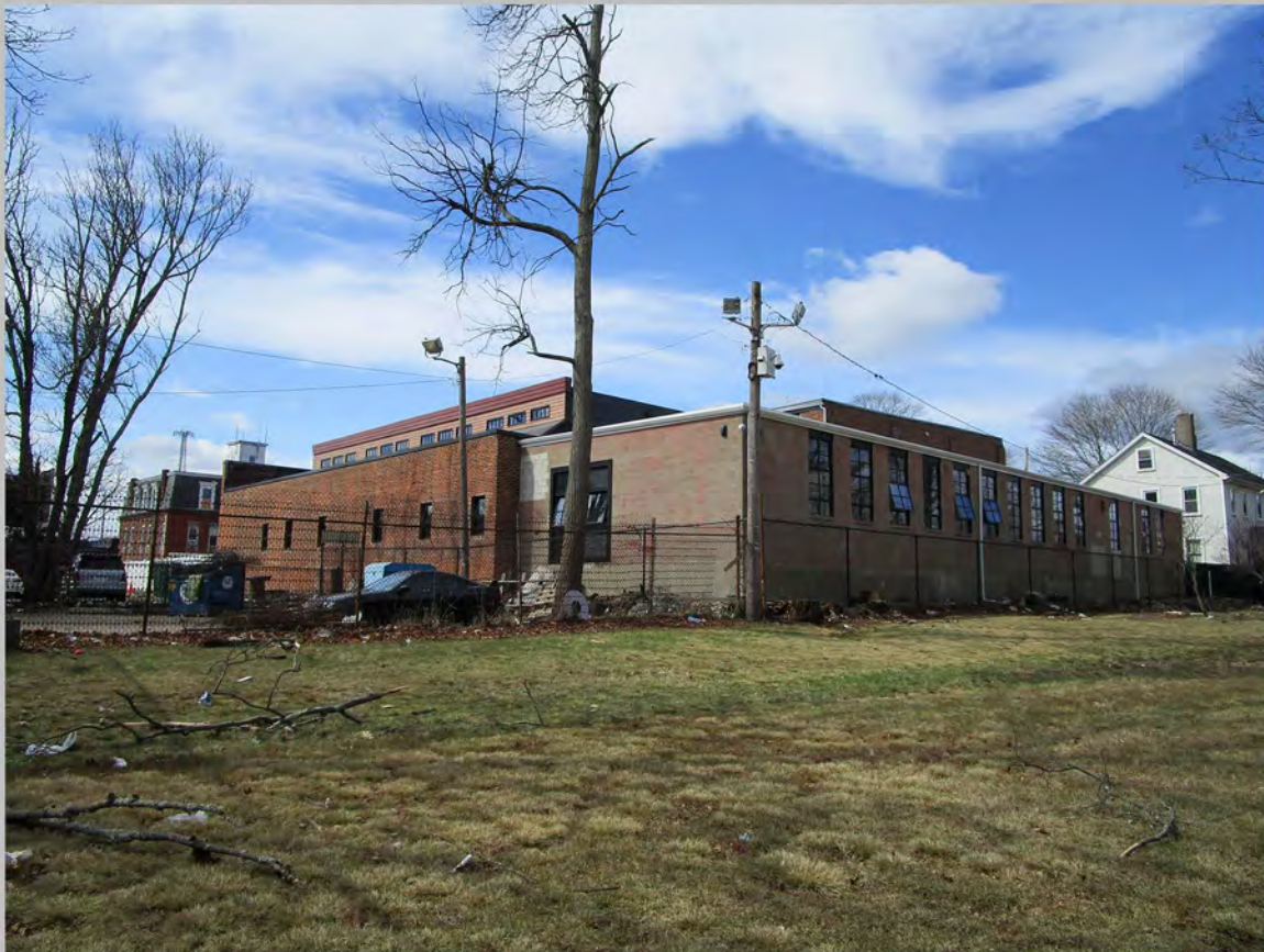
5. View southwest of north and east elevations
