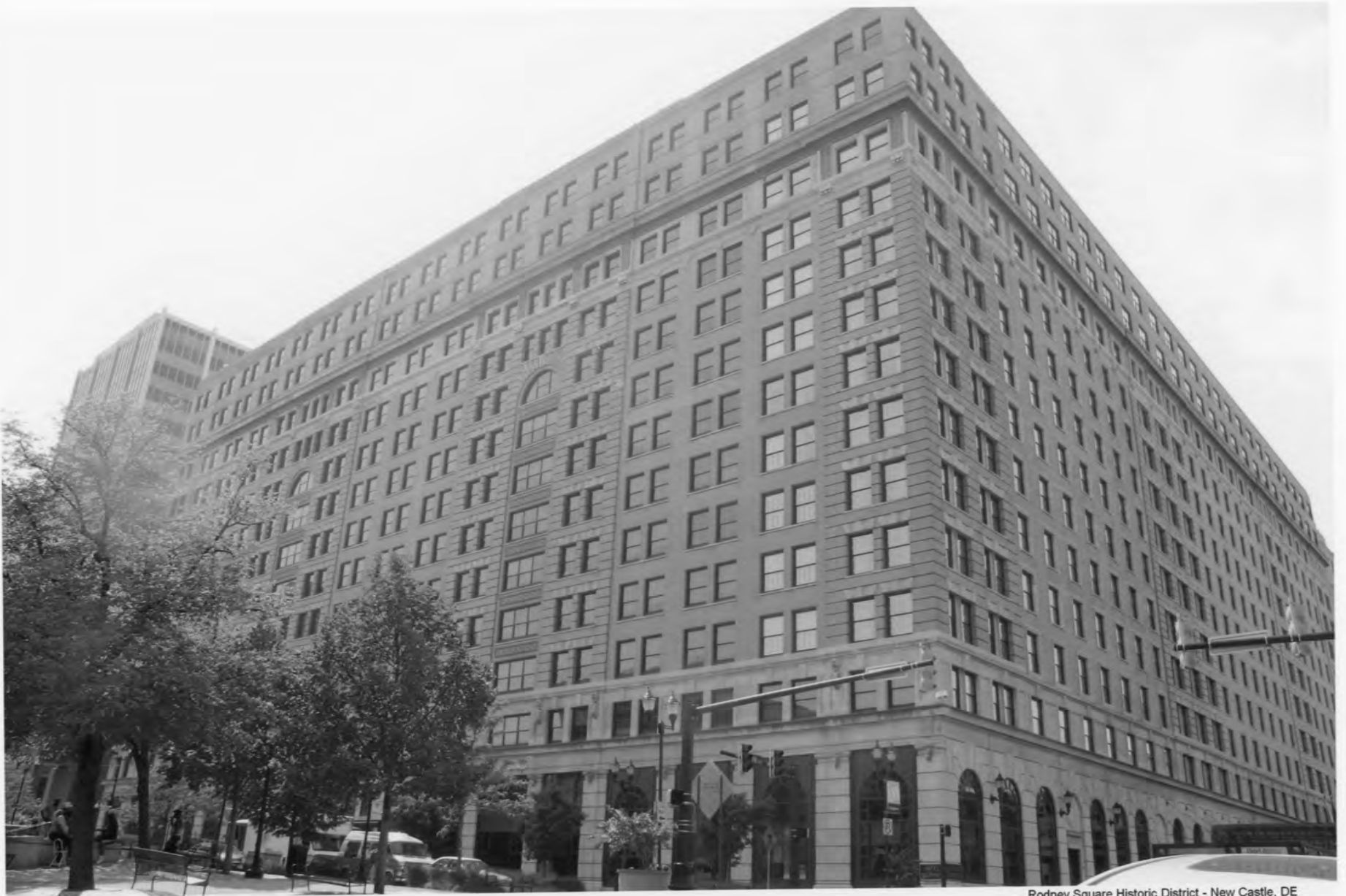
Rodney Square Historic District - New Castle, DE DuPont Building, North and East elevations, view southwest 20 of 28
