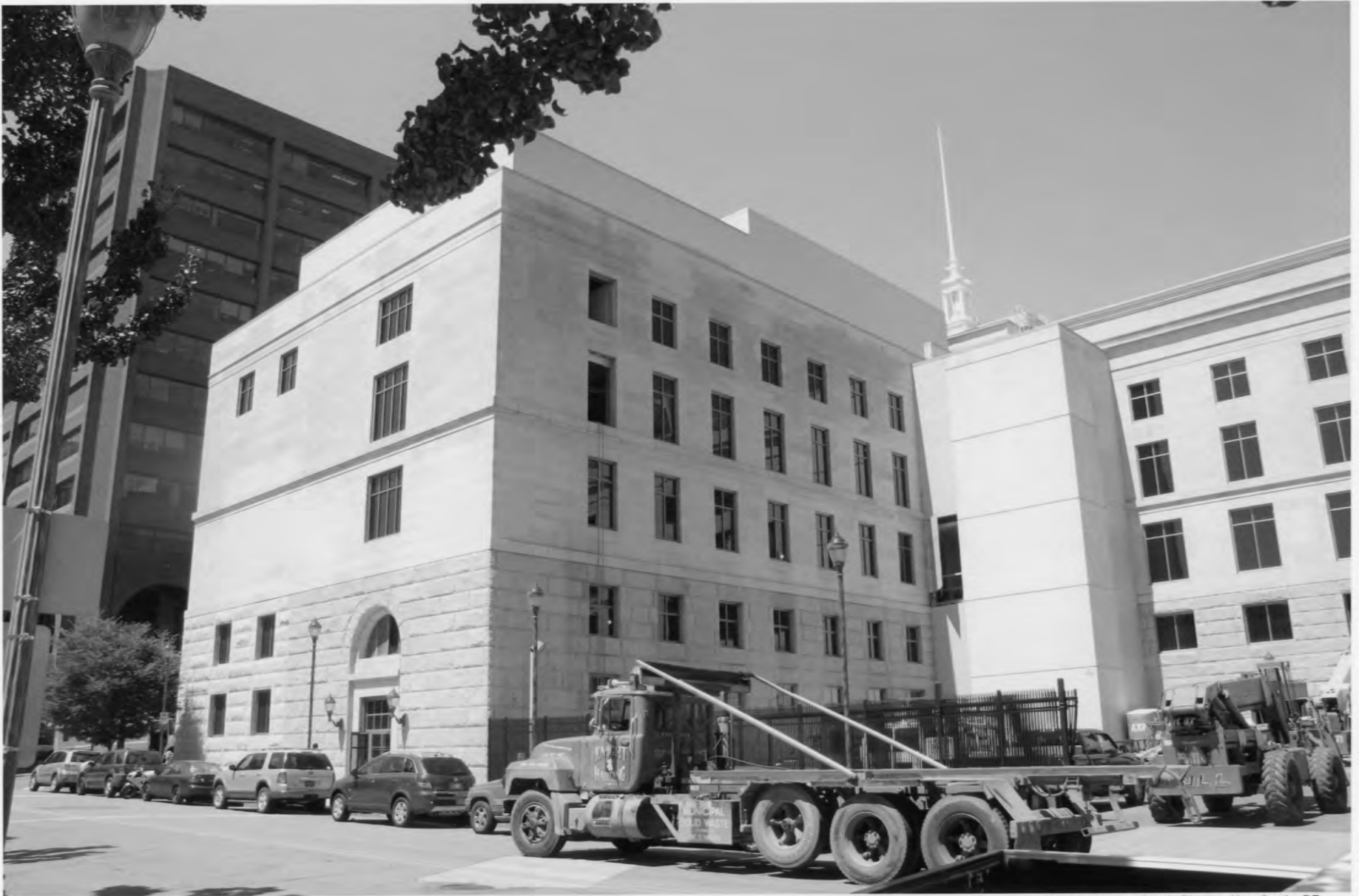
Rodney Square Historic District - New Castle, DE Wilmington Public Building, East elevation view southwest
