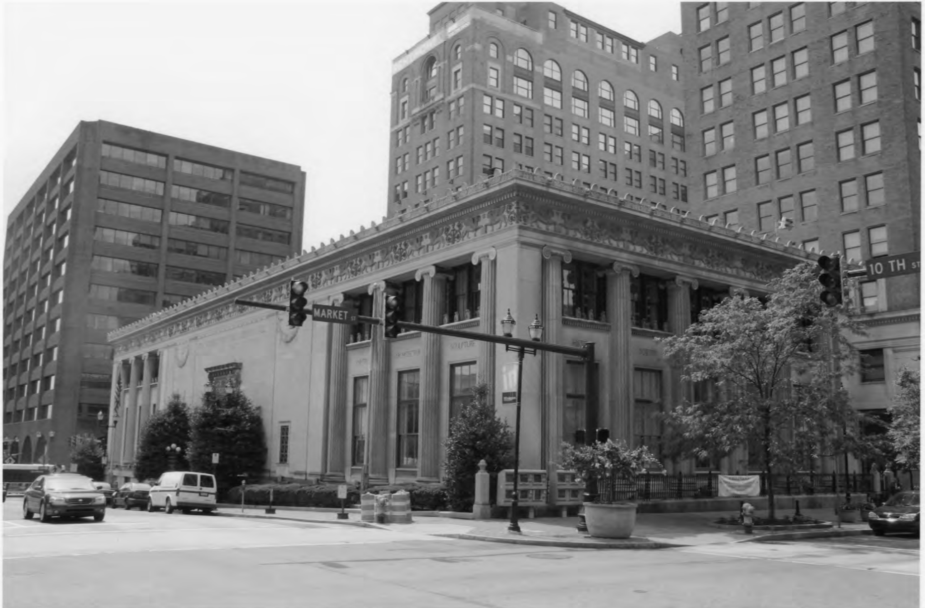
Rodney Square Historic District - New Castle, DE Wilmington Institute Free Library, North and West elevations, view southeast 12 of 28
