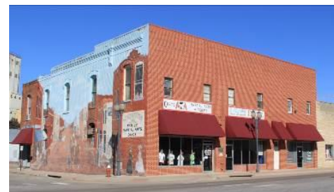
Figure 1: Alterations made to front elevation at 135-140 W. 13th (SA01-375). APMA, 2015.
