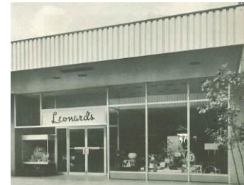
Figure 6: Example of a 1960s aluminum storefront. Kawneer Architectural Products, 1960 Catalog, Building Technology Heritage Library, archive.org.
