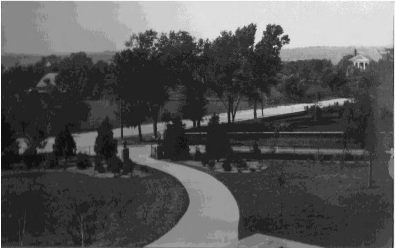
Figure 25 – The house at 6300 Dodge overlooked the intersection of Dodge Street and Fairacres Road. The driveway is seen in the foreground. Photo taken prior to the paving of Fairacres Road in 1915. (Courtesy of James and Elizabeth Quinn).
