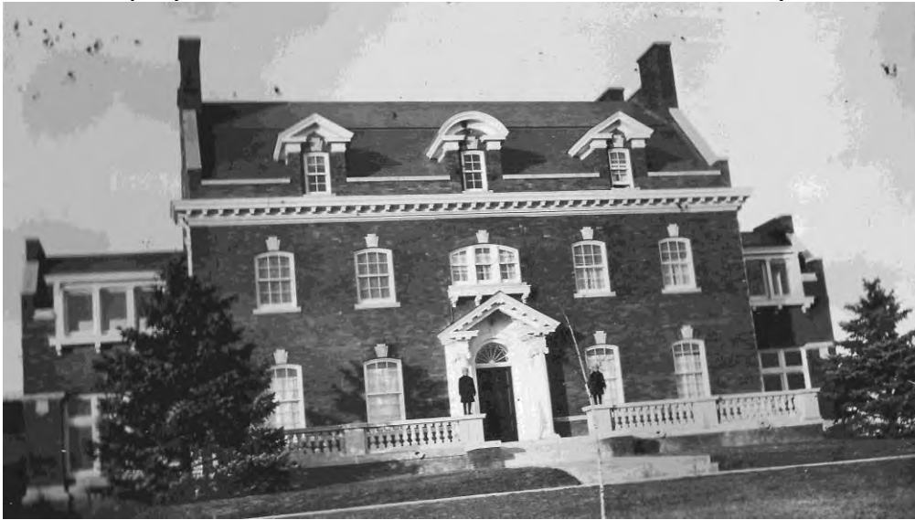
Figure 30 – The house at 6300 Dodge Street was designed by Frederick A. Henninger. Photo taken in 1912, prior to the addition of a two-story central portico in 1925. (Courtesy of James and Elizabeth Quinn).
