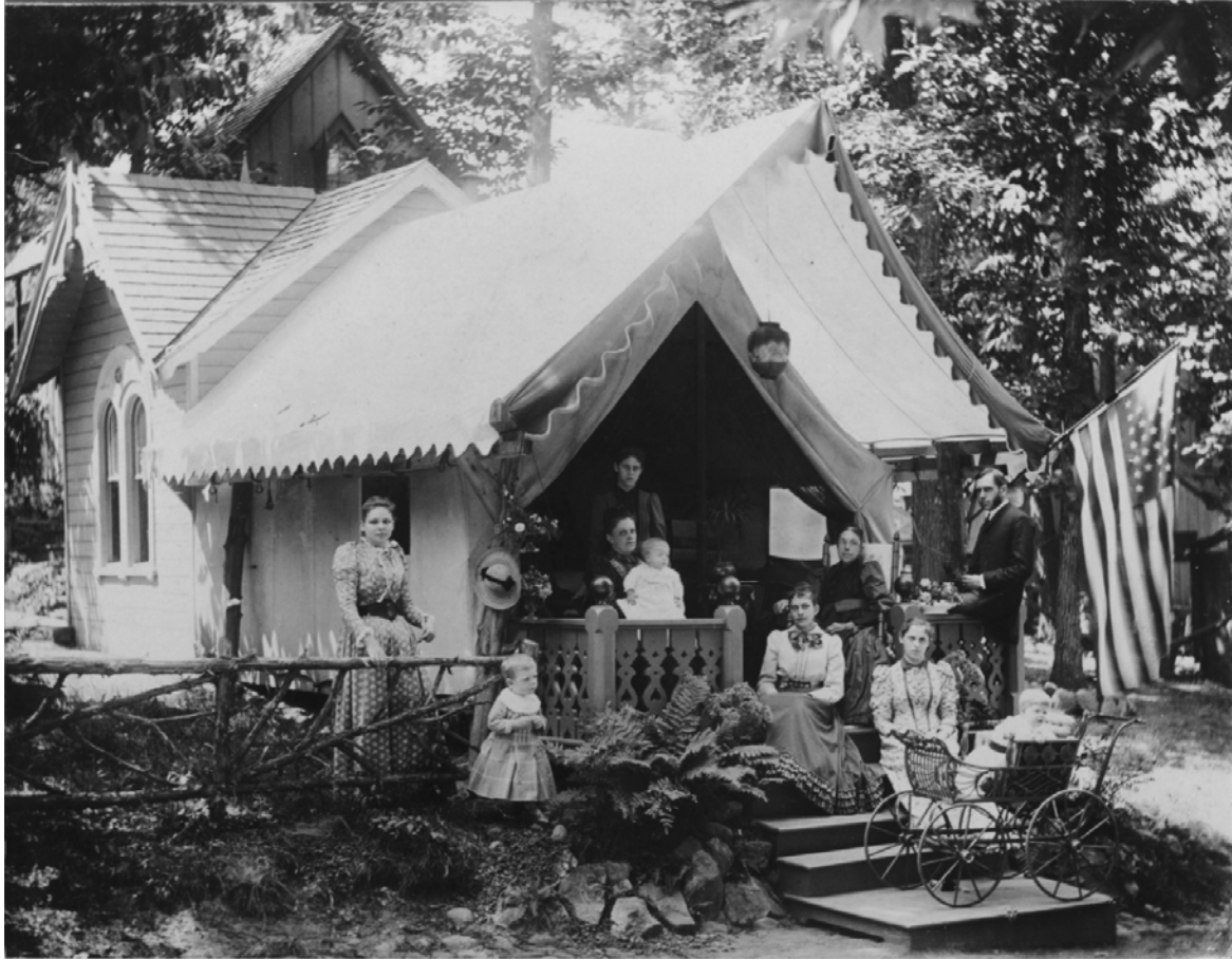
Figure 19: The Coit Family tent shows the tent-cottage combination with frame section at the rear fronted by a canvas section
