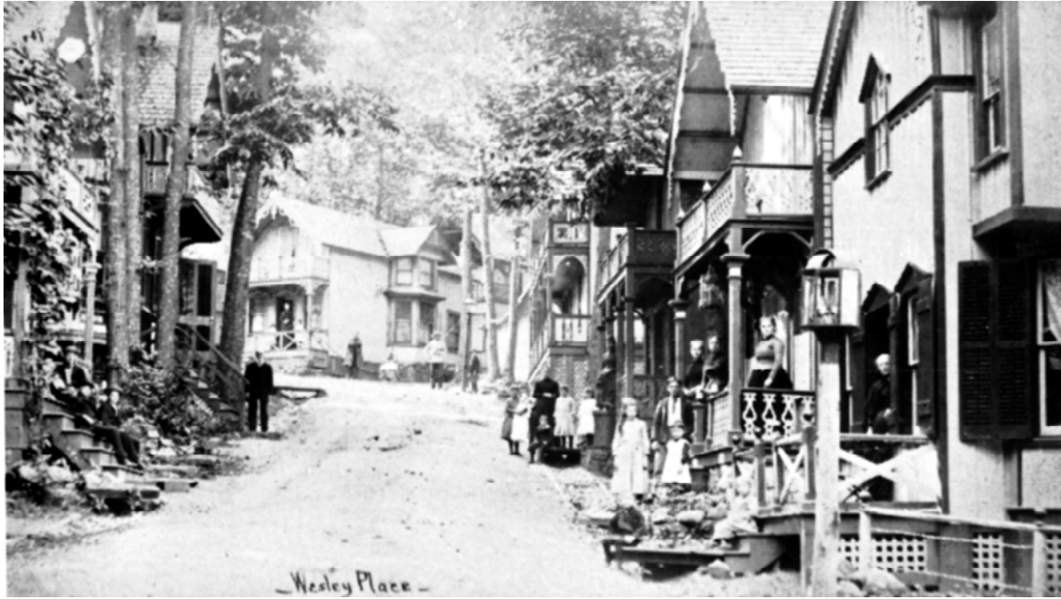
Figure 5: Undated photo of Wesley Place. Note the wooden entrance bridges that cross the side gutters.
