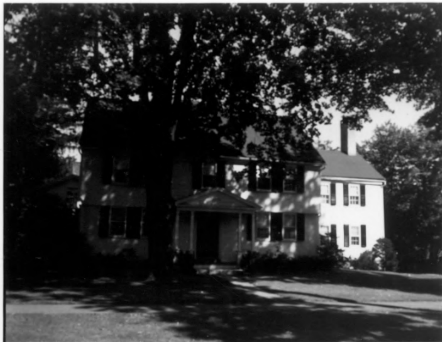
Oliver Wolcott, Sr. House, 1753 South Street
