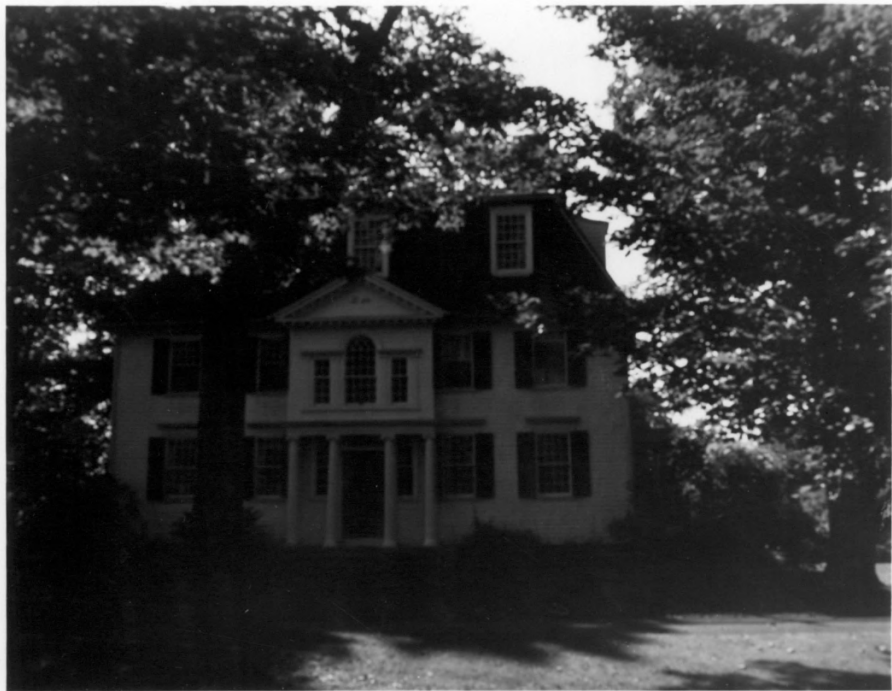
Sheldon's Tavern, 1760 North Street Iitchfield, Connecticut
