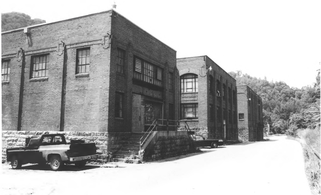
FORDSON COAL CO. BLDGS. RKE CO. KY ①
