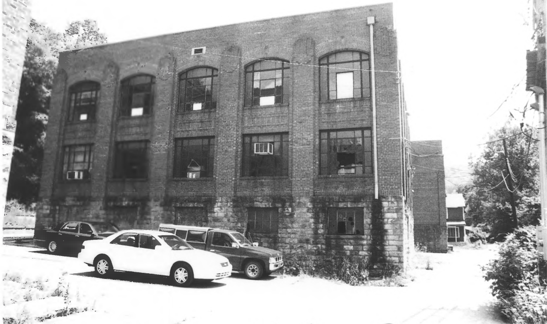
FORDSON COAL CO BLDG, PIKE CO, PA
