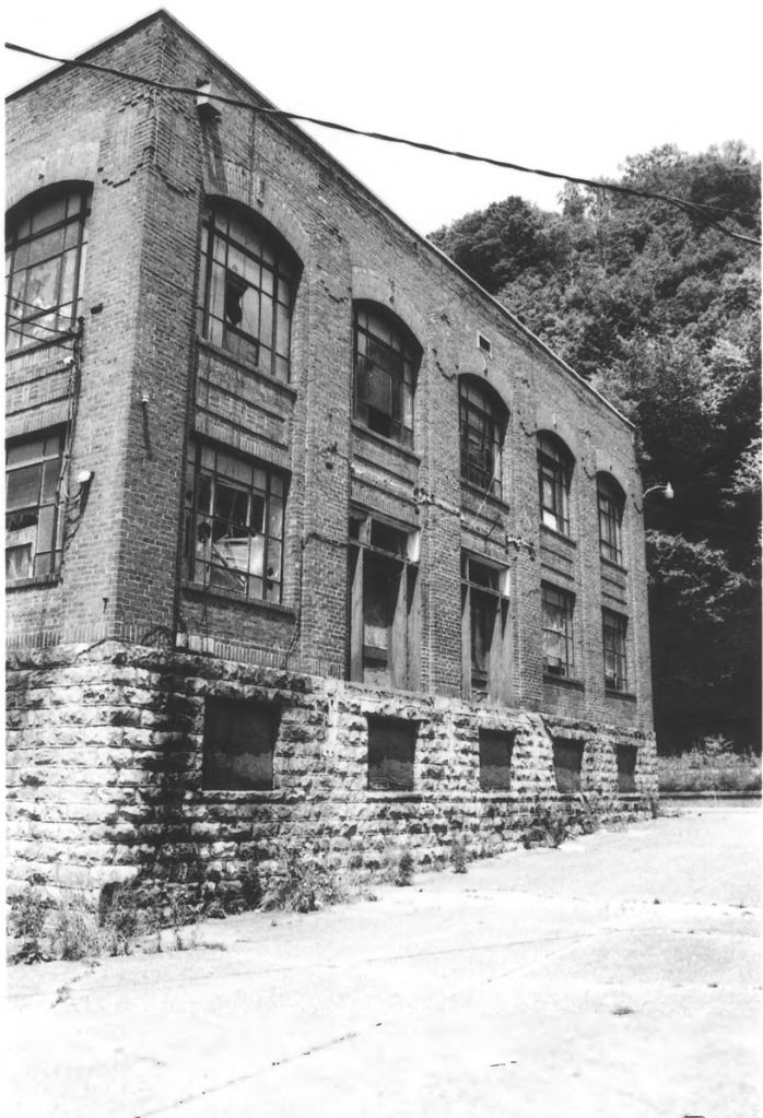
FORDSON COAL CO BLDGS PIKE CO, PA (11)
