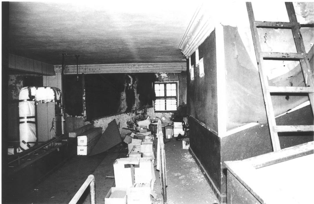
FORDSON COAL Co. BLDG, PIKE Co, PA
