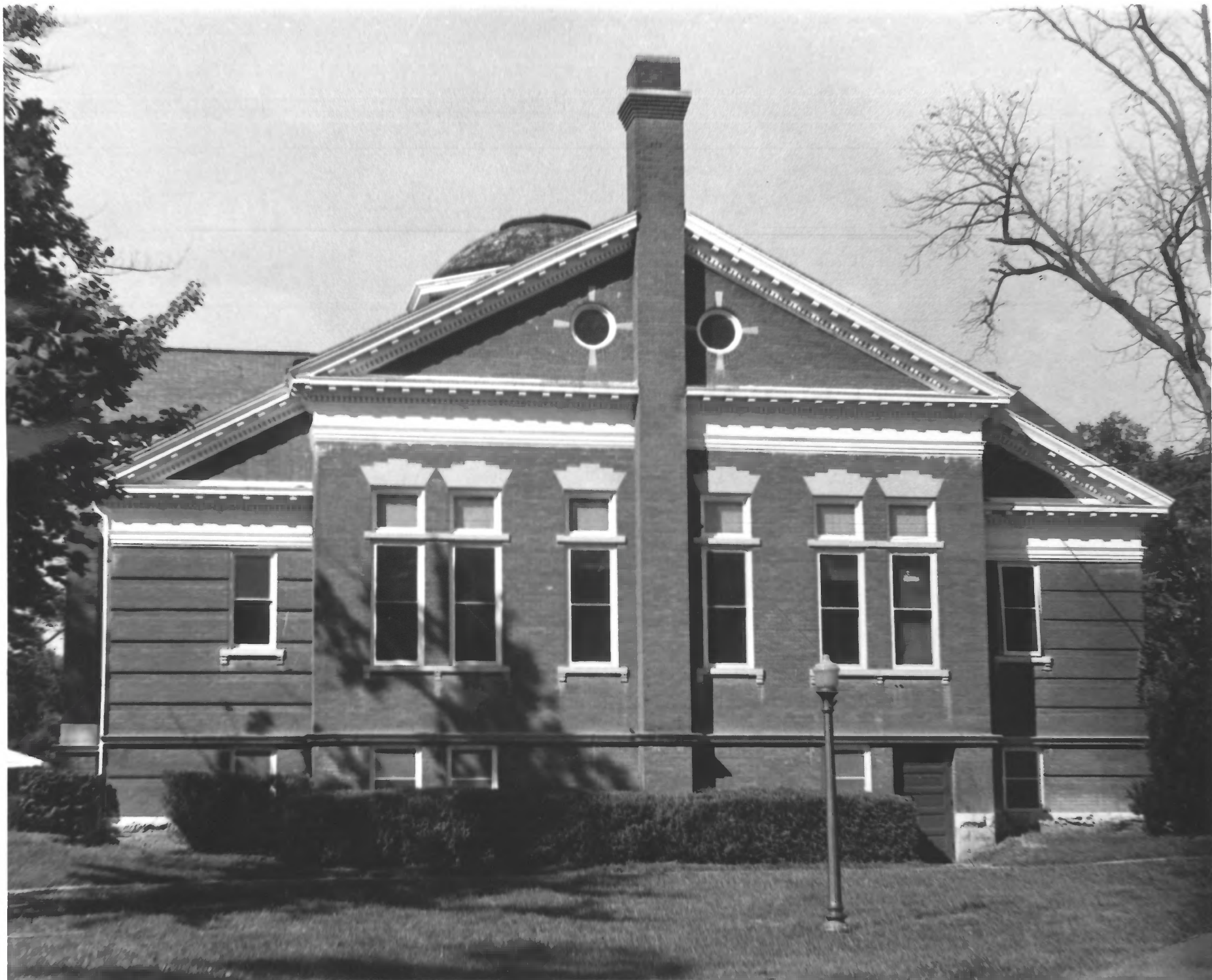
East side of building, rear
