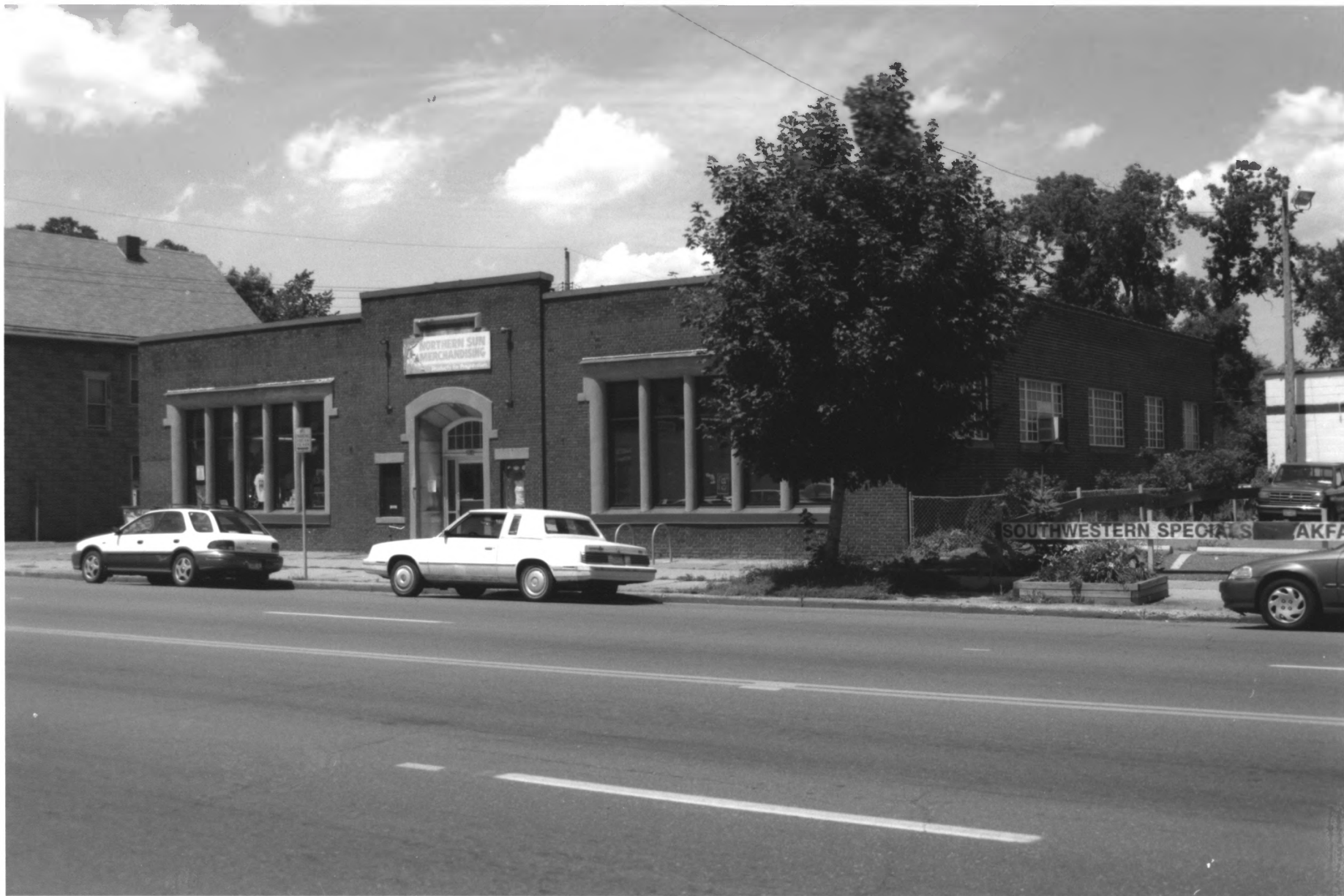
East Lake Branch Library 2916 E. Lake St., Minneapolis Hennepin County, MN 013407-4
