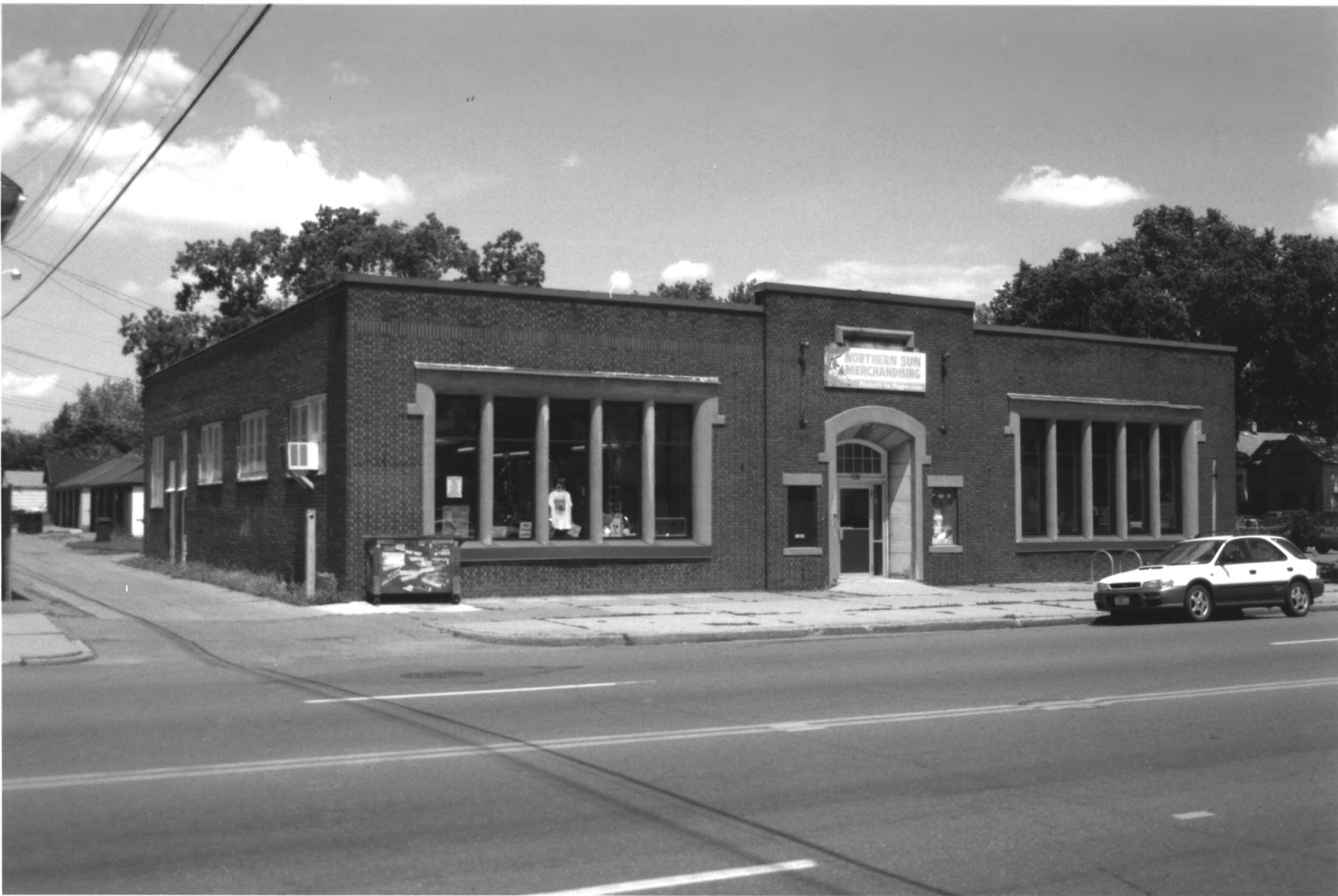
East Lake Branch Library 2916 E. Lake St., Minneapolis Hennepin County, MN 013407-3
