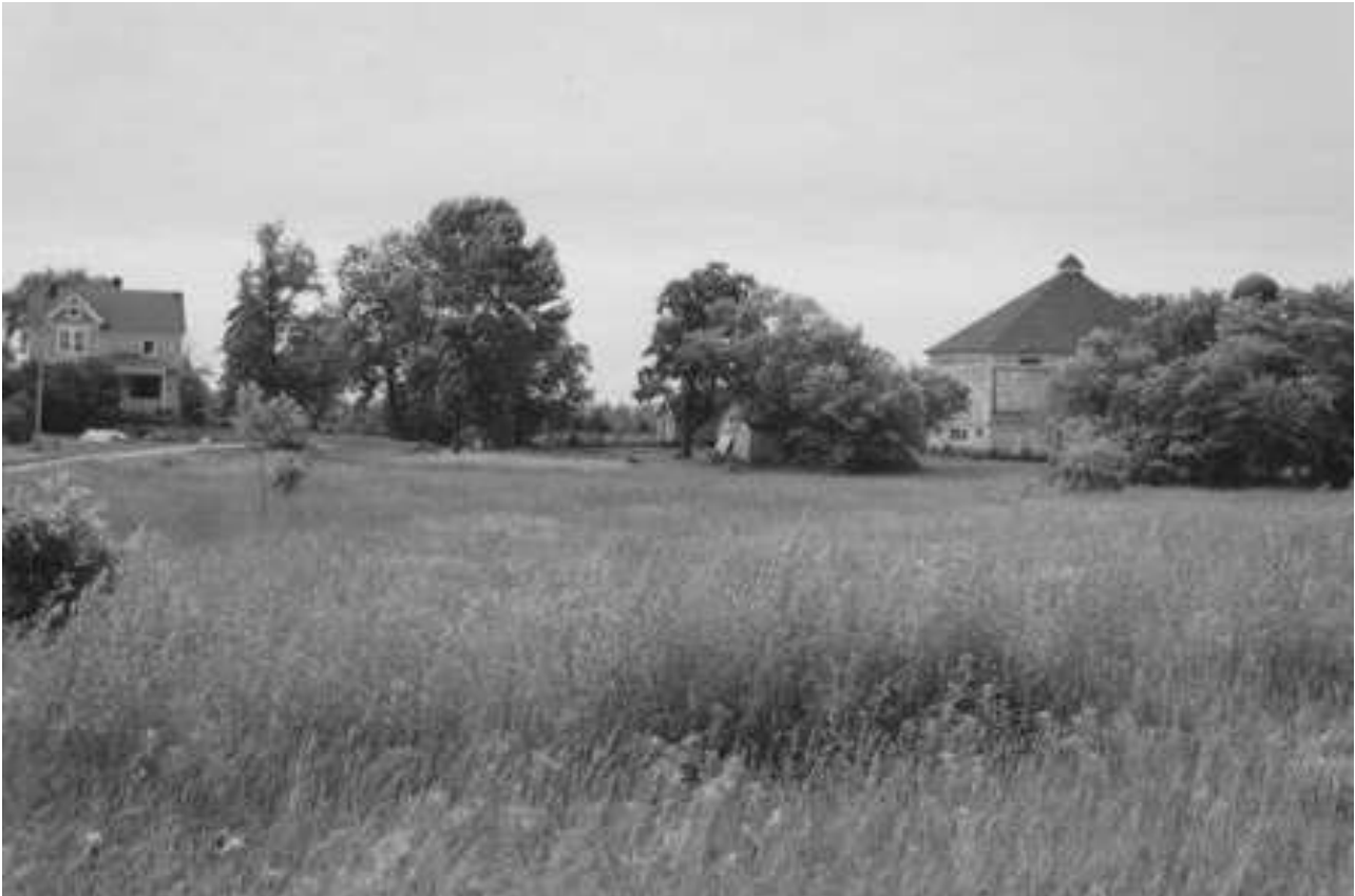
Photograph of the Frank Vocke Octagonal Barn and site from the north circa 1975. Image courtesy of the Wisconsin Historical Society.
