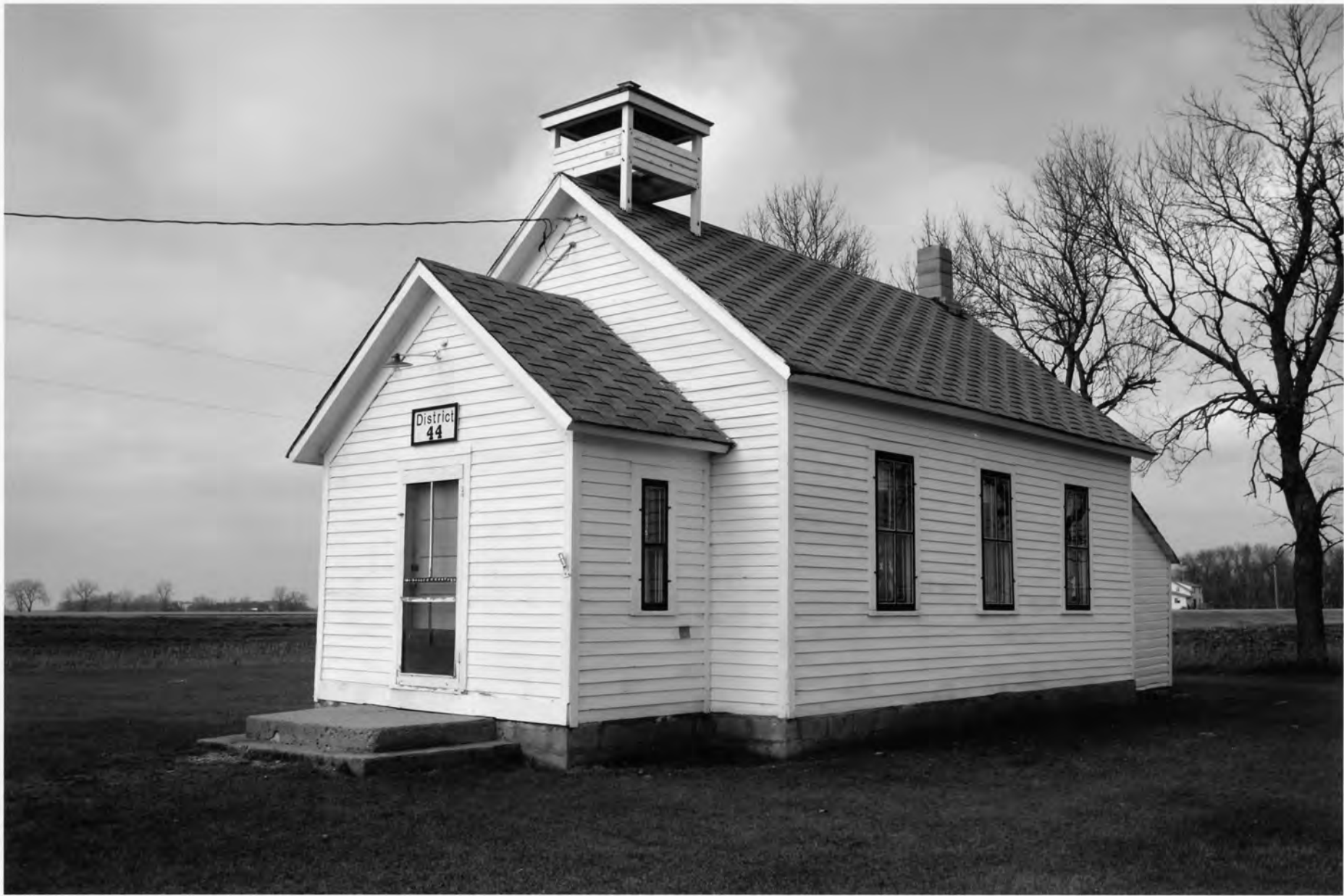
MN - Traverse County - School District No. 44 - 0003
