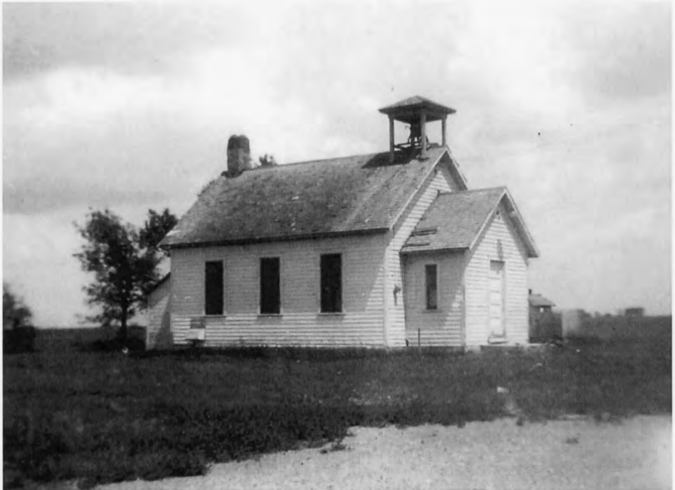
Figure 2: District No. 44 School, ca. 1940s. Photograph in the historical collection of Dawayne Novak, a former student at District No. 44 School.
