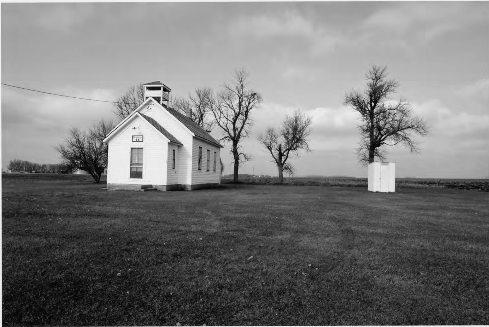
MN - Traverse County - School District No. 44 - 0001
