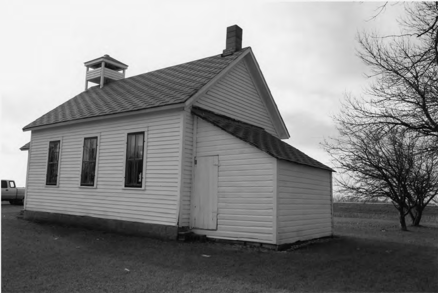
MN - Traverse County - School District No. 44 - 0004
