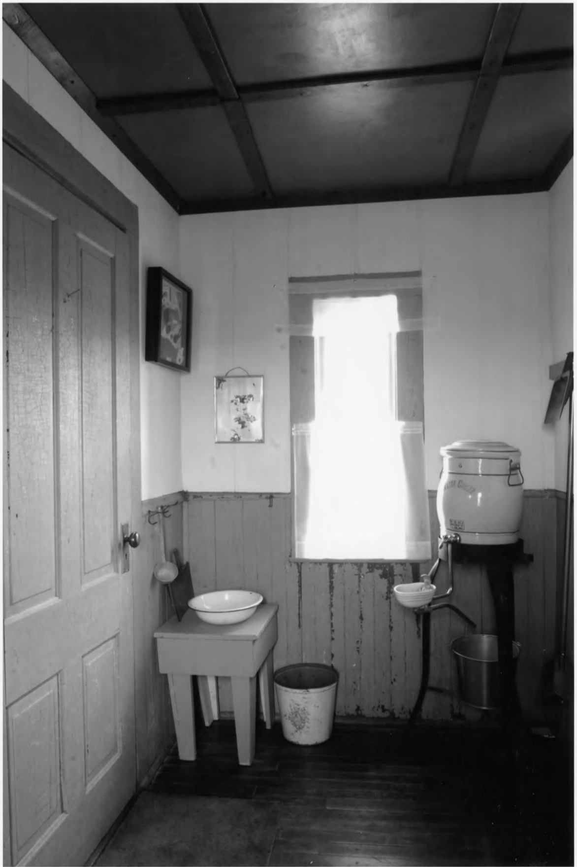
MN - Traverse County - School District No. 44 - 0007
