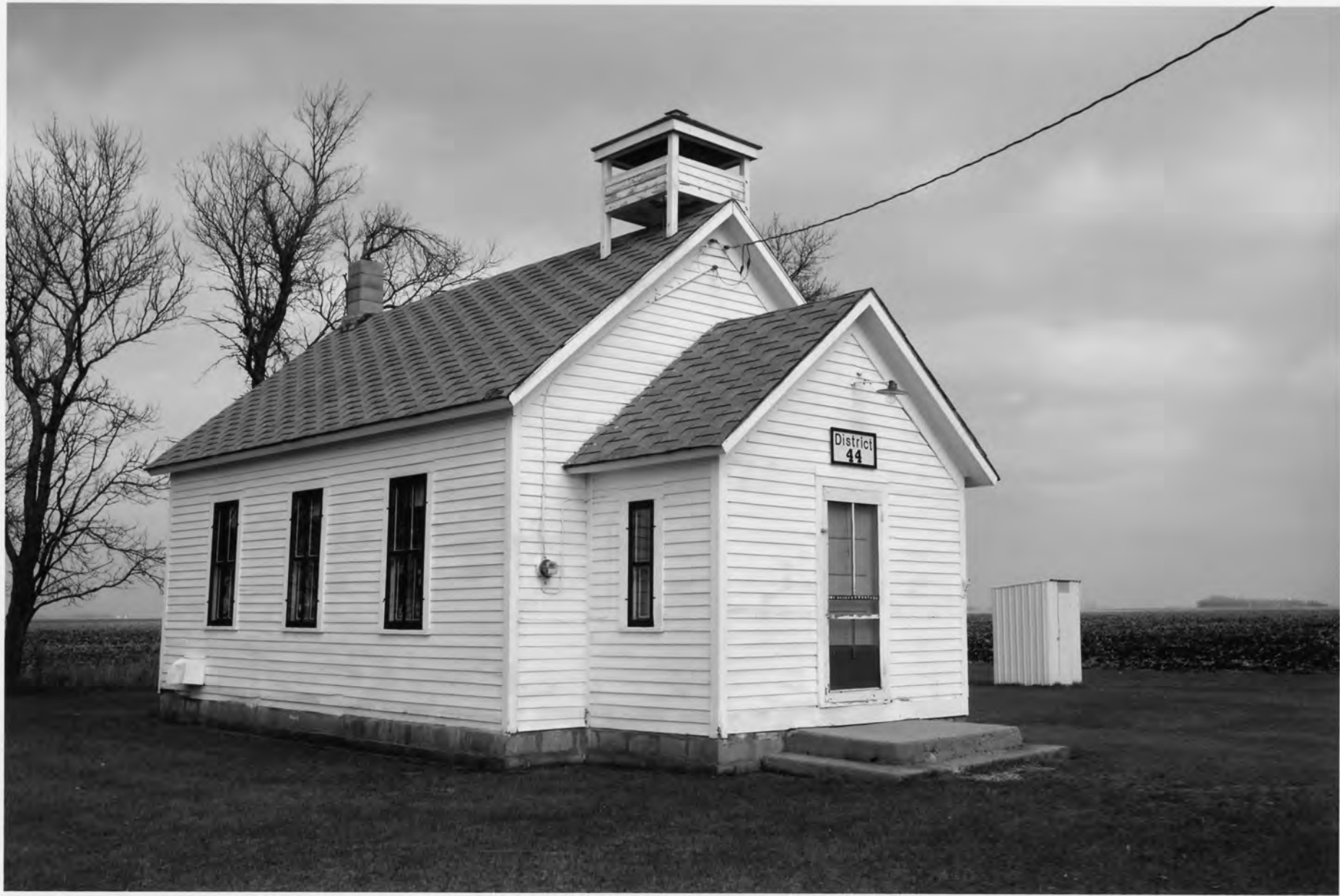
MN - Traverse County - School District No. 44 - 0002
